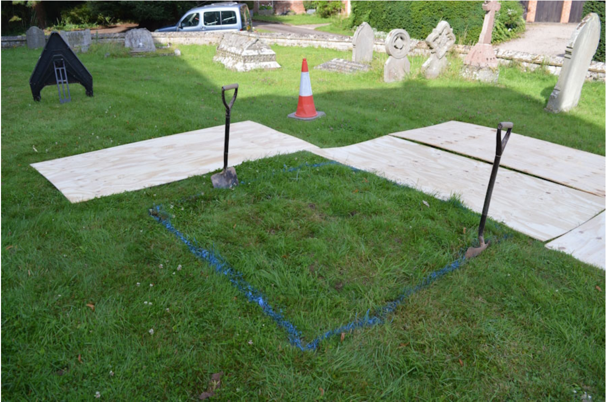
Plate 3. Area of the soakaway prior to excavation, view north-west
