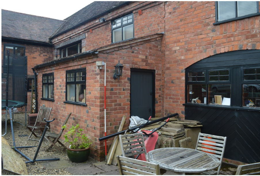
Plate 11. Lean-to to rear of Building 1
