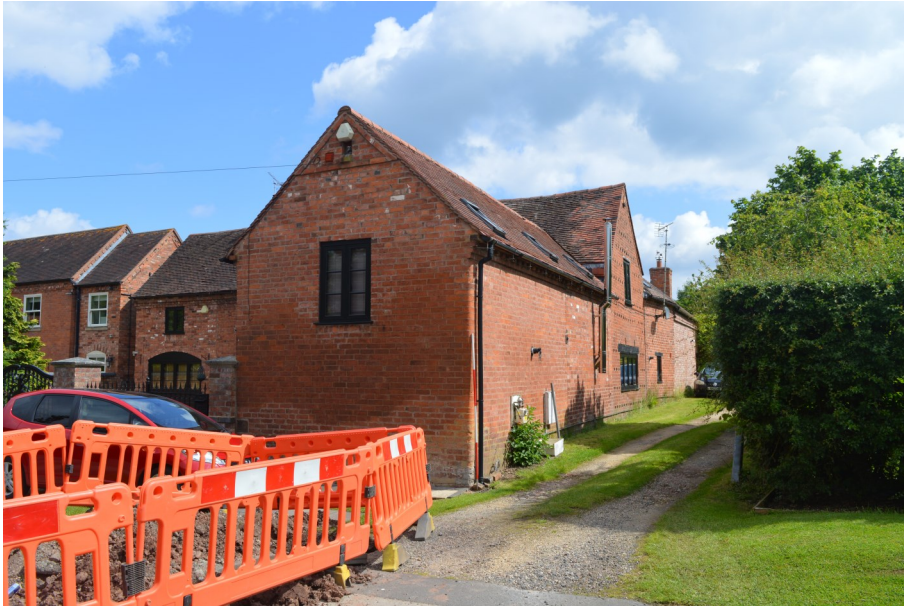
Plate 19. Oblique view of south-west gable, Building 4
