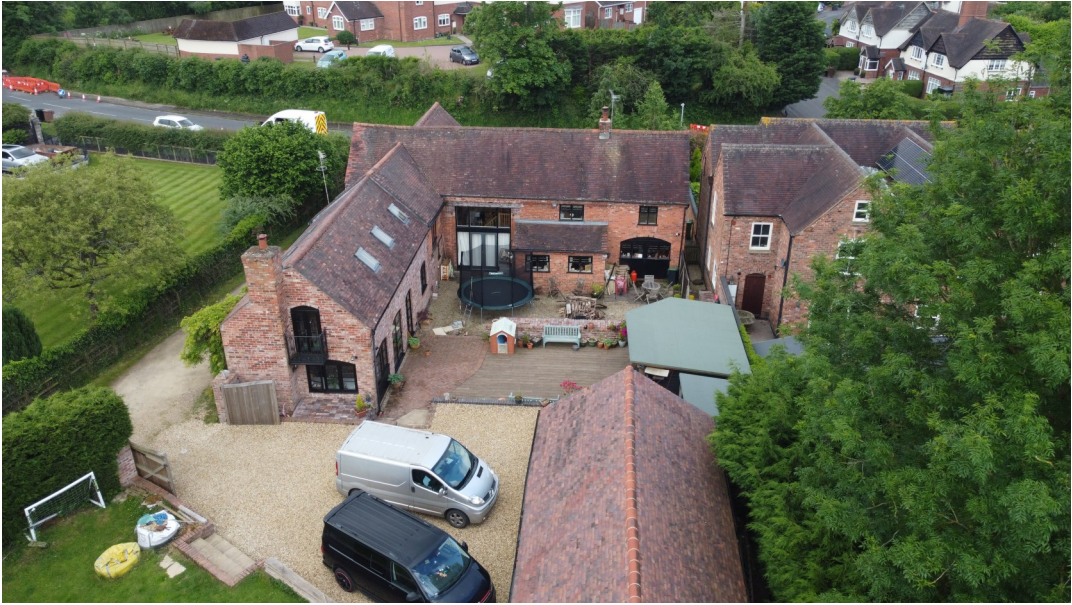
Plate 3. Low level aerial view south-west of the former farmstead
