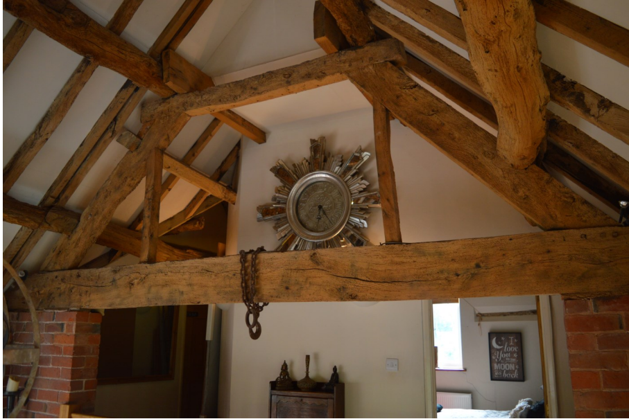
Plate 21. Roof truss, view north-west
