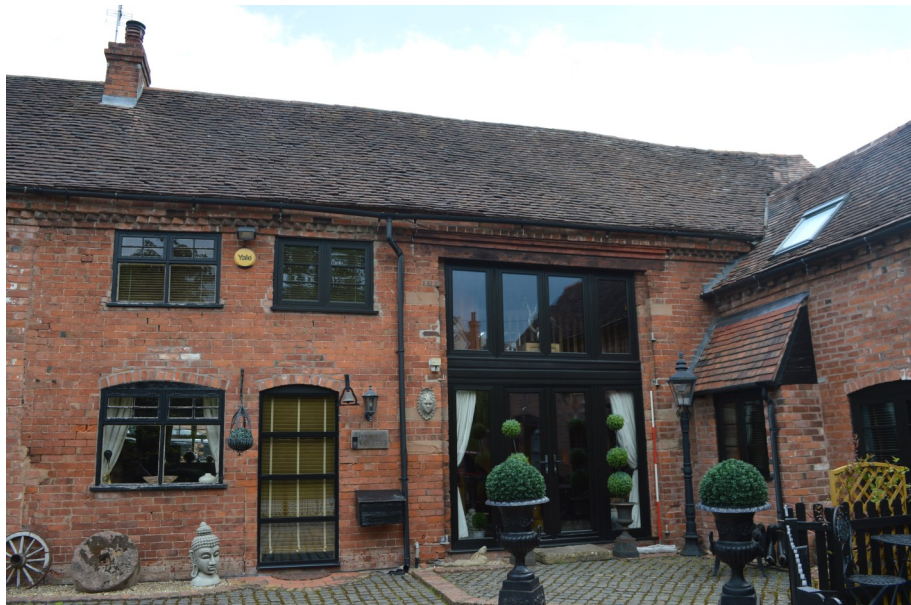
Plate 4. View north-east towards threshing doorway in Building 1
