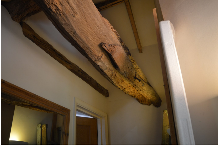
Plate 25. Exposed timbers in landing
