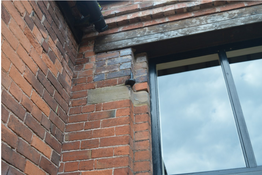
Plate 7. Detail of stone work in doorjamb in rear of Building 1
