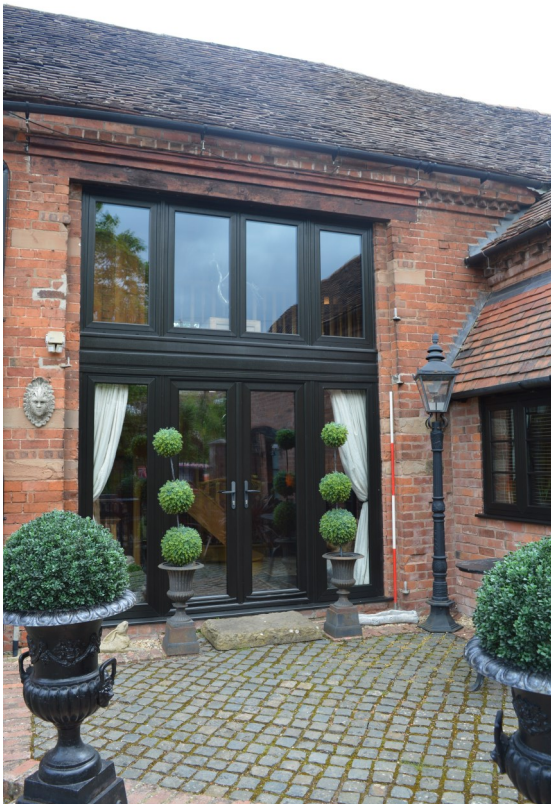
Plate 6. Threshing doors on the front elevation in Building 1
