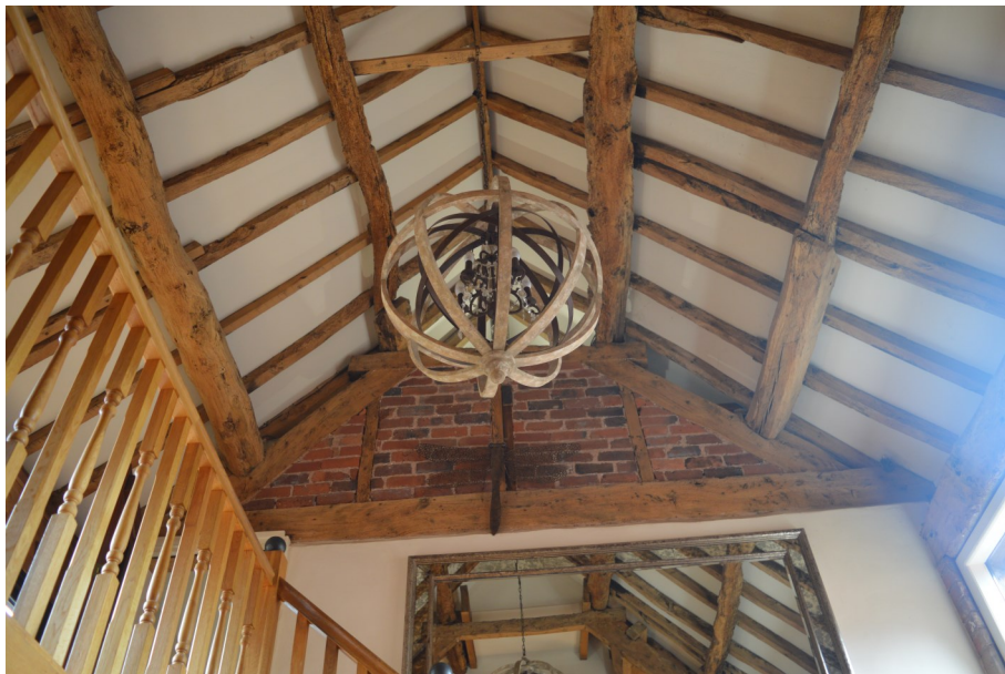
Plate 22. Roof truss, infilled with brick, view south-east
