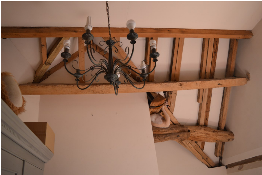
Plate 24. View north-east in bedroom, first floor, Building 1
