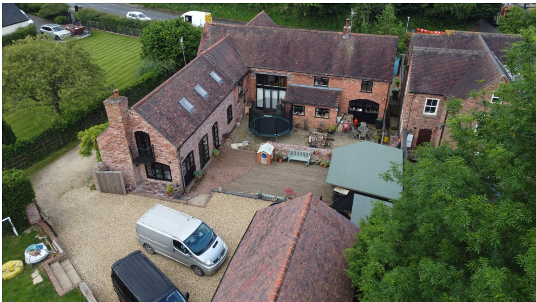
Plate 2. Low level aerial view south of the former farmstead
