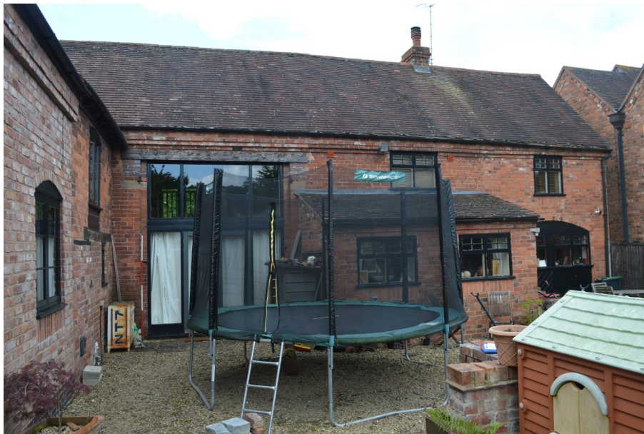
Plate 10. Rear elevation of Buildings 1 and 2
