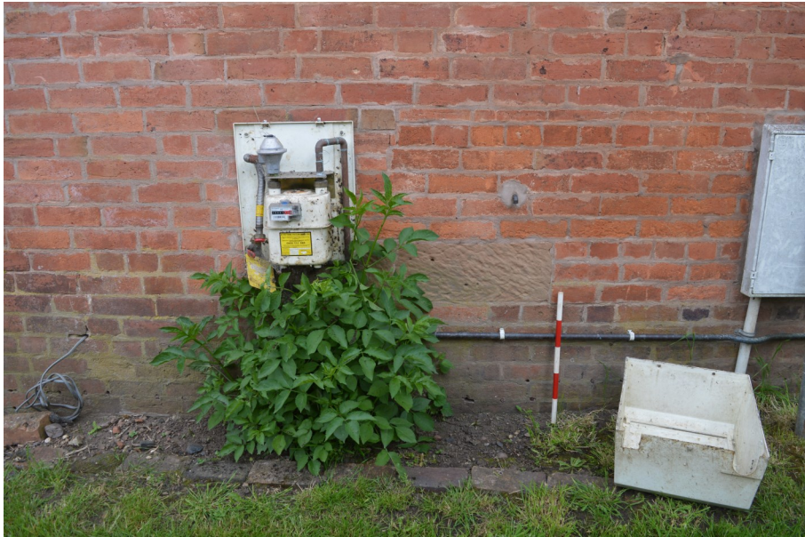
Plate 18. Reused ashlar blocks in Building 4, view north-west
