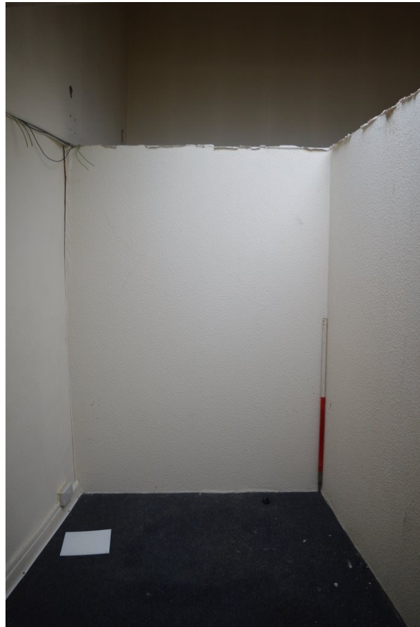
Plate 21. Stud walls define small area within Room 8, view west, scale 1m
