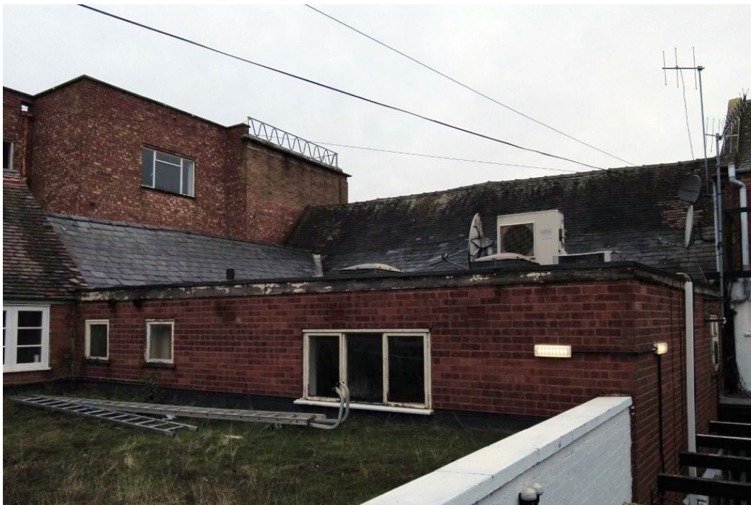
Plate 2. Rear view of building, view south-west. Ridge line of Phase 1 section of building to rear of air conditioning unit, Phase 2 extension with slate lower and to left, Phase 3 flat roofed extension in foreground.
