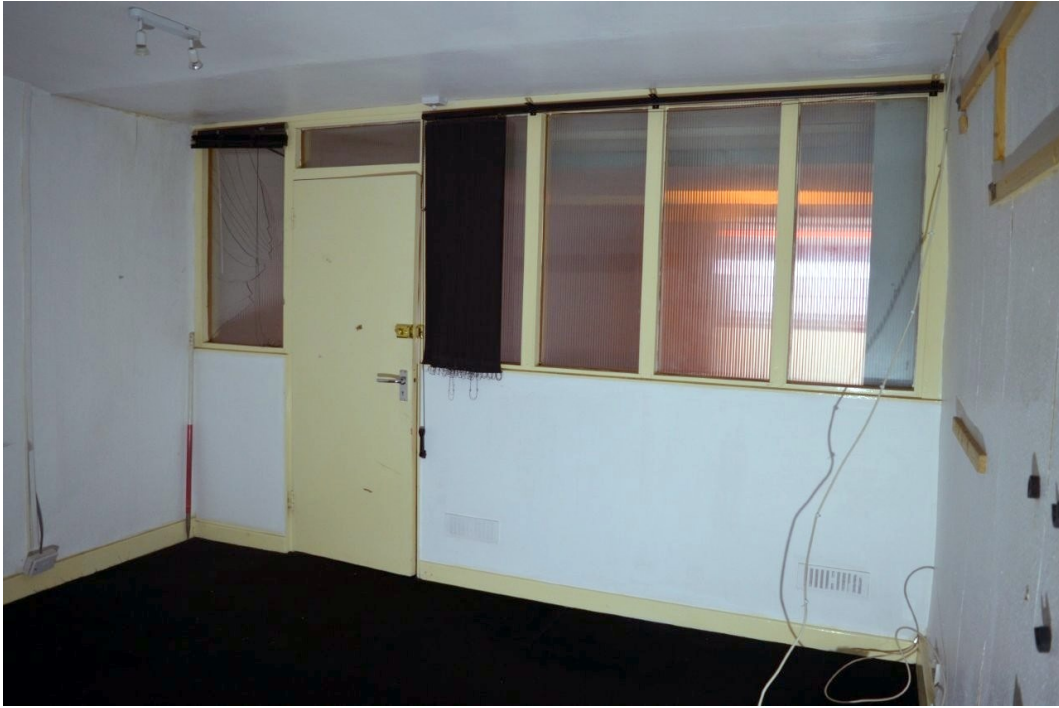
Plate 11. Room 2, view north-west, scale 1m
