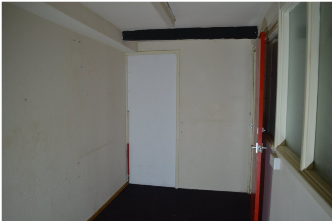
Plate 22. Room 9, view north, scale 1m
