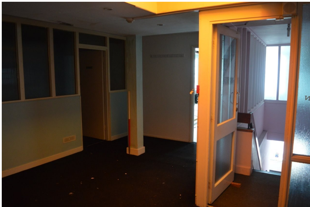
Plate 14. Room 3, view south-west, scale 1m, propped against boxed-in timber
