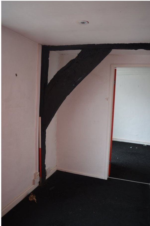
Plate 25. Knee brace exposed in Room 11, view NNW, scale 1m
