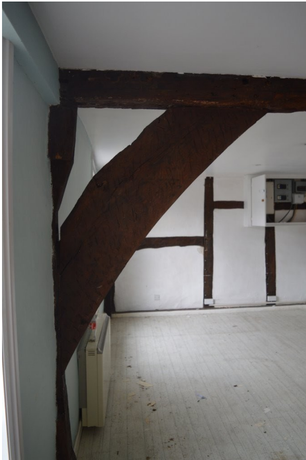
Plate 6. Knee brace extending from post in western wall, Room 1, view north.
