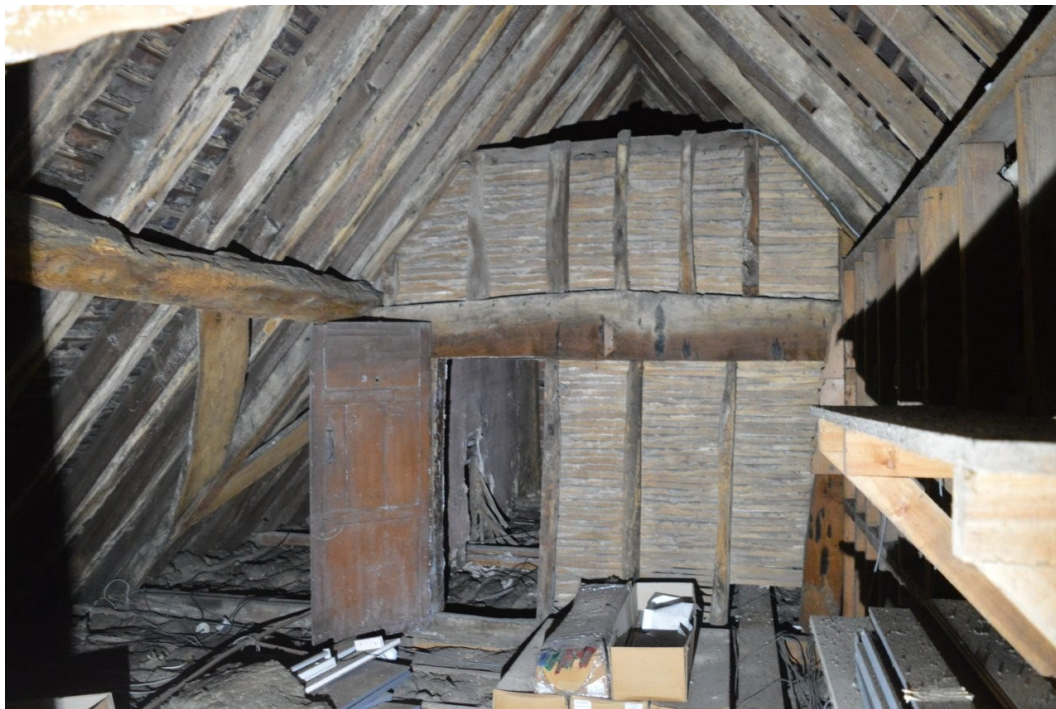
Plate 28. View north to northernmost bay in Phase 1 building
