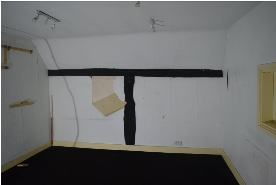
Plate 12. Room 2, view SSE, scale 1m
