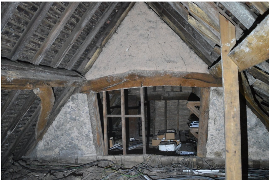
Plate 26. View north to central truss in Phase 1 building
