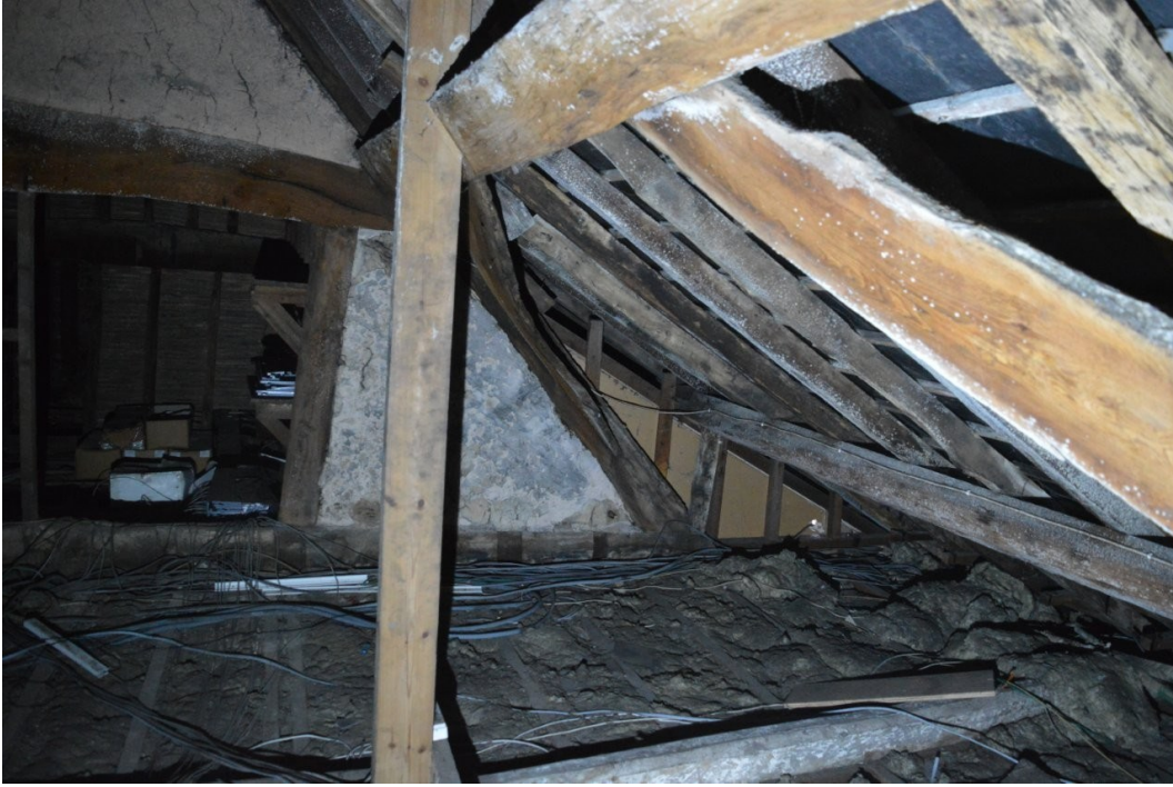
Plate 29. View north in attic space of Phase 1 building showing how the southern pitch of the roof has been raised
