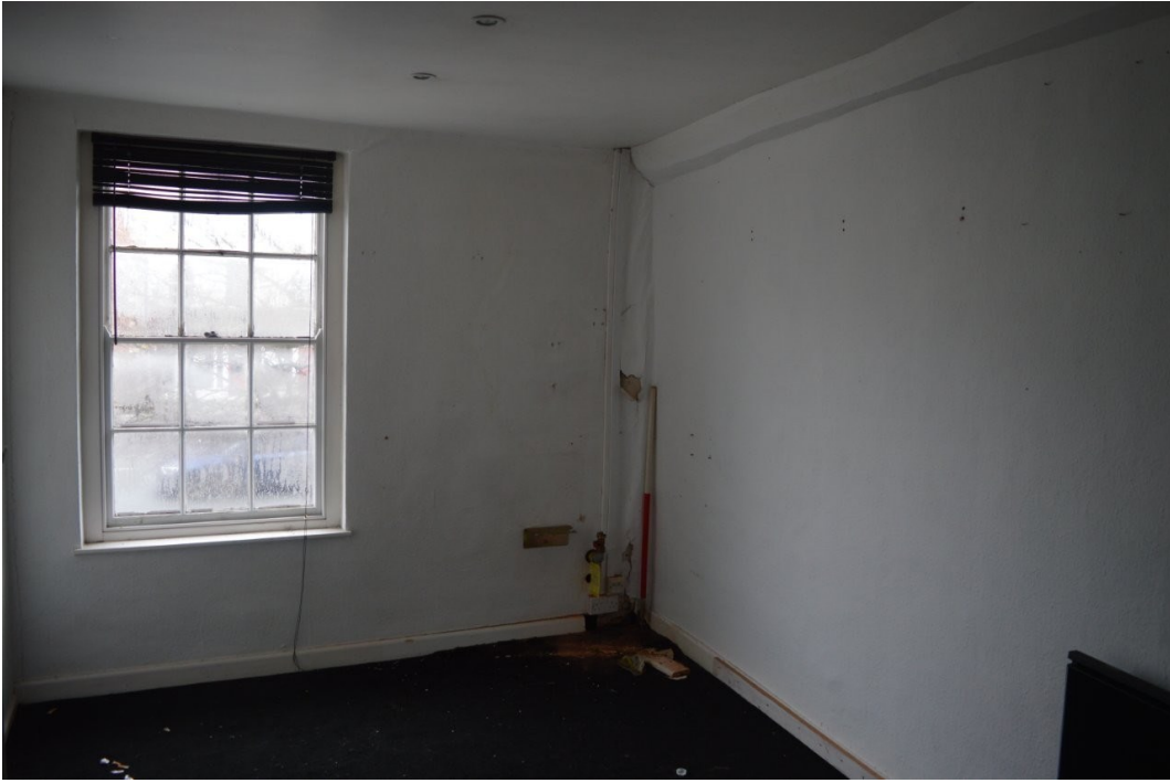
Plate 23. Room 10, view WNW, scale 1m
