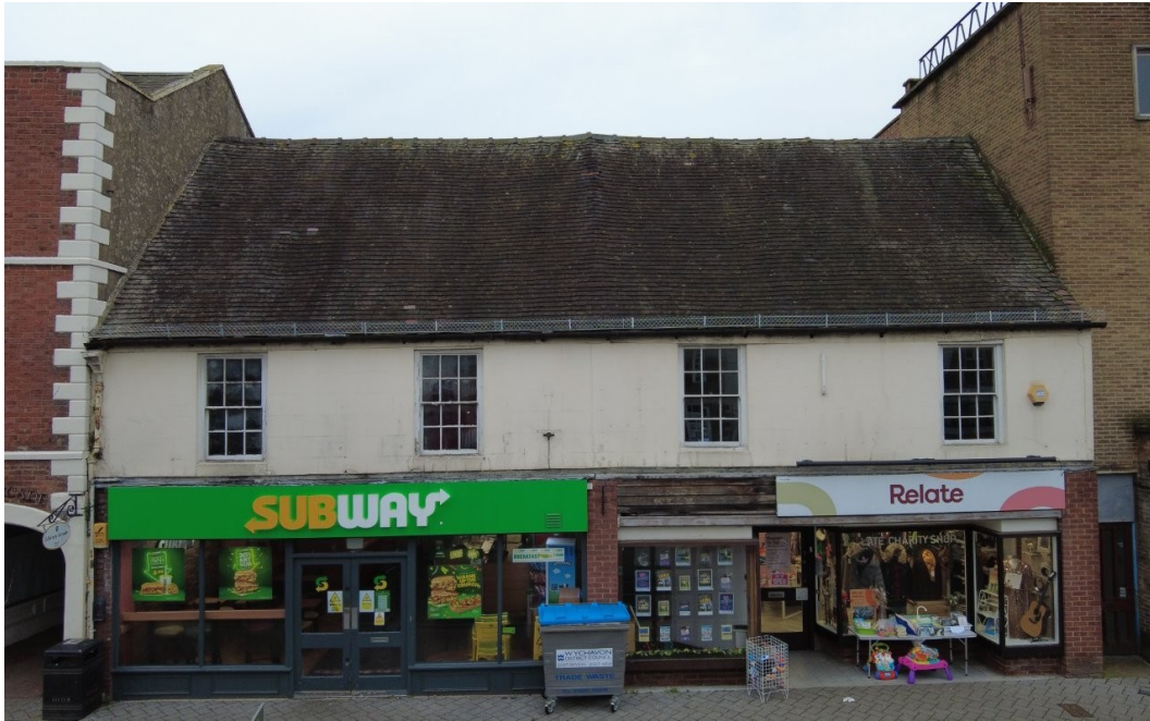
Plate 1. Western elevation of building, view east
