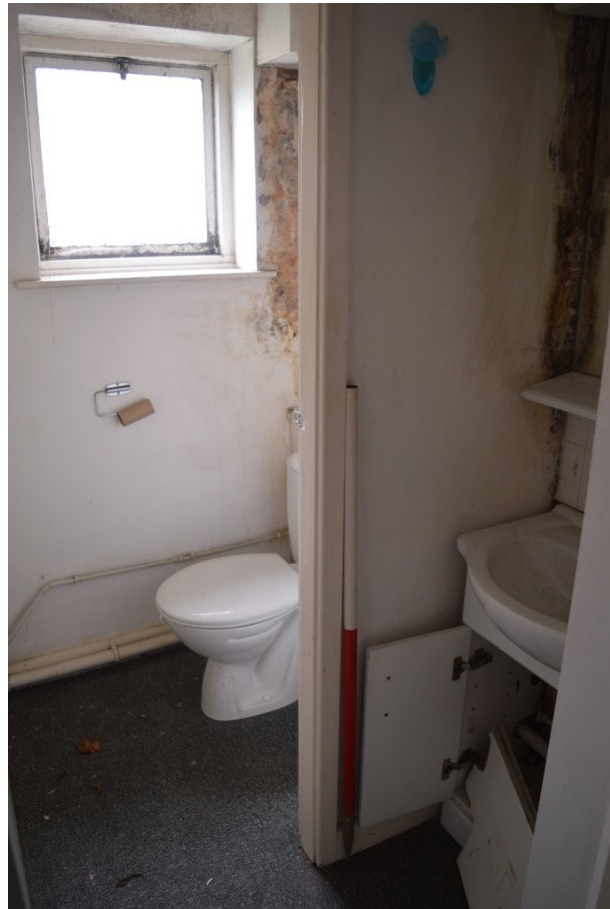
Plate 18. Room 5, female toilets, view south-east
