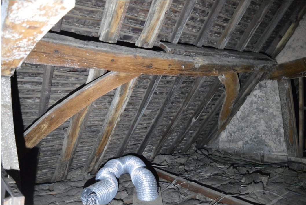
Plate 27. Curved windbraces in western pitch of roof above Phase 1 building, view north-west
