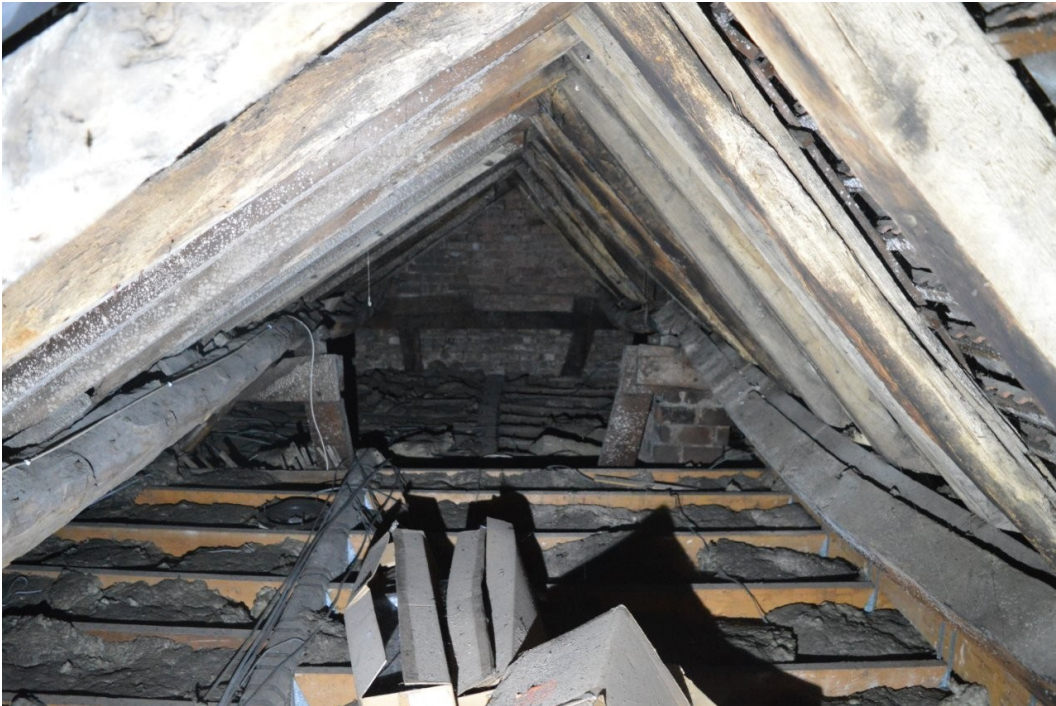
Plate 30. View east through attic space above Phase 2 extension to the rear. Note truncated collar beam.
