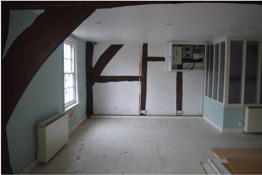
Plate 9. Room 1, view north to central division of Phase 1 building, scale 2m
