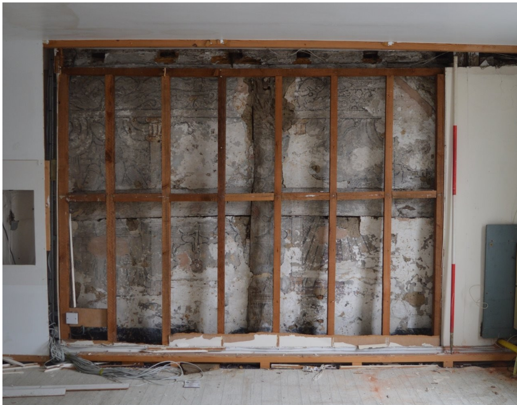
Plate 10. Exposed area of wall painting, Room 1, view south, scale 2m (see also Figures 9 and 10)
