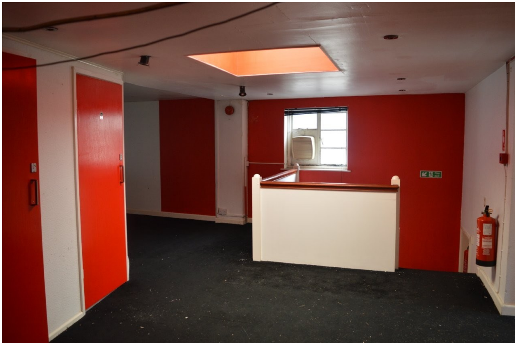
Plate 20. Room 7, view north-west, scale 1m against boxed-in timber
