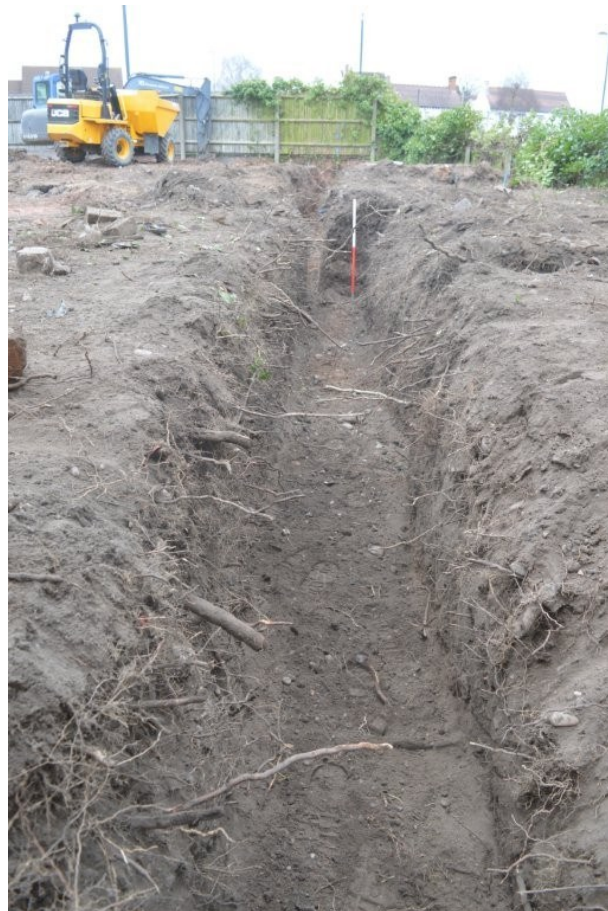
Plate 4. View north-east along arm of foundation trench, scale 1m
