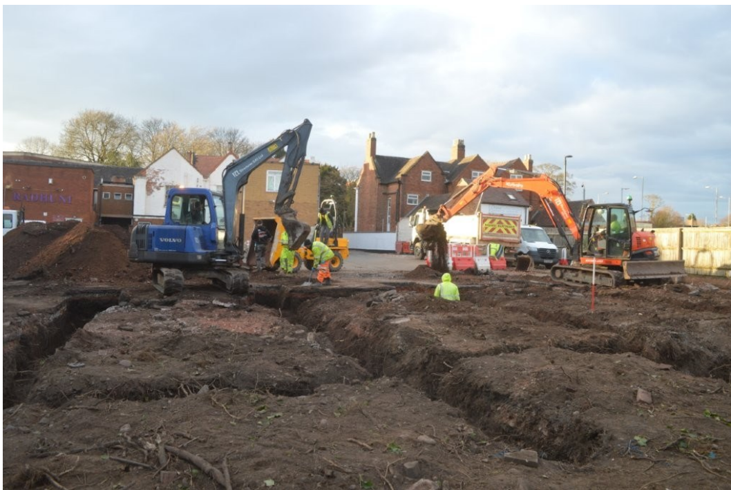
Plate 2. Excavation of foundations in progress, view NNW
