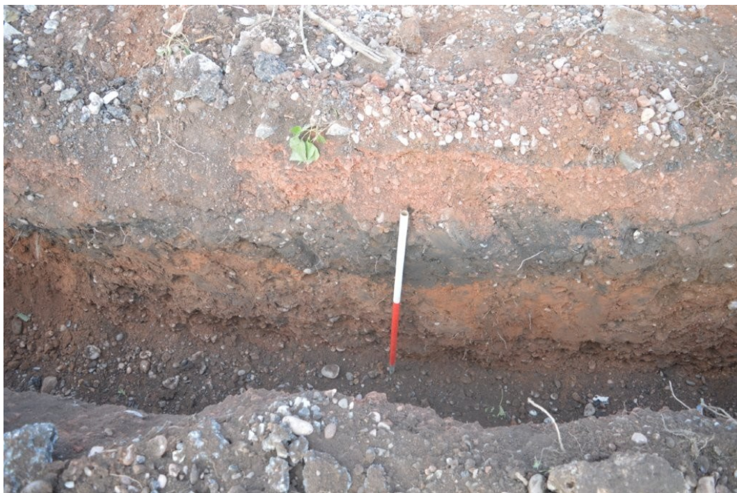
Plate 8. Section in central part of foundation trenches showing thicker layer of subsoil (1006), view north-east, scale 1m
