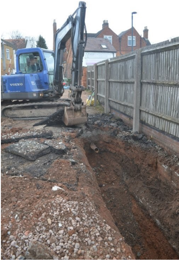
Plate 9. North-eastern arm of foundations under excavation, view north-west
