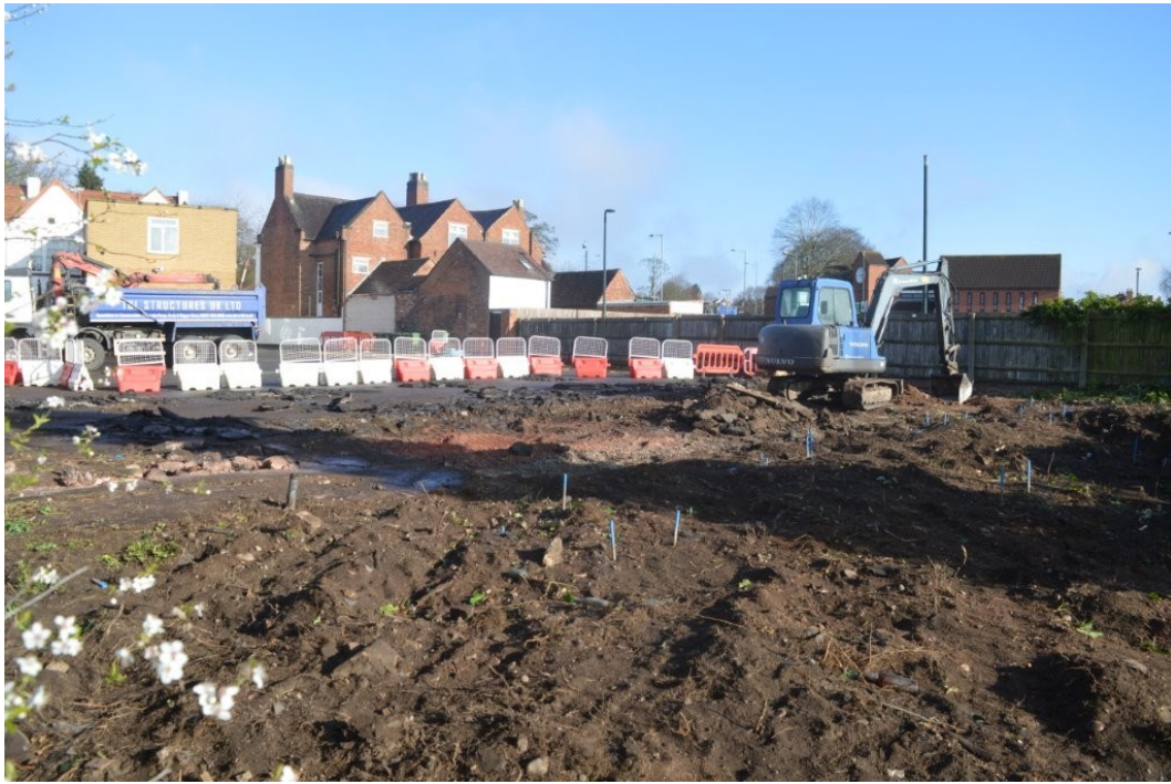
Plate 1. View north across site prior to excavations
