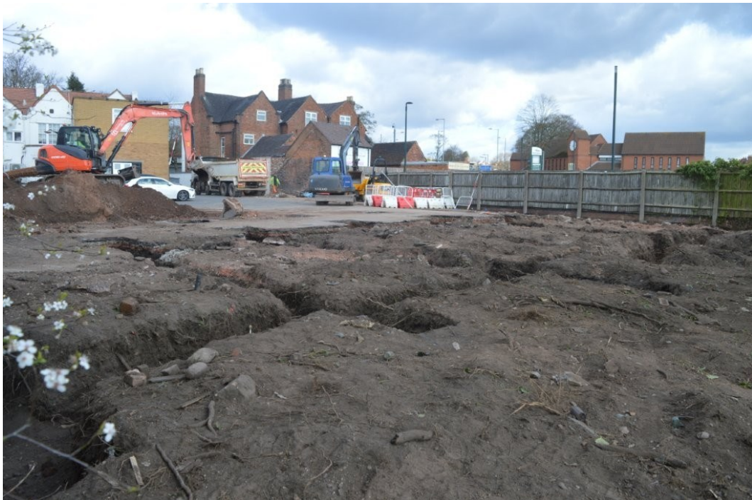
Plate 12. The site with foundation trenches completed, view north
