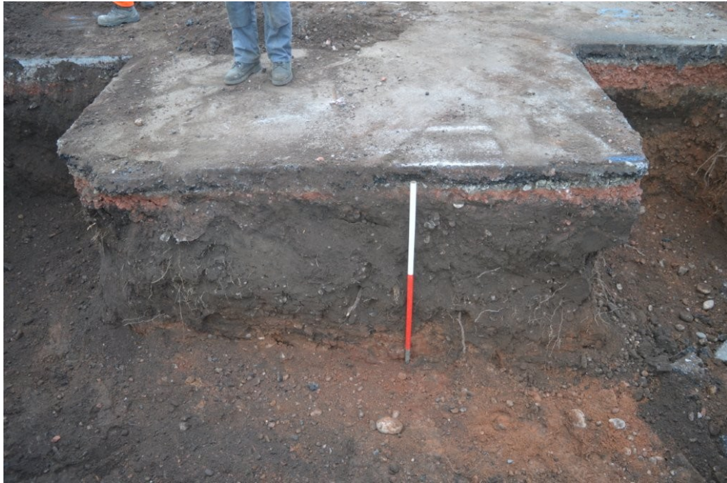
Plate 3. Section in north-western arm of foundation trenches, view north-west, scale 1m
