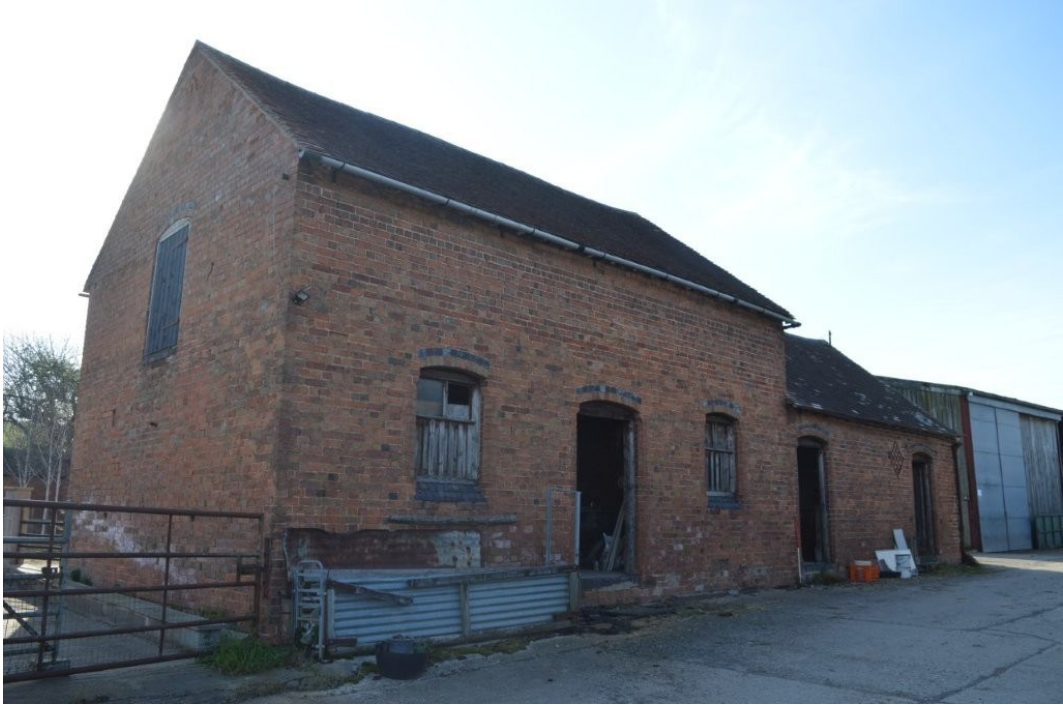
Plate 5. North and west elevations of Stables Barn, view south-east, scale 1m
