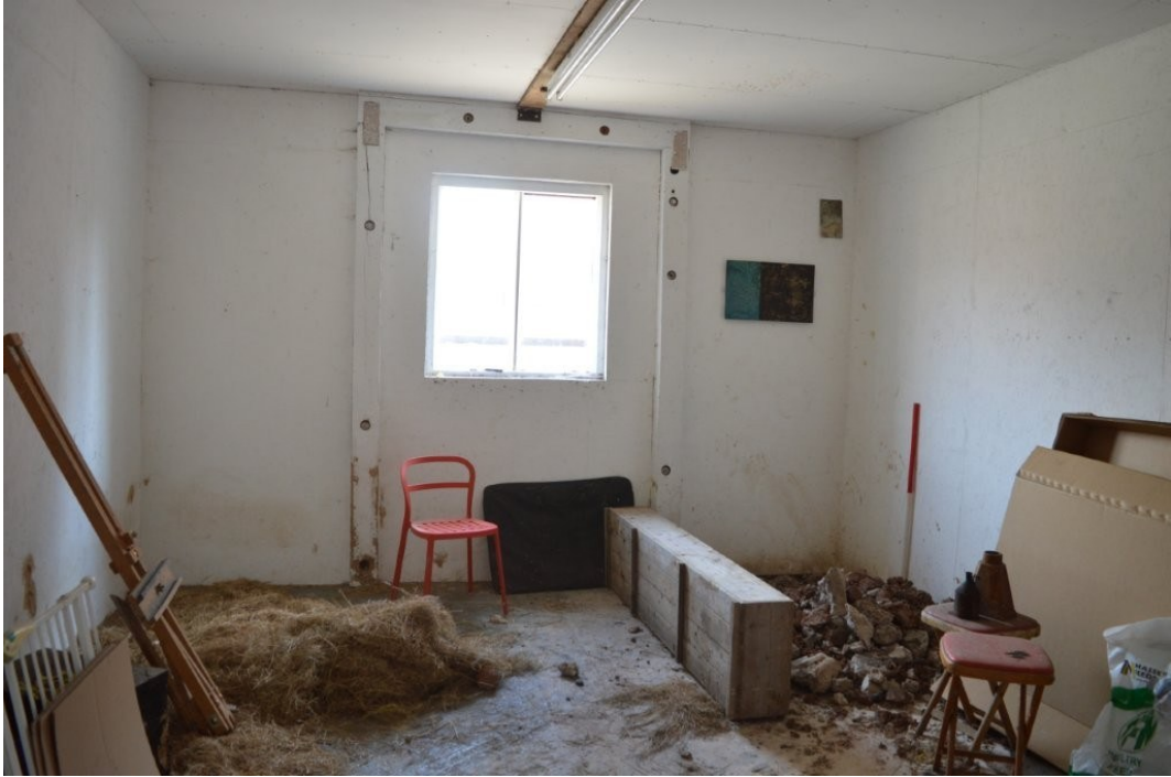
Plate 31. View north east in southern room of building, scale 1m
