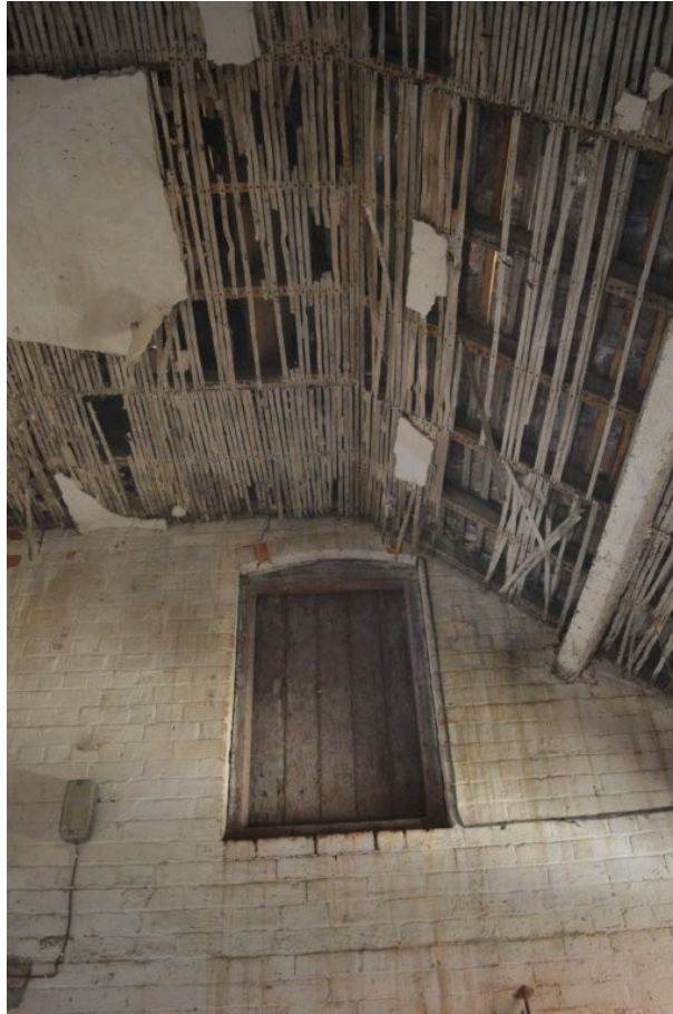
Plate 29. Remains of ceiling and hay door in north wall of central-east section
