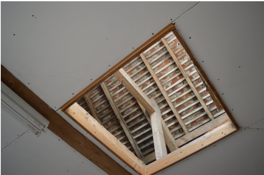
Plate 32. View into attic space above southern room
