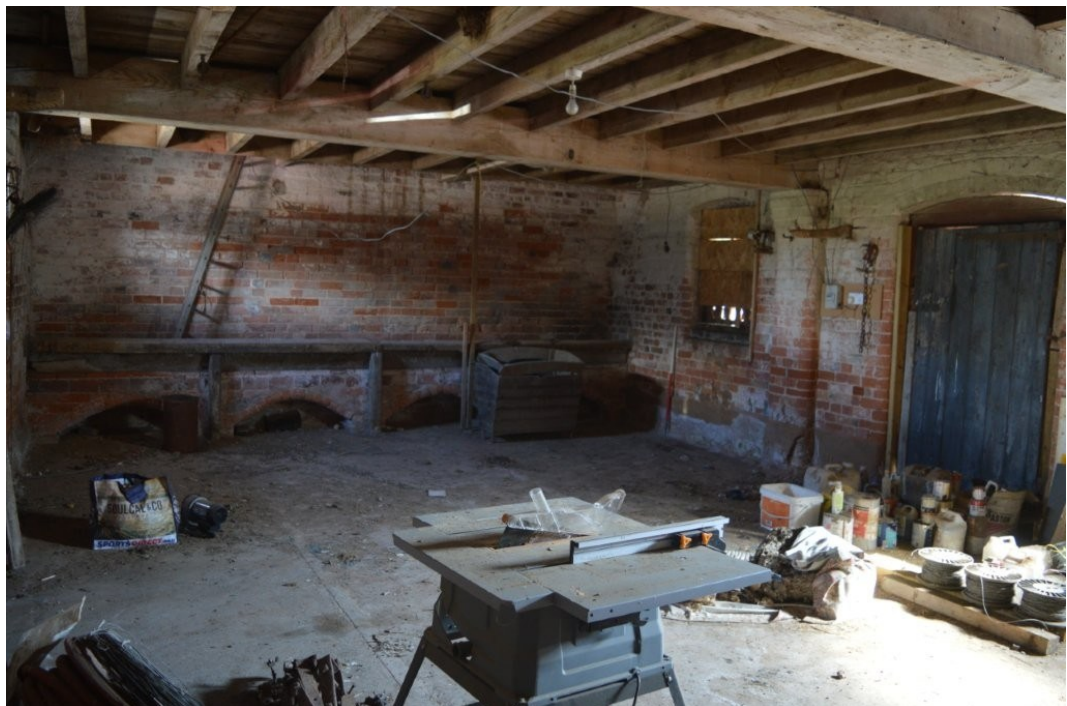
Plate 16. Stables on ground floor of two storey section, view north-east
