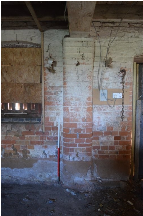
Plate 18. Brick pilaster supporting transverse beam in stables, view east, scale 1m
