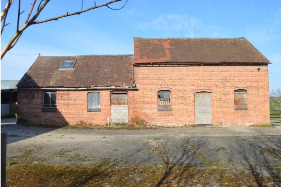
Plate 13. Eastern elevation of Stables Barn, view west, scale 1m
