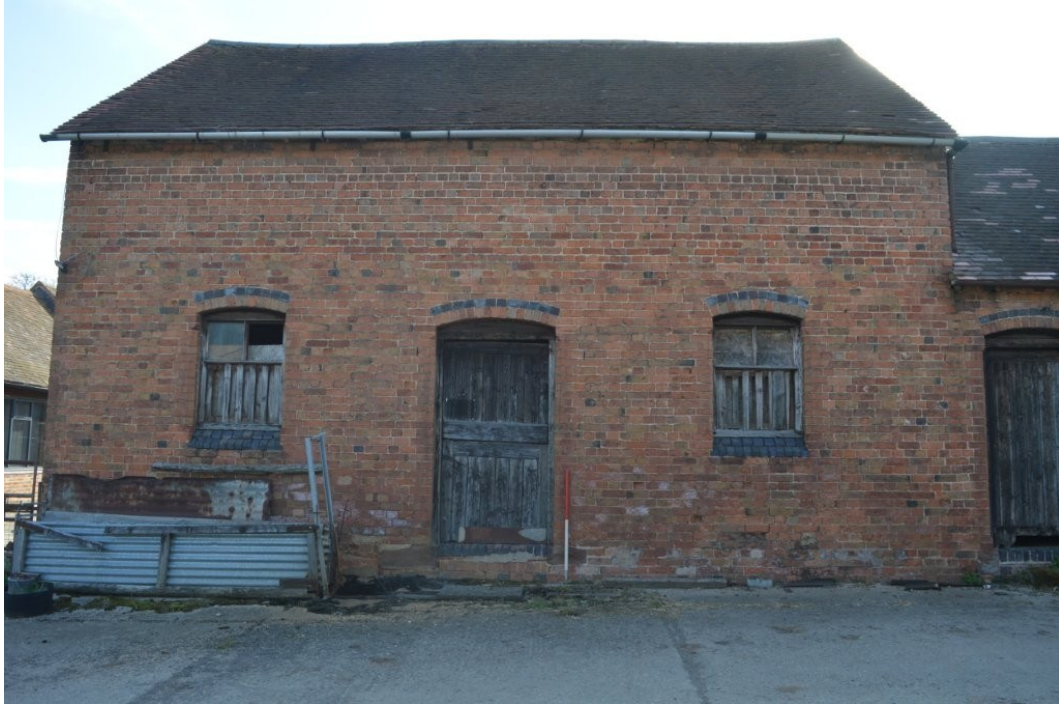
Plate 7. West facing elevation of northern section of Stables Barn, view east, scale 1m
