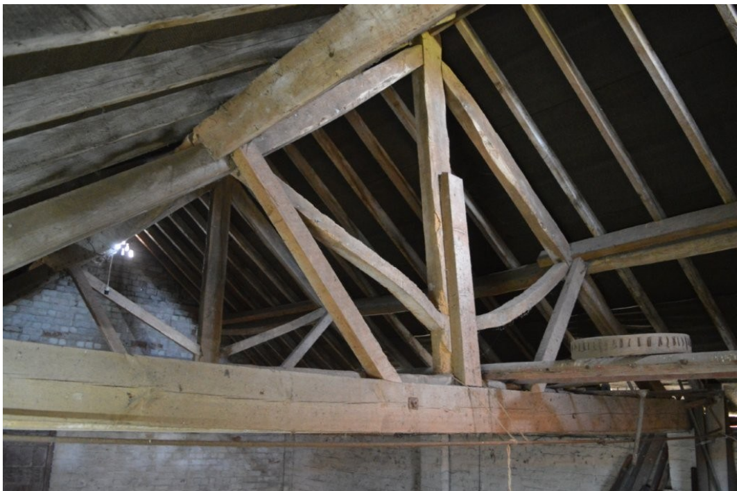
Plate 24. Roof trusses in hay loft, view south-west
