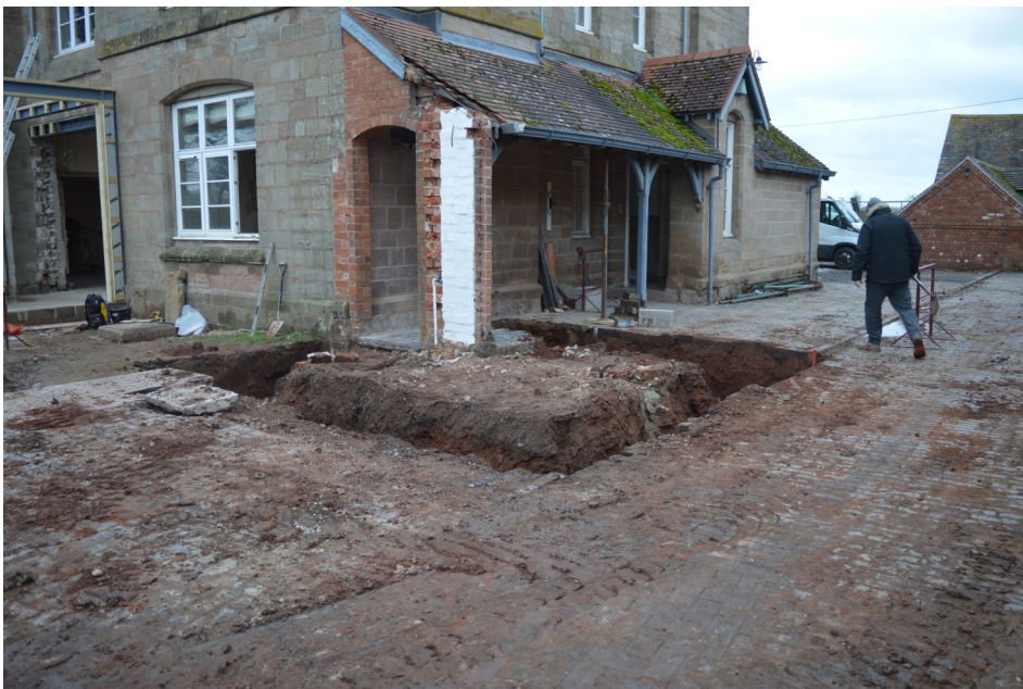
Plate 10. View NW of Trench 2
