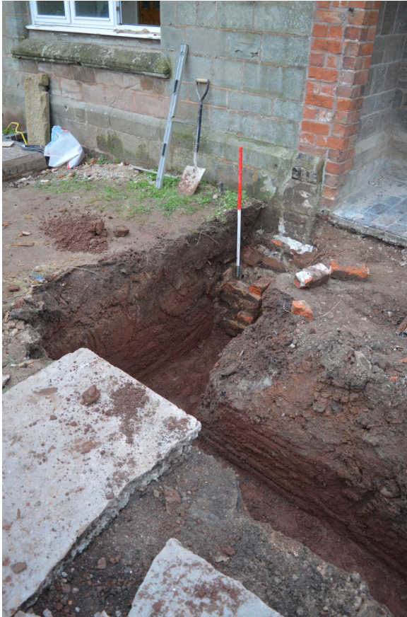
Plate 7. View NNW of part of house foundation (217), scale 1m
