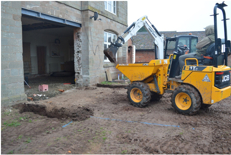
Plate 1. View north-east mid way through excavation of Trench 1
