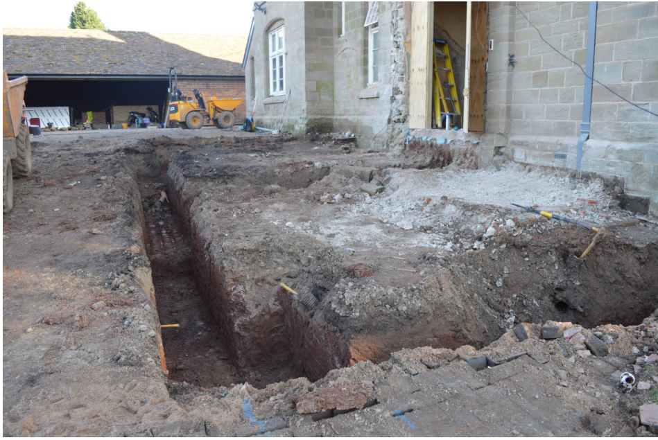
Plate 15. View SW of Trench 3
