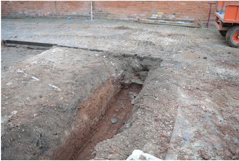
Plate 5. View ENE of southern arm of Trench 2
