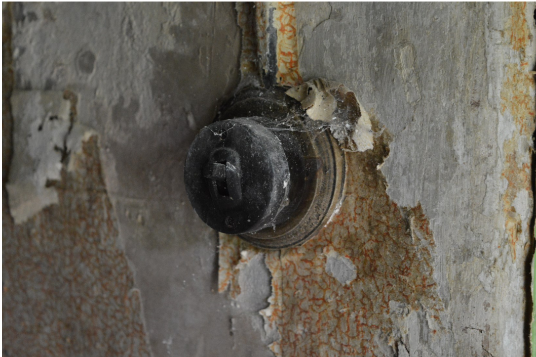
Plate 20. Plastic and Bakelite electrical fitting, Room A
