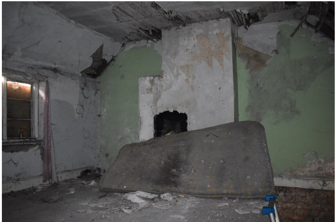
Plate 24. View west in Room C
