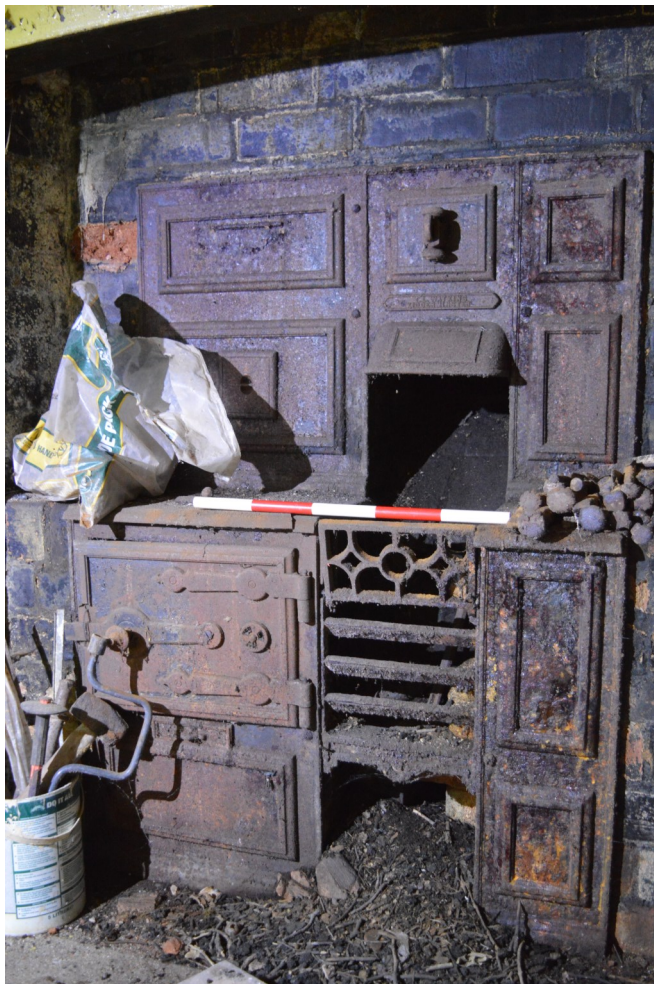
Plate 16. Cast iron range in north-west of Room A, Scale 0.50m
