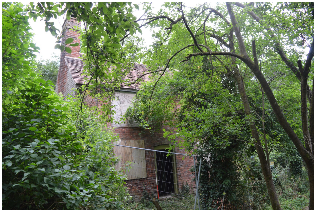
Plate 2. View north-east of Ford Cottage, scale 1m
