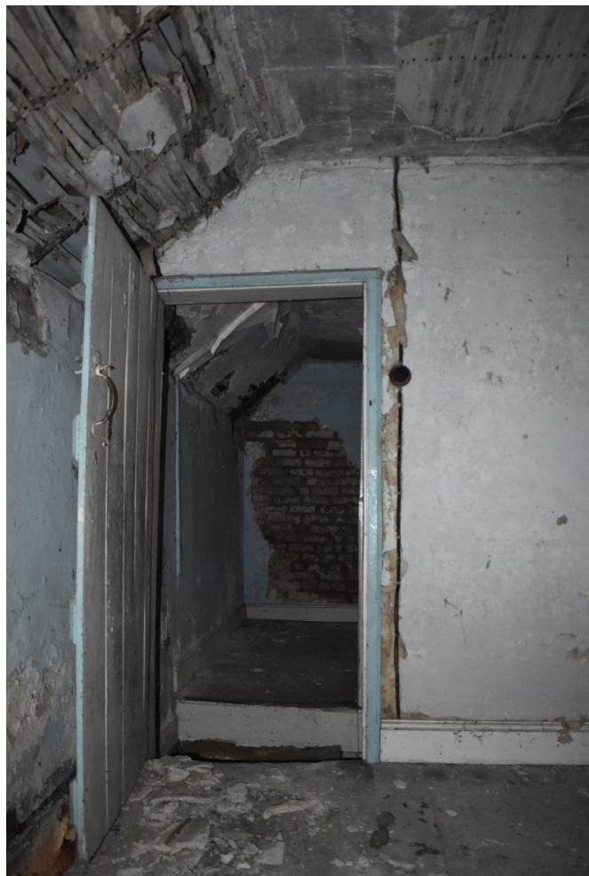
Plate 26. View east in Room C
