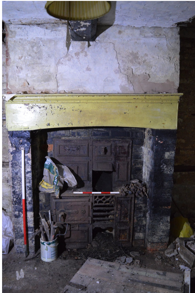
Plate 15. Cast iron range in north-west of Room A, Scales 1m and 0.50m
