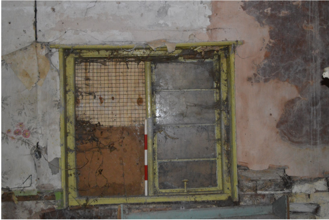
Plate 19. View south-west of Crittall style window, Room A, scale 0.50m
