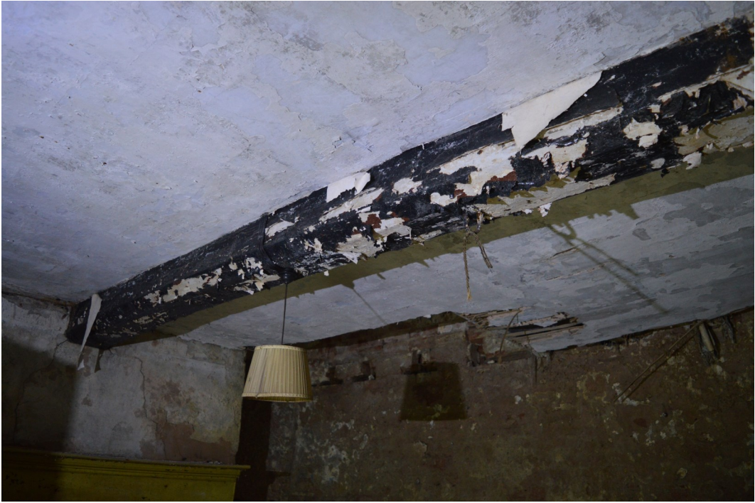
Plate 17. View north of chamfered beam in Room A
