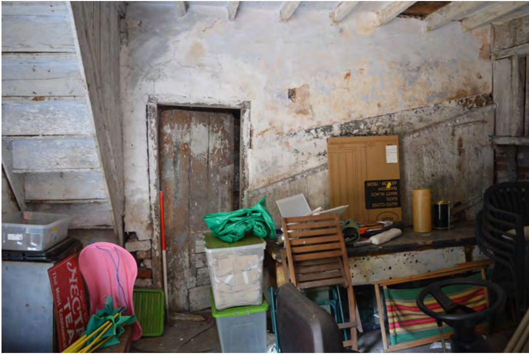
Plate 23. View west in Room 2
