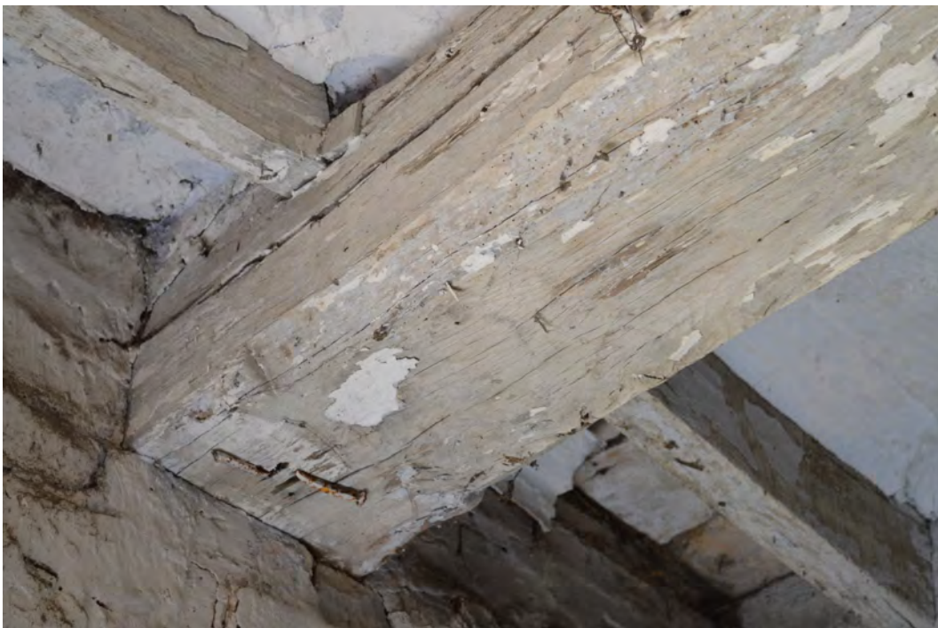
Plate 20. Beam with chamfer and stops in Room 2, view south-south-west
