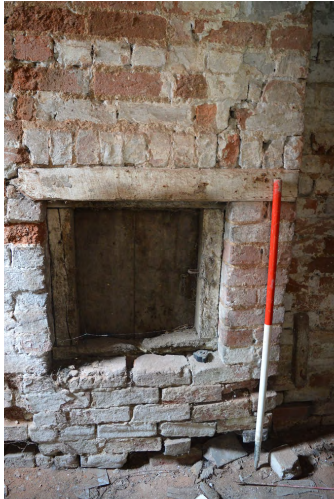
Plate 27. View west in half bay, to west of main building
