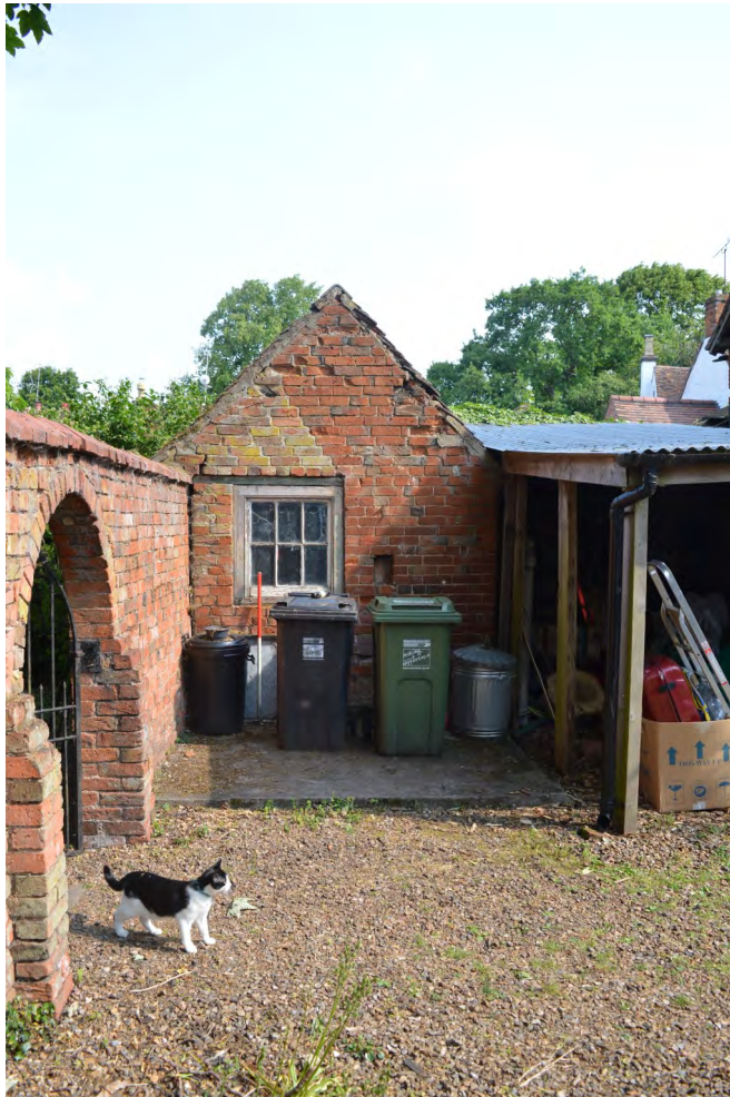
Plate 9. Brick building to west of lean-to, view north
