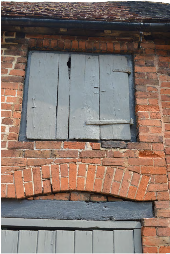
Plate 5. Segmental arch of former opening, view north
