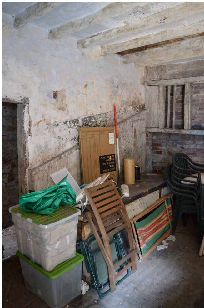
Plate 22. Remnants of manger and side of loose box in Room 2, view north-west
