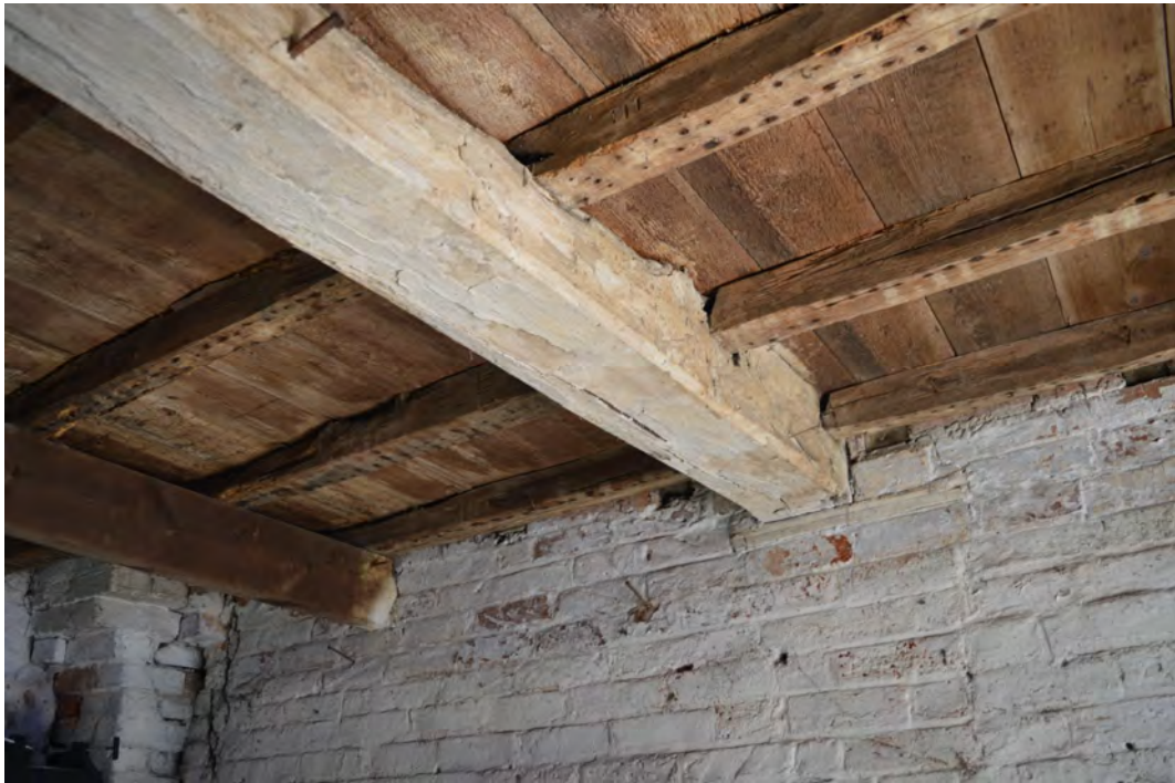
Plate 15. Beam in Room 1, view north-east
