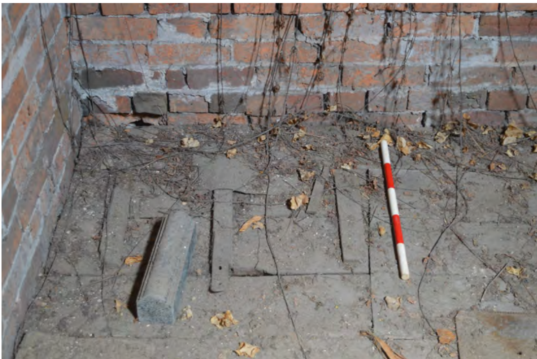
Plate 34. View north in north-western corner of Room 5, scale 0.50m
