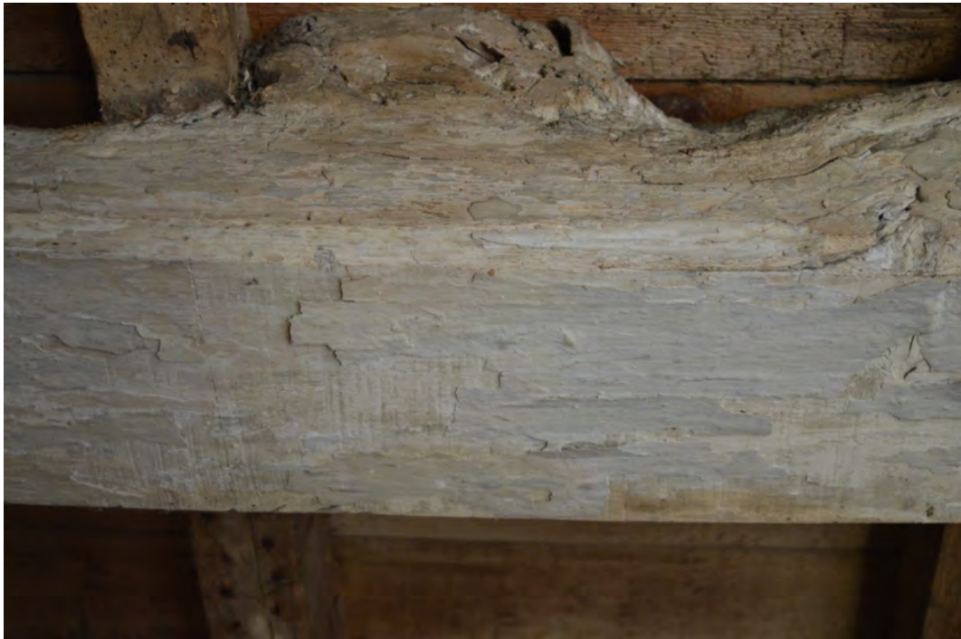
Plate 16. Pit saw marks on beam in Room 1
