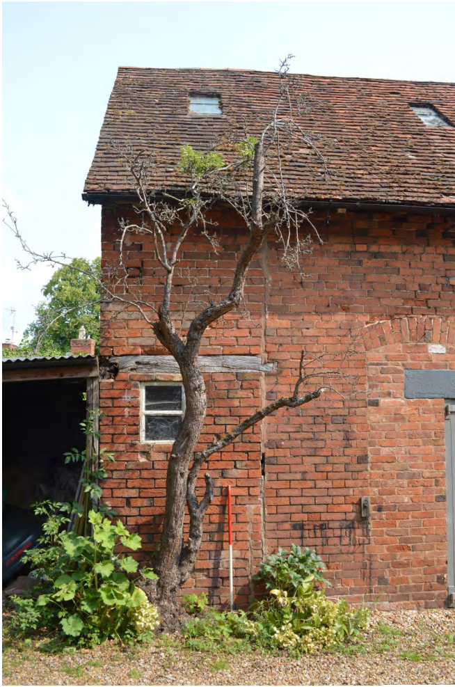
Plate 7. View north to added half bay
