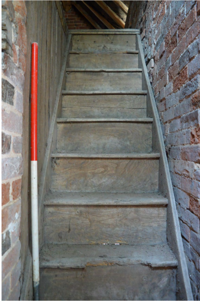
Plate 29. Stairwell to first floor, view east
