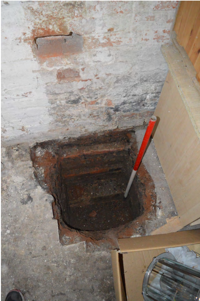
Plate 19. Trial pit in northern part of Room 1, showing brick foundation
