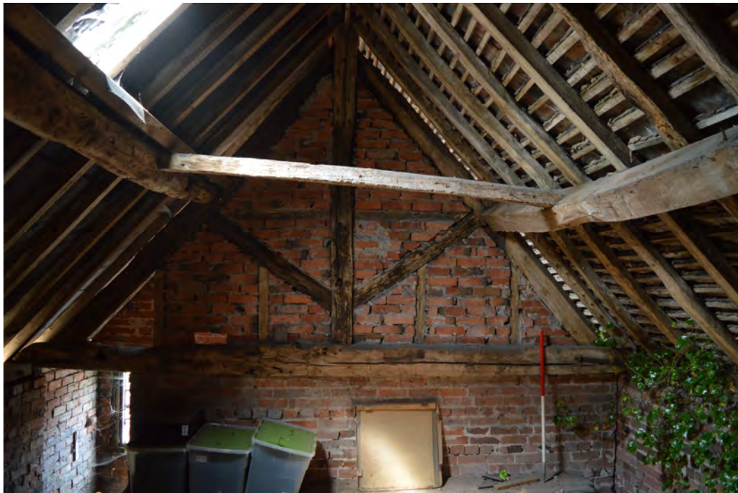
Plate 30. View west in Room 3
