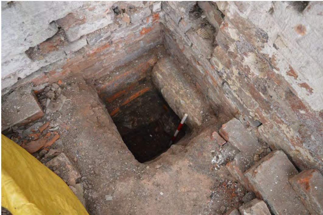
Plate 25. View north-east in Room 2 showing foundations exposed in Trial Pit, scale 0.50m
