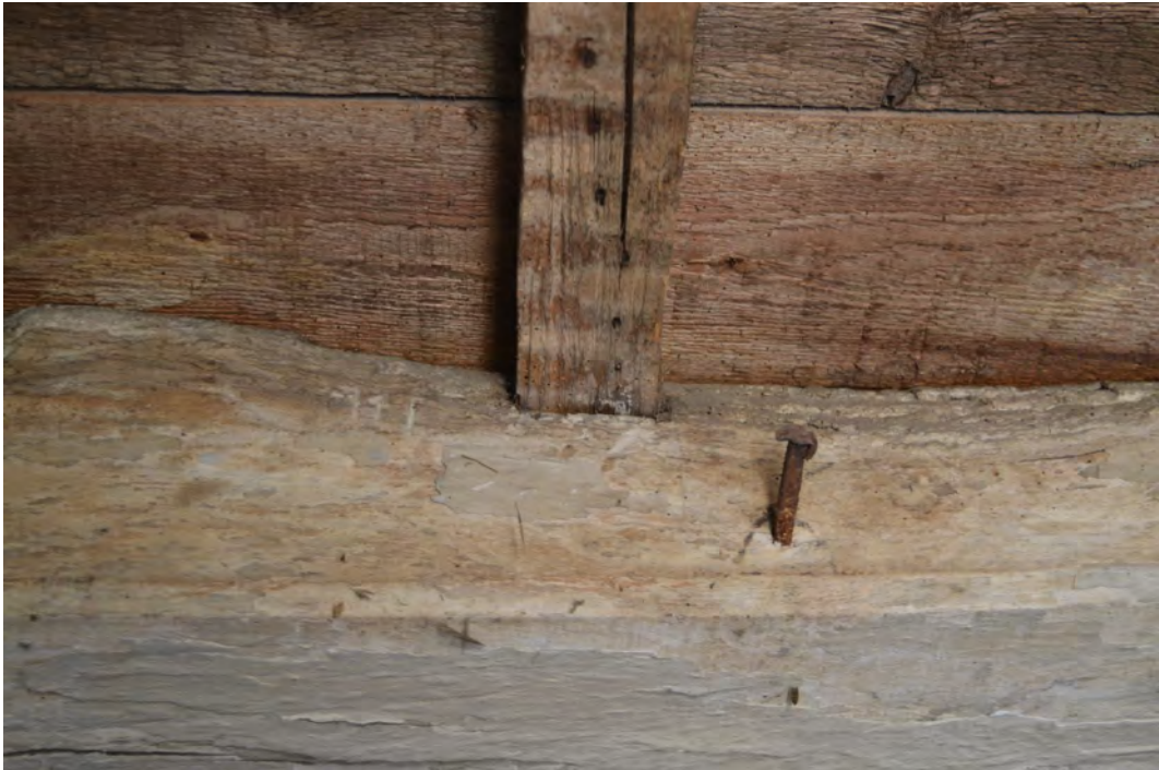
Plate 17. Carpenter's marks and blacksmith's nail, Room 1
