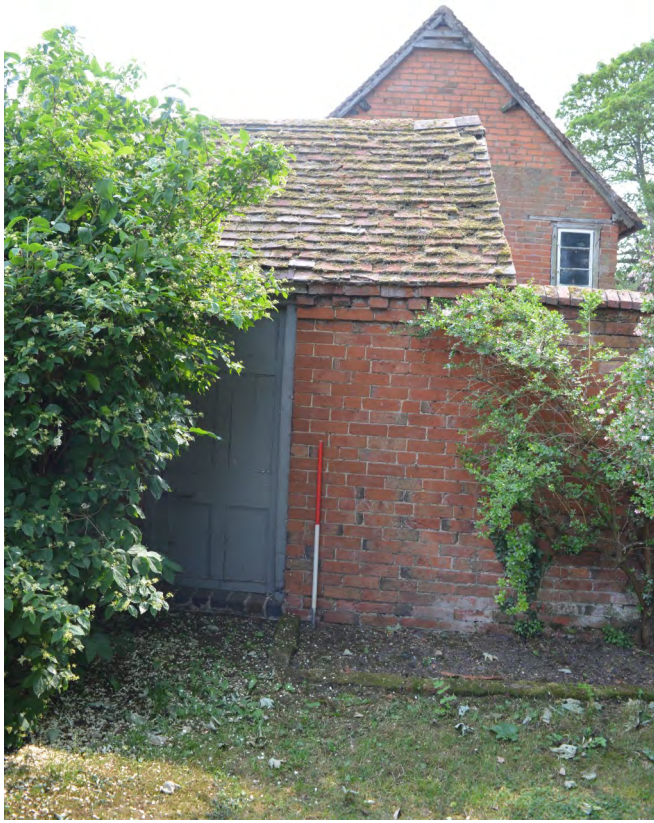
Plate 13. Western gable of stable building behind brick garden wall and shed
