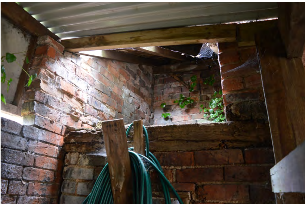
Plate 12. View east in north-western corner of the building
