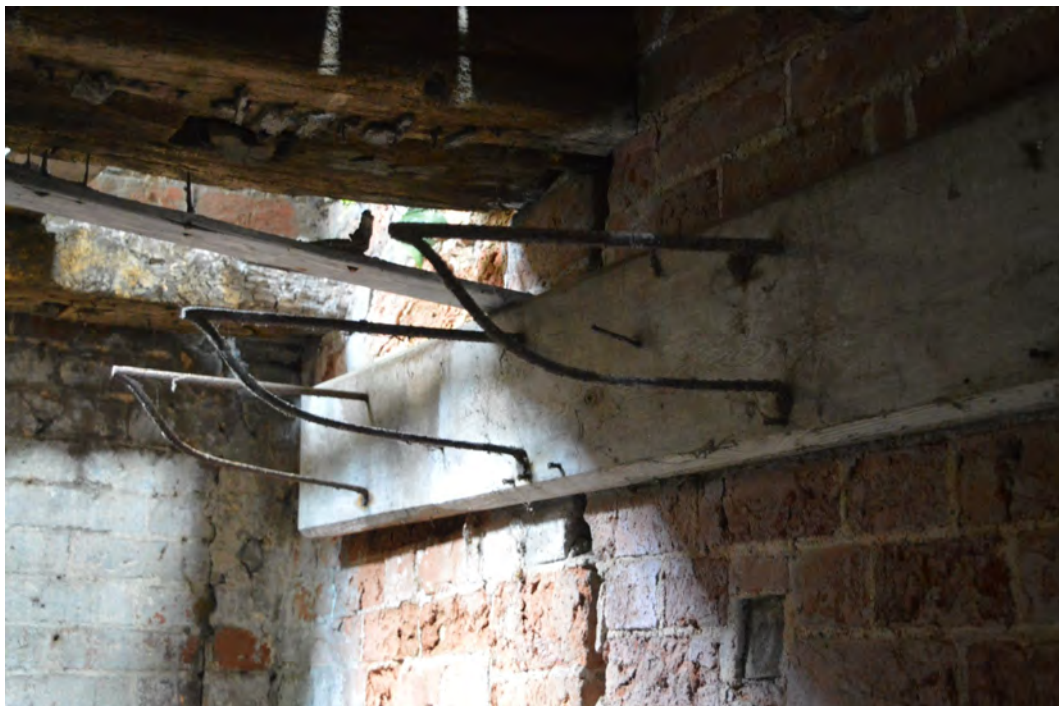
Plate 28. View north east in half bay to west of main building
