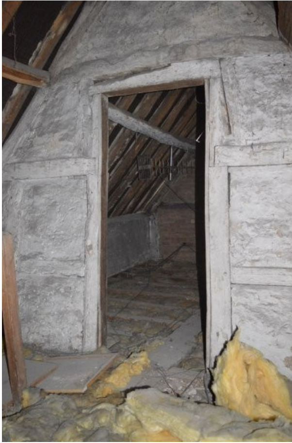
Plate 67. Partition to space above northern rear extension, view north-east
