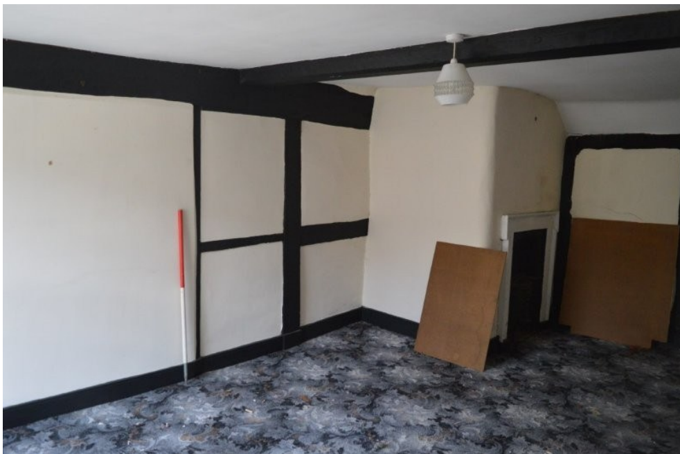
Plate 44. Room 12, view north-east
