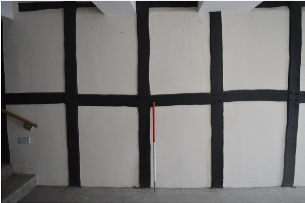
Plate 15. Box framing in south wall of Room 2, view south
