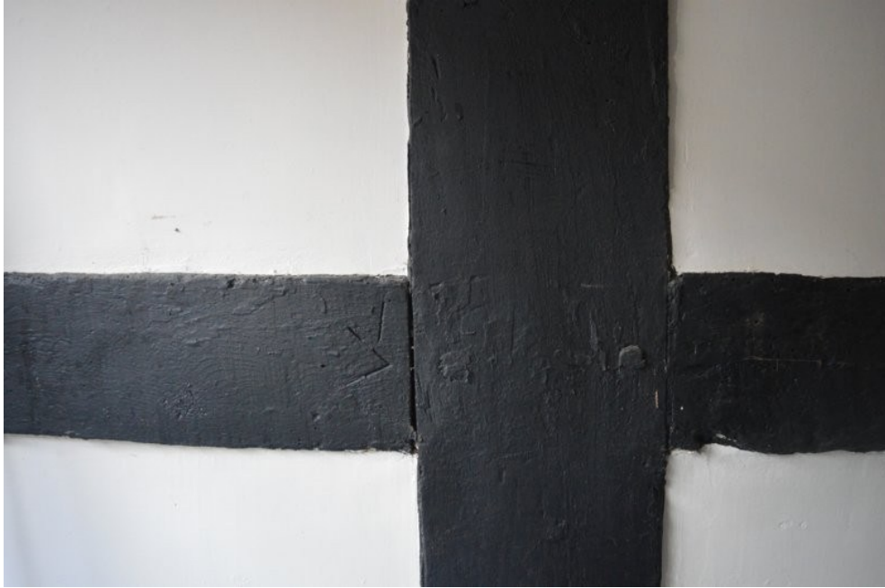
Plate 53. Carpenters' marks, west wall of Room 15
