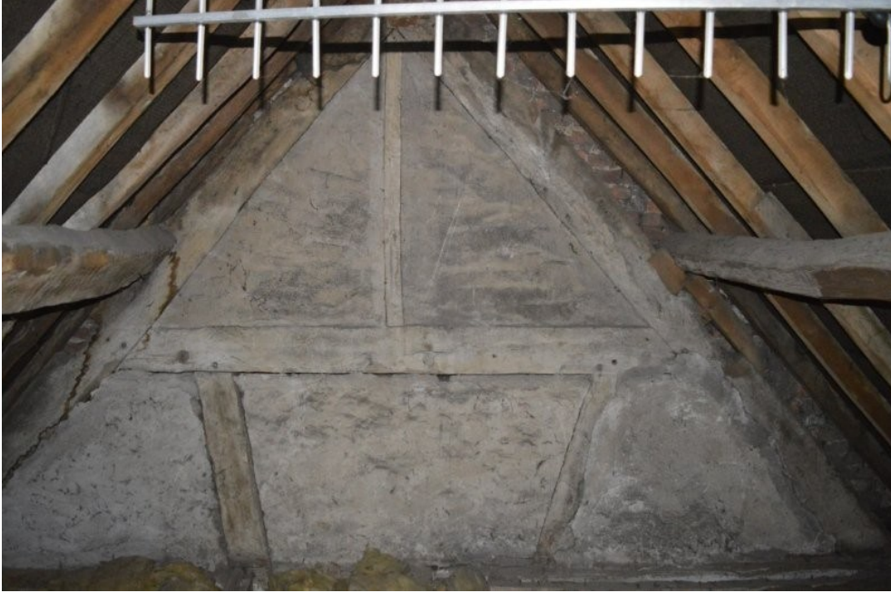
Plate 71. Southern truss in main axis of building, view south
