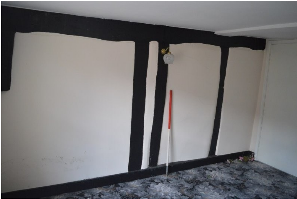
Plate 43. Room 11, view north-east
