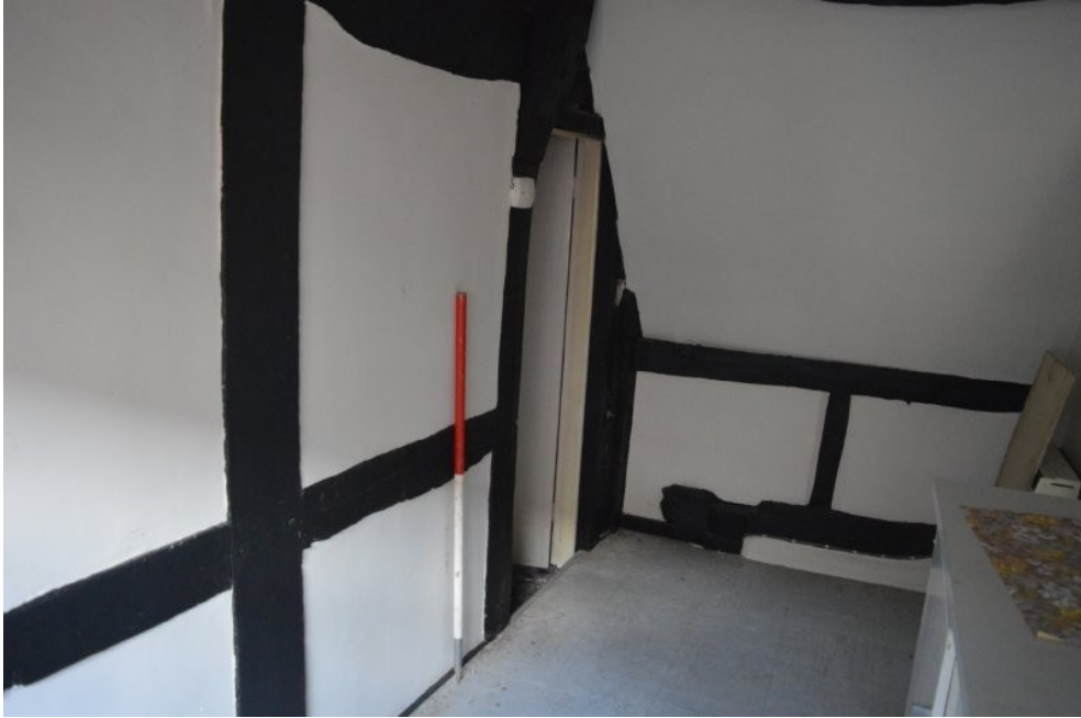
Plate 51. Room 15, view WNW
