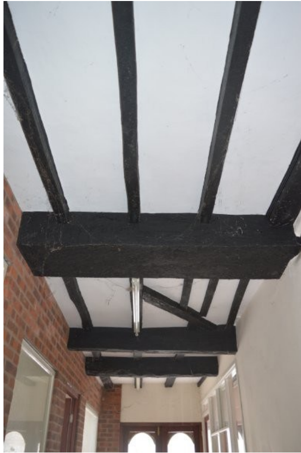
Plate 13. Axial beams crossing Room 1, view west
