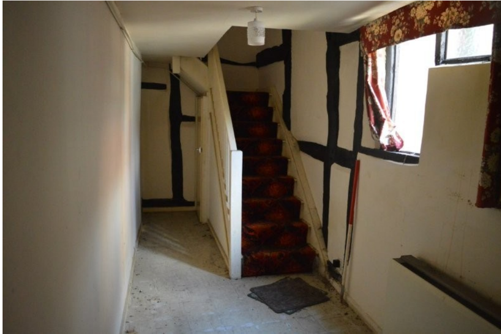
Plate 27. Room 5, view WNW
