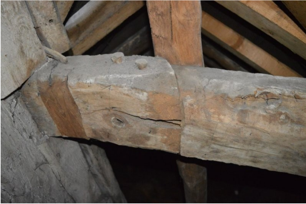
Plate 73. Pegged scarf joint in area over southern rear extension
