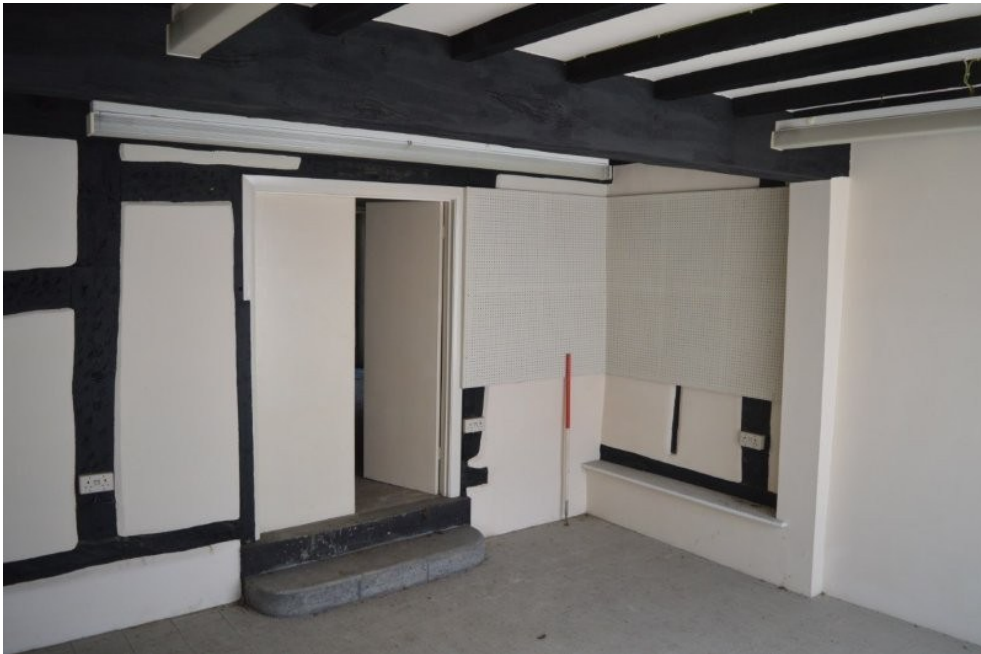
Plate 24. Room 4, view south-east
