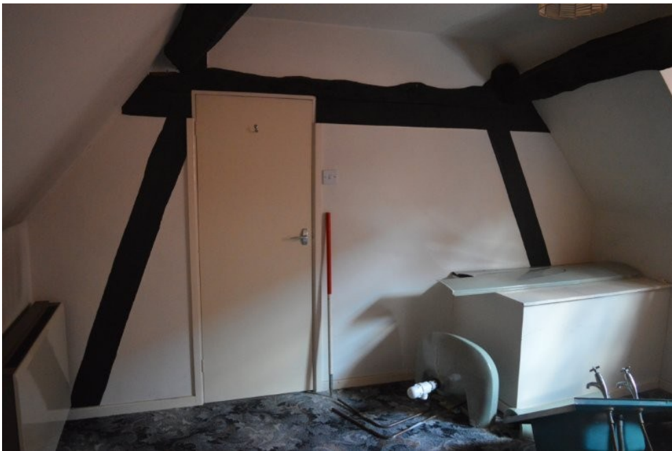
Plate 56. East wall of Room 15, view ESE
