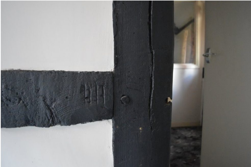
Plate 52. Carpenters' marks, west wall of Room 15, view west
