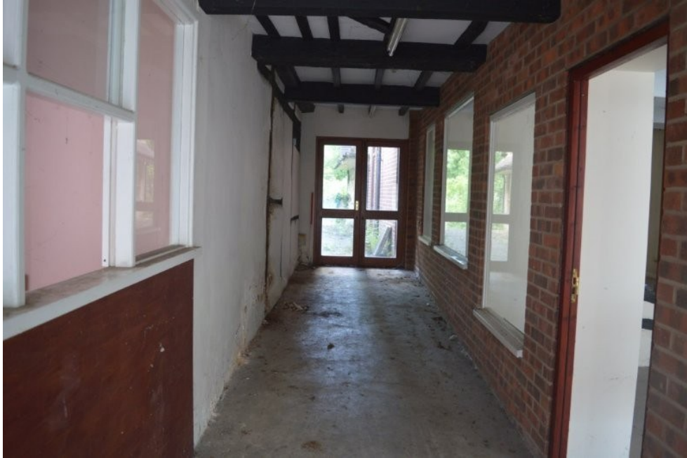
Plate 9. Central corridor, Room 1, view east
