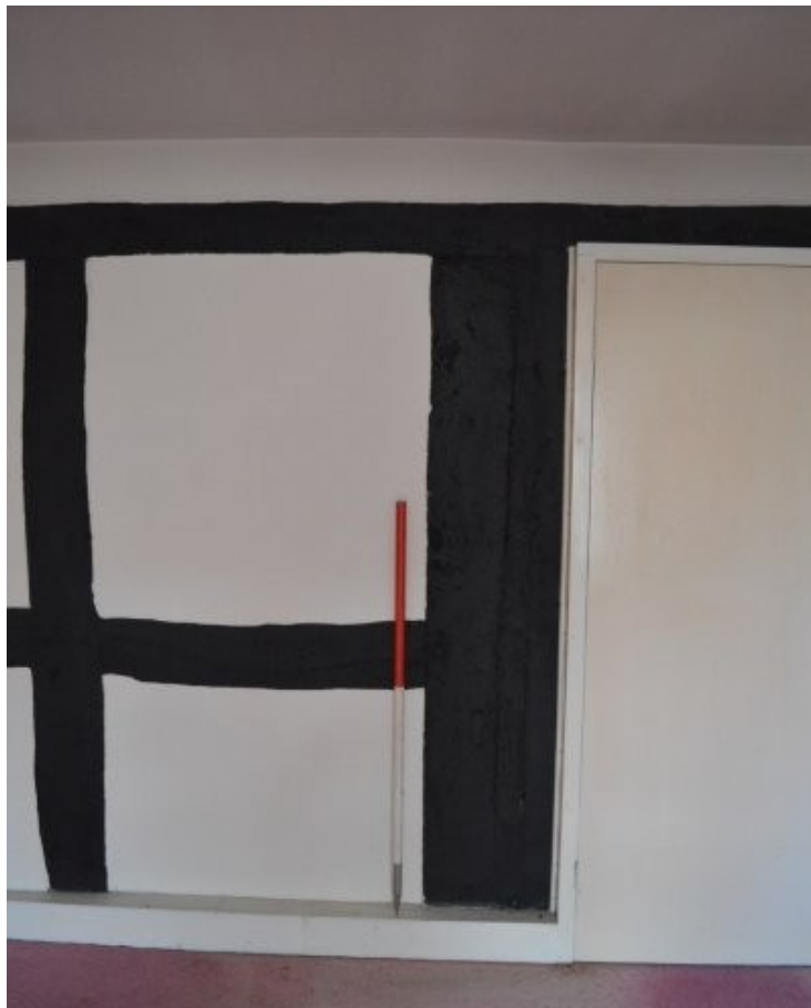
Plate 34. Large post in east wall of Room 7
