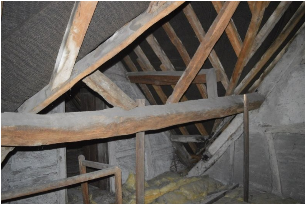
Plate 65. View south-east toward rear extension in northern attic space
