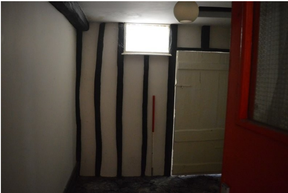
Plate 38. West wall of Room 9, view west
