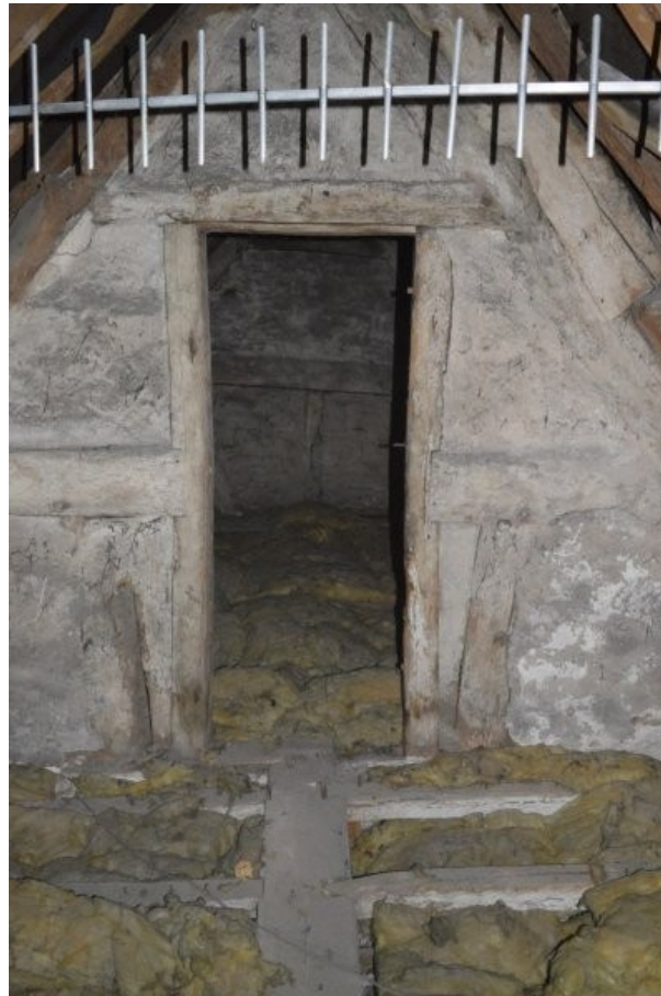
Plate 70. Central partition in southern attic space
