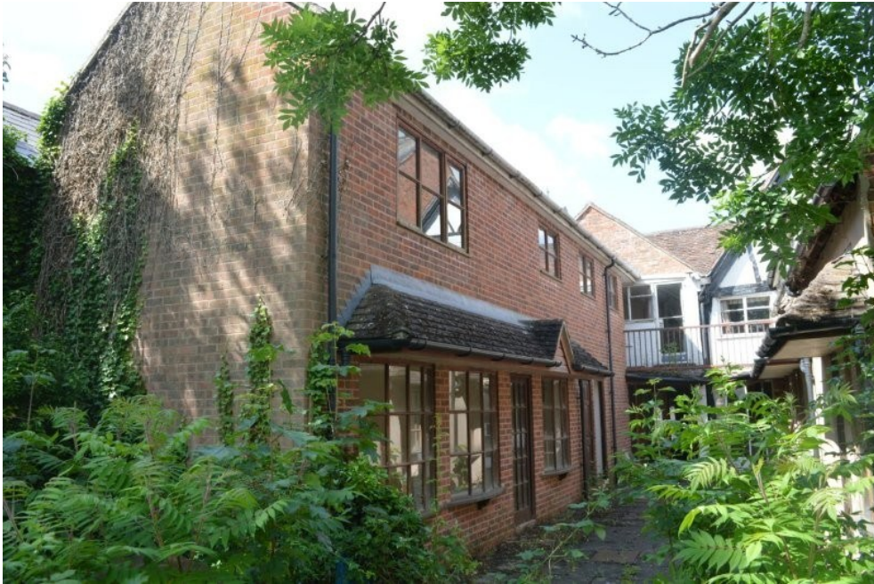
Plate 5. North and east elevations of the 1980s southern range, view WSW
