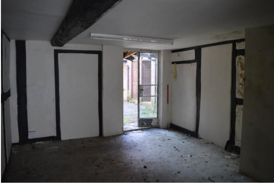
Plate 21. Room 3, view south-east
