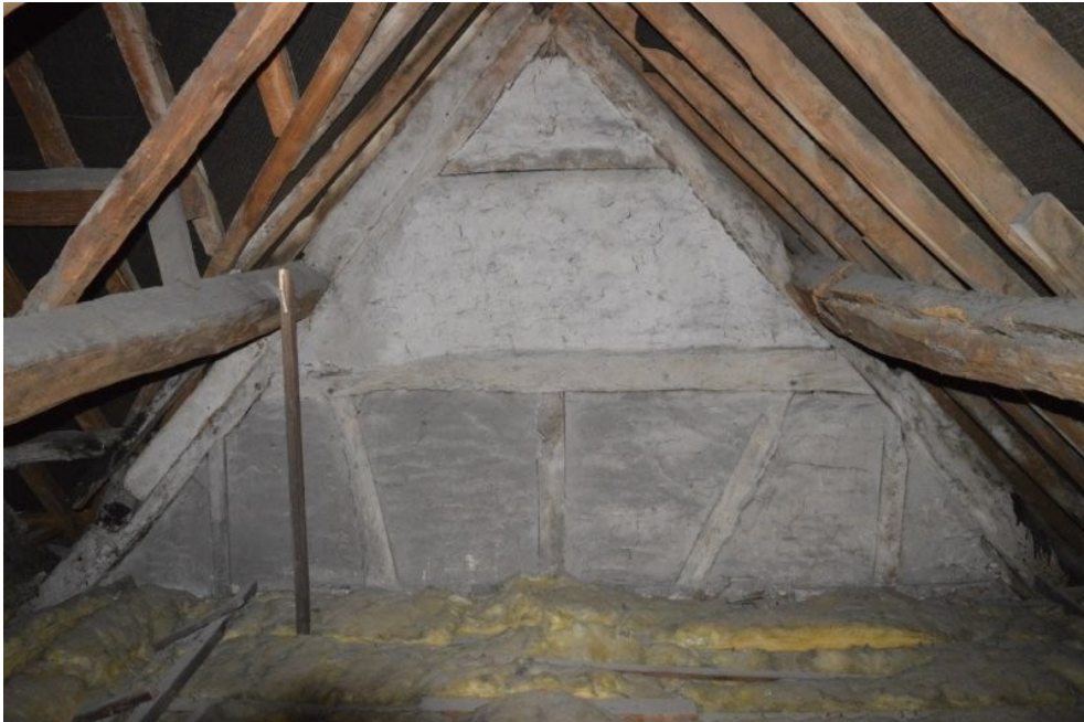
Plate 64. View south in northern attic space
