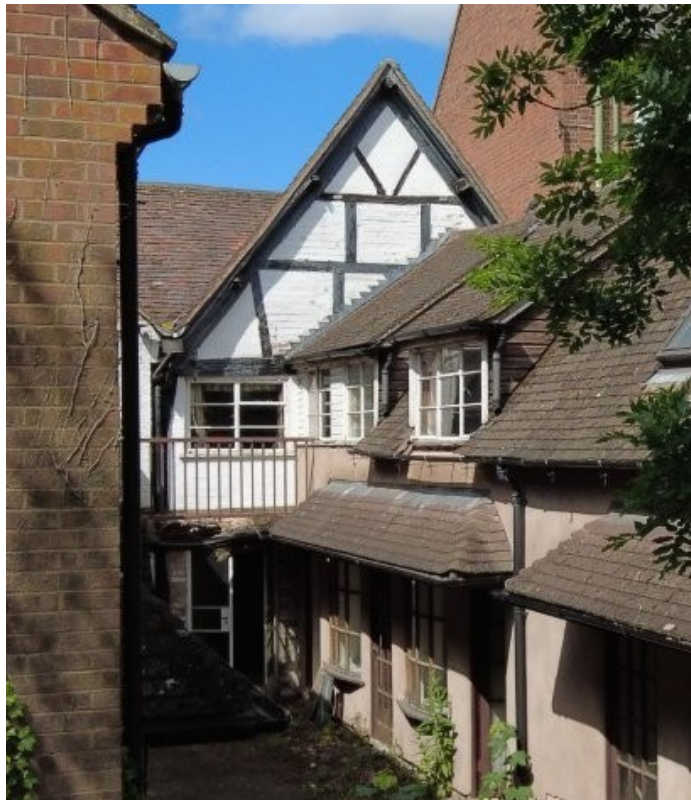
Plate 6. East facing gable end of northern extension
