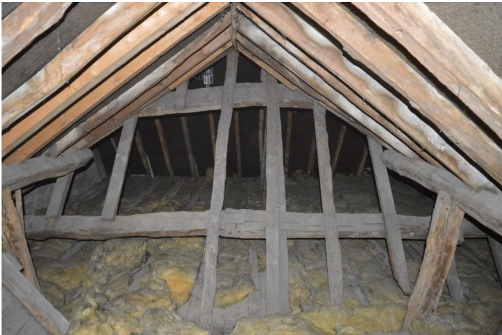
Plate 72. Roof structure of original house preserved within southern rear extension
