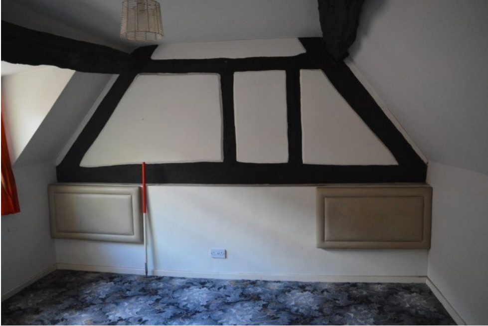
Plate 55. West wall of Room 18, view west
