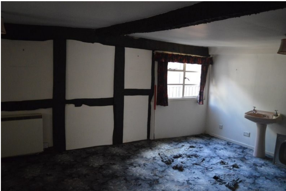
Plate 30. Room 6, view south-east
