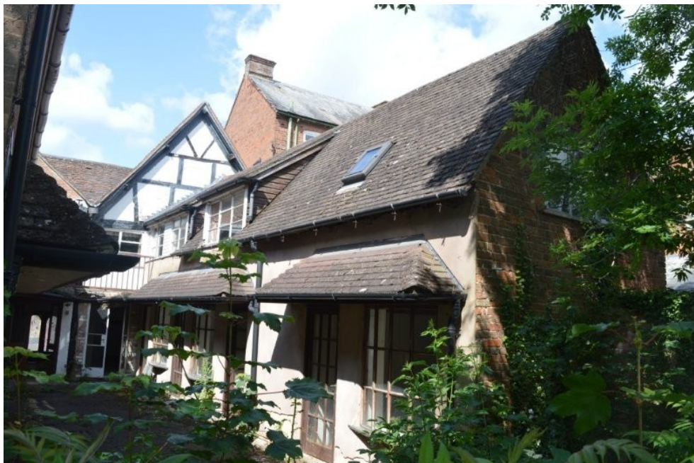
Plate 8. South elevation of northern range
