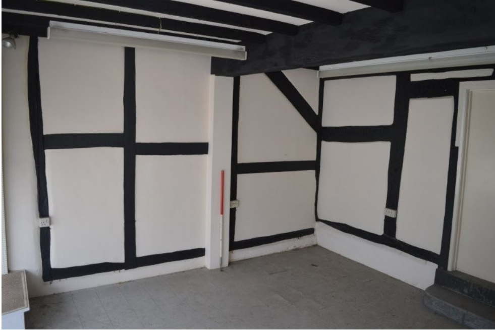
Plate 23. Room 4, view north-east
