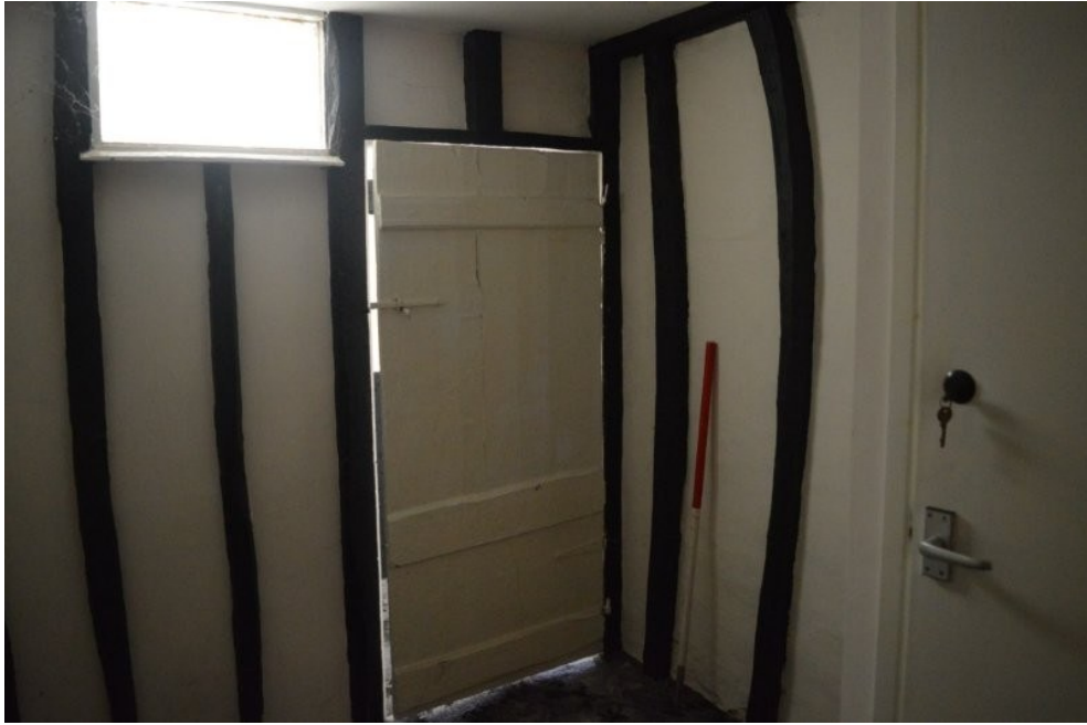
Plate 39. Room 9, view WNW
