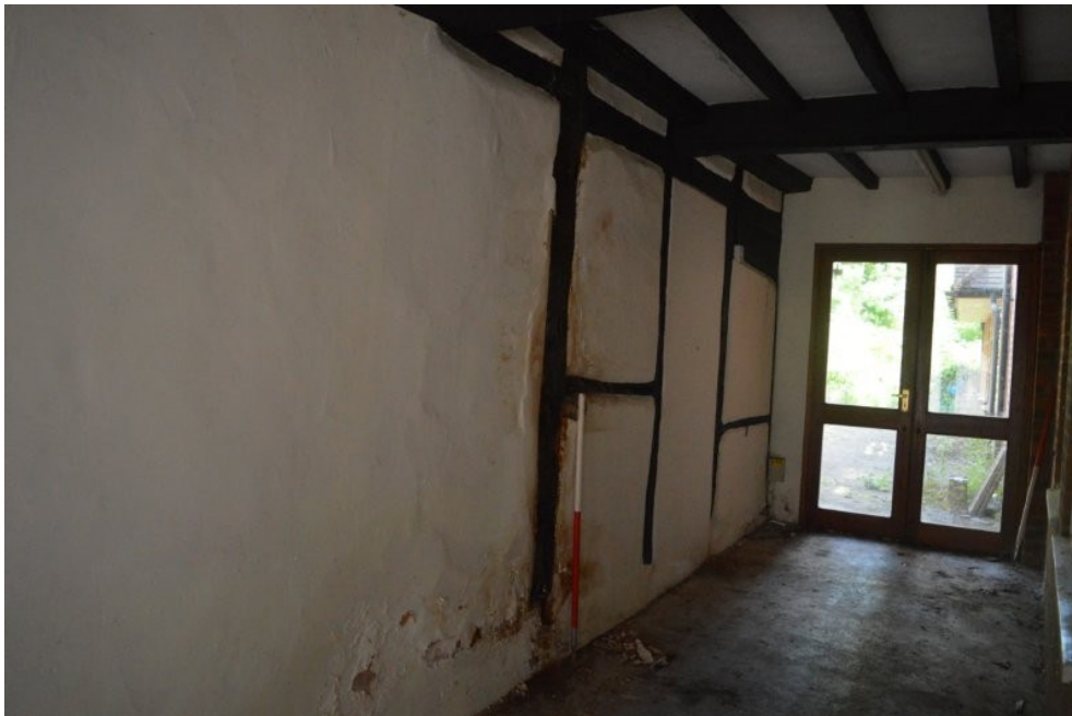
Plate 12. box framing in north wall of Room 1, View ENE
