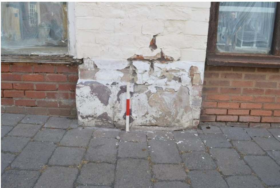
Plate 2. Stone base to brick pillar, view east, scale 0.30m
