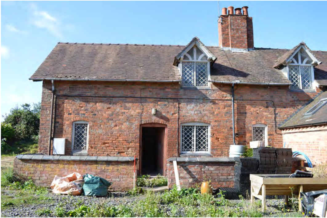
Plate 5. North-east elevation of No. 123 Pensax
