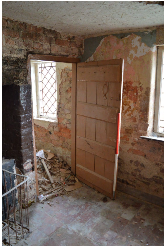
Plate 23. View north in Room A towards small store room between chimney and front wall
