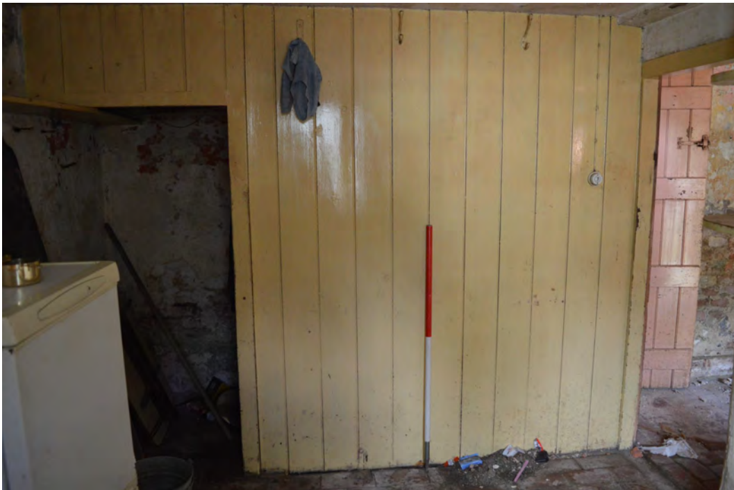
Plate 26. View south-west in Room B
