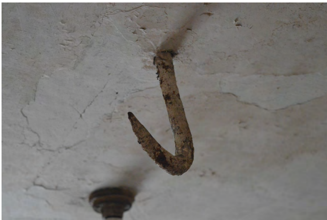
Plate 29. Hook in ceiling, Room B
