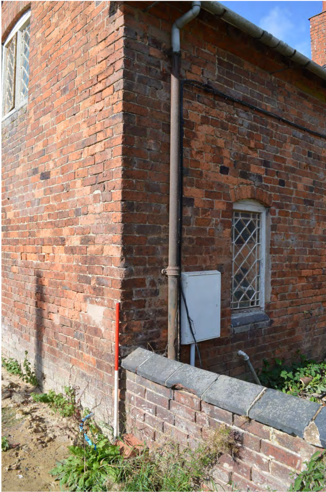
Plate 7. View west of No. 123 with wall to front
