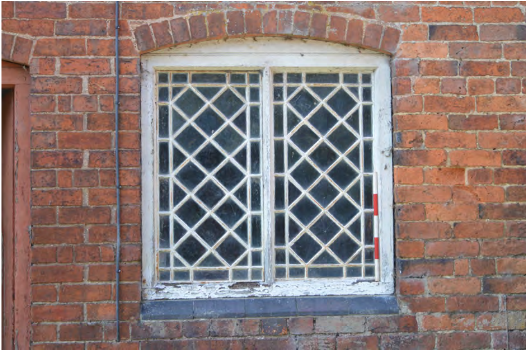
Plate 11. Casement window in main elevation
