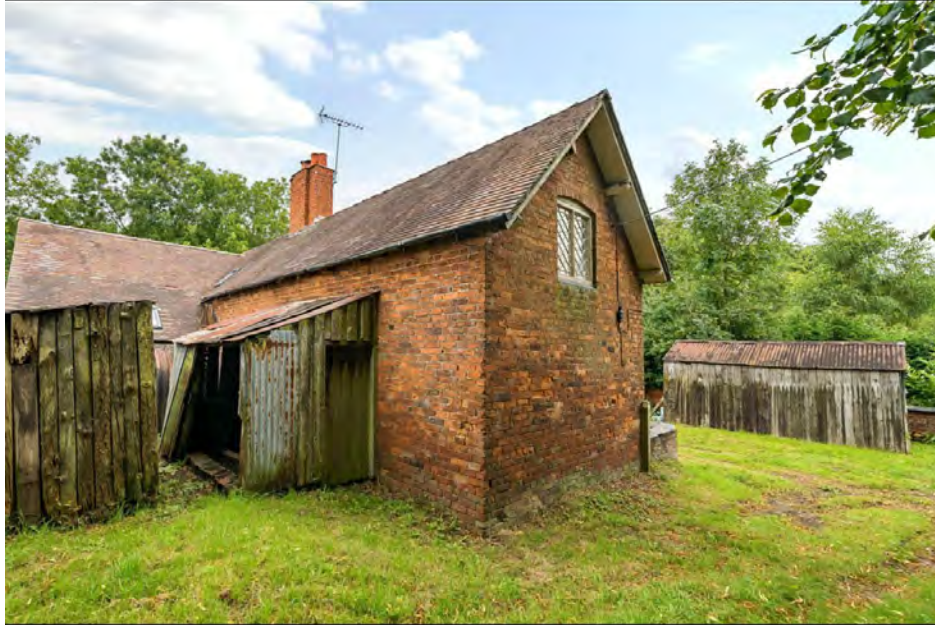
Plate 3. Former outhouses to rear of No. 123 Pensax. Photograph provided by the client
