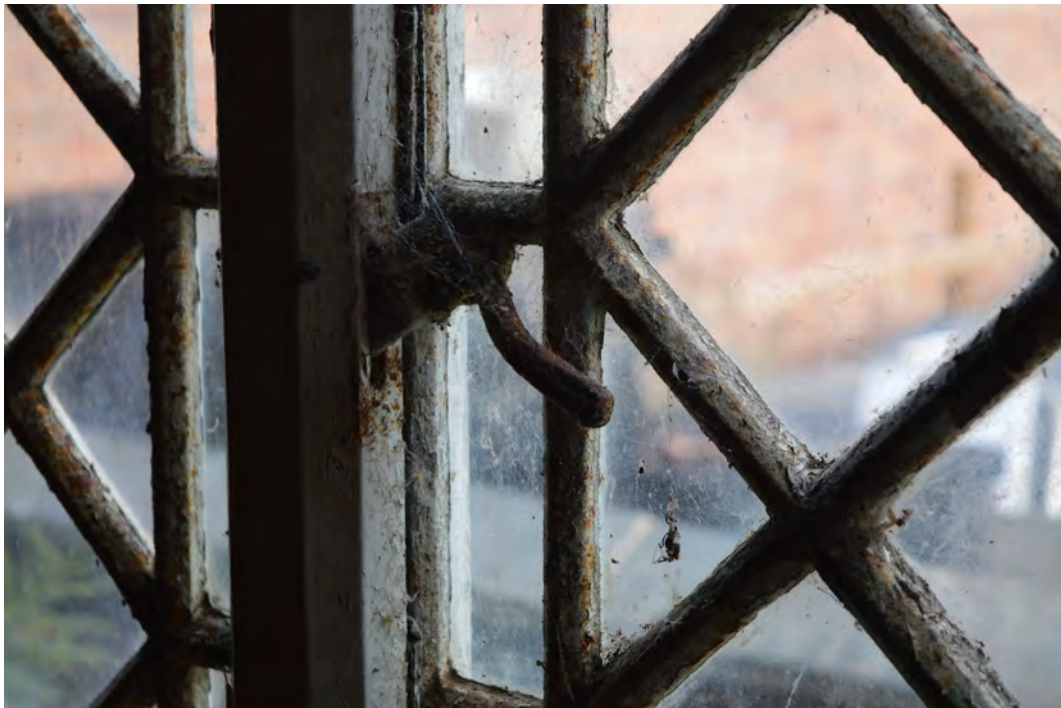
Plate 22. Detail of interior of casement window in Room A
