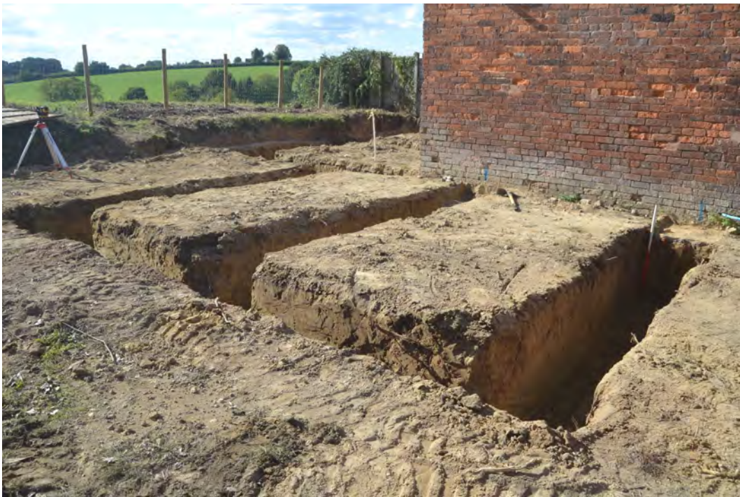
Plate 46. View west of foundations fully excavated
