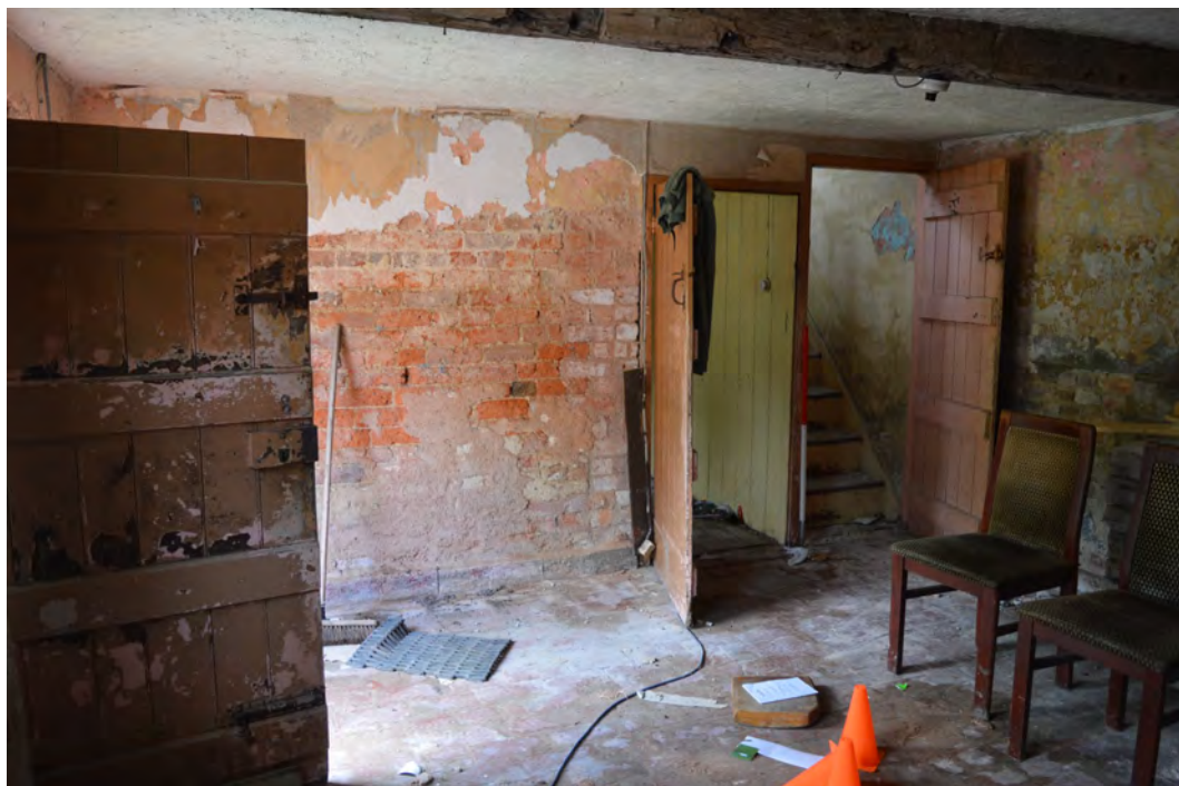
Plate 24. View south-east in Room A towards doors to Kitchen (Room B) and Stairwell
