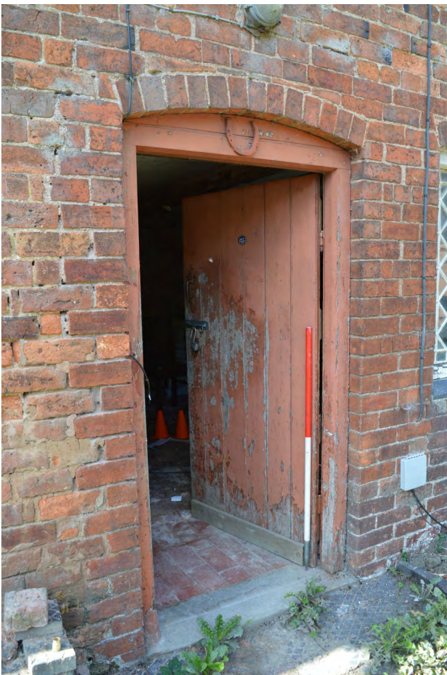
Plate 10. View north-west to front door of No. 123
