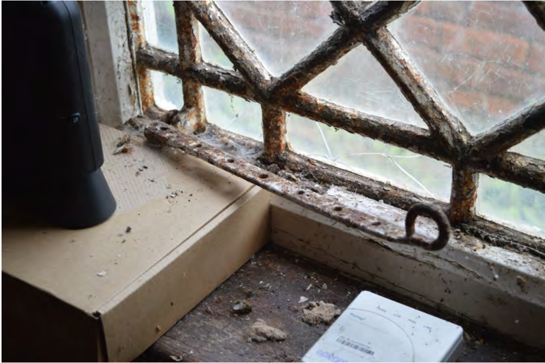
Plate 21. Detail of interior of casement window in Room A
