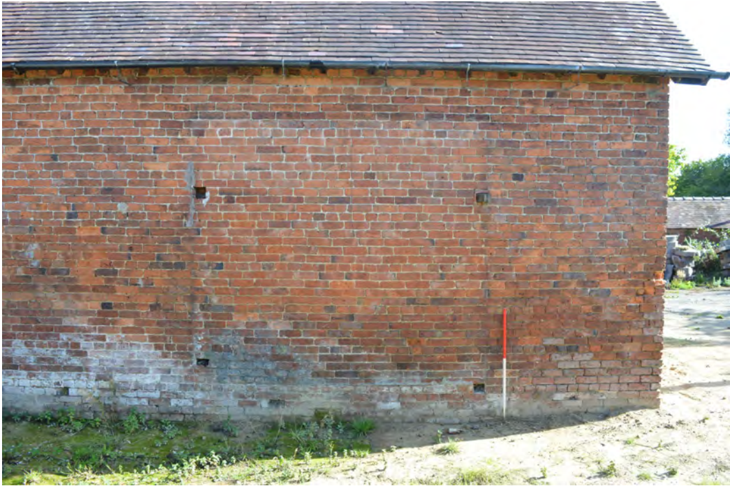
Plate 13. Rear elevation of No. 123, showing scar of former lean-to outbuilding
