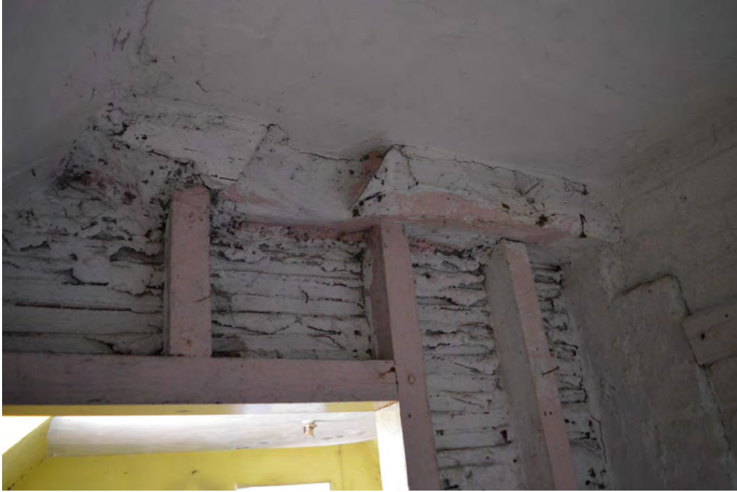
Plate 39. View south in cupboard in Room D
