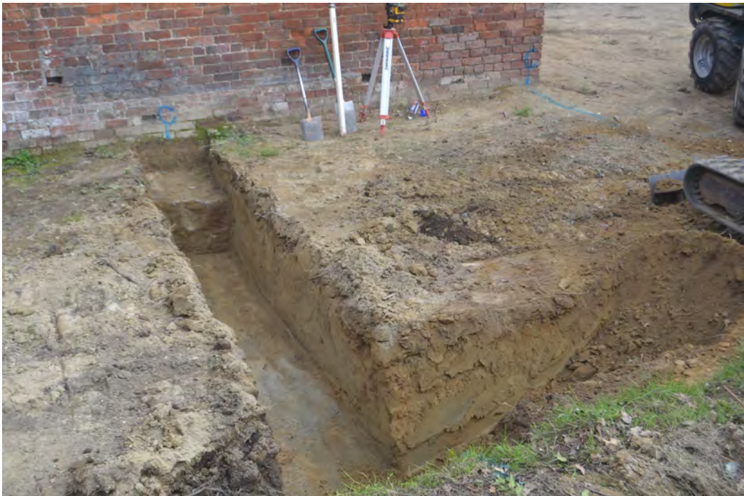
Plate 42. View east toward former concrete underpinning (106)
