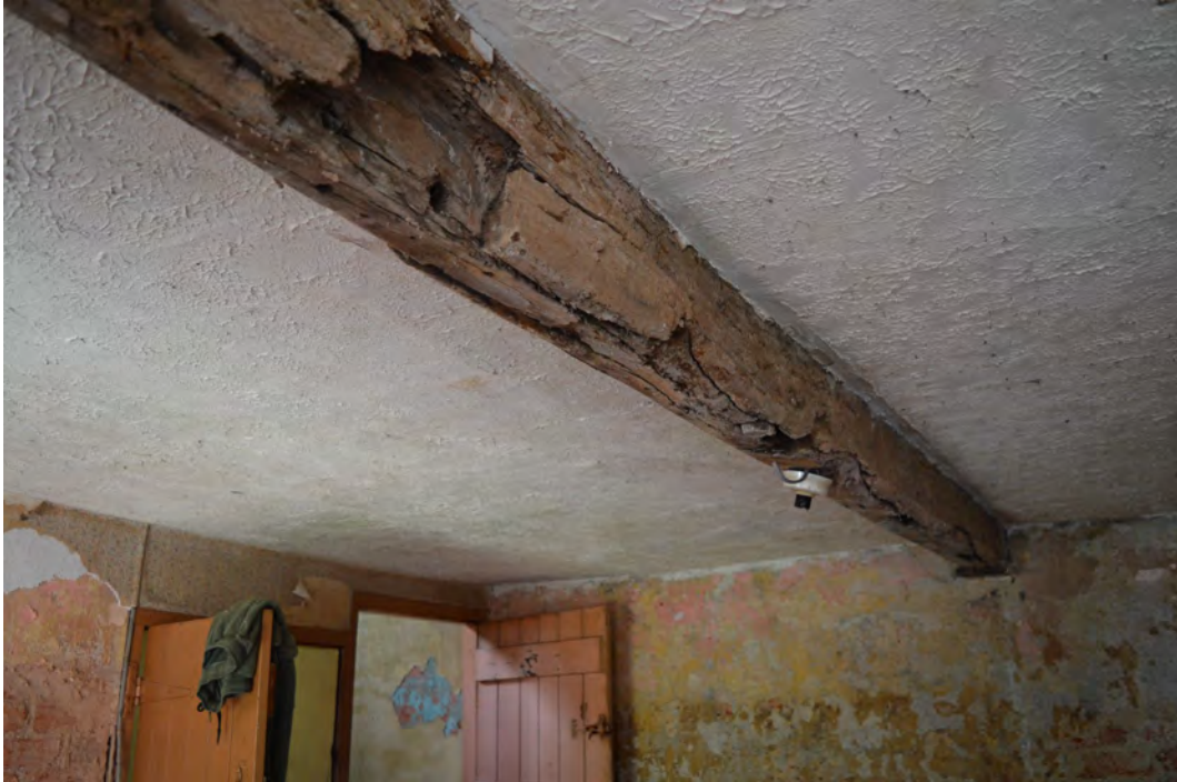
Plate 16. Transverse beam in Room A, view south-west
