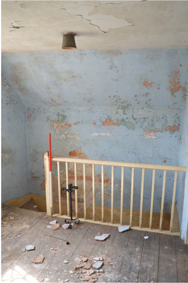
Plate 31. View south-west in Room C
