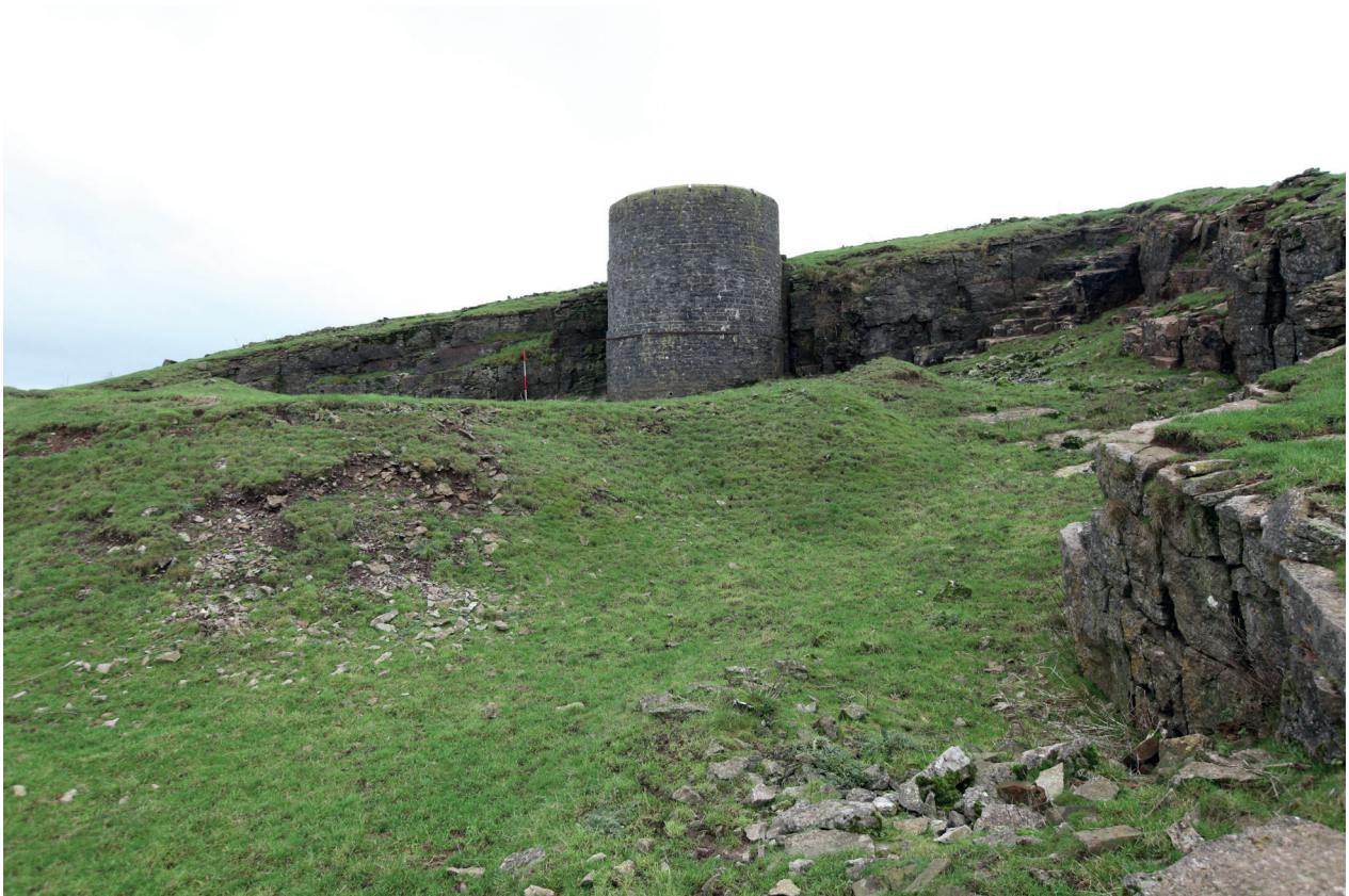
Plate 10 (ref. ext13_02_01_22) View of the tower built into the east face of the quarry. To the immediate left is the rubble base of the former limekiln, which has been largely dismantled, leaving a platform. It seems highly likely that the highly durable carboniferous limestone stones for the limekiln were robbed out and re-used for the tower.
