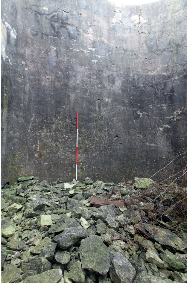
Plate 24 (ref.int02_02_01_22) Junction of rubble floor and rendered walls
