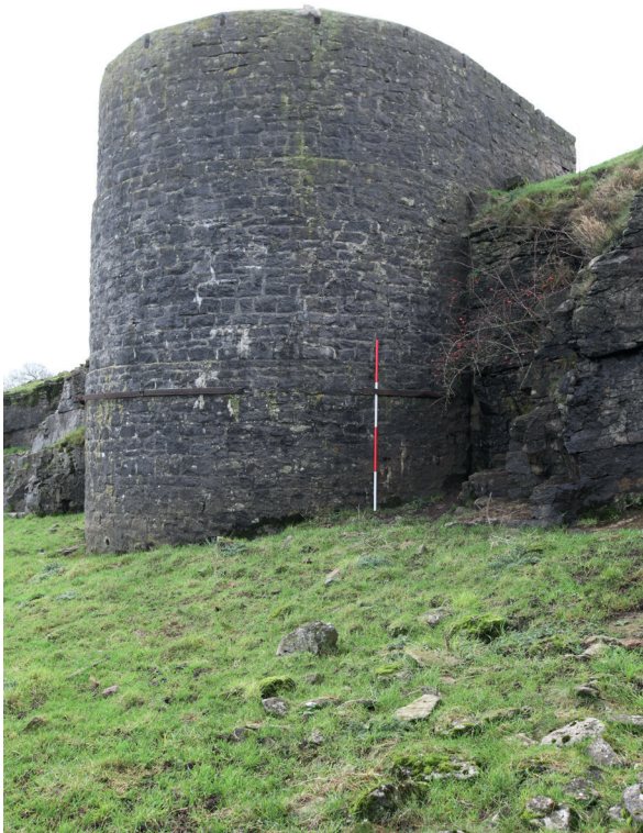
Plate 8 (ref. ext01_02_01_22) The tower from the north, built into the quarry face, which appears to have been deliberately part-removed to accommodate this structure.
