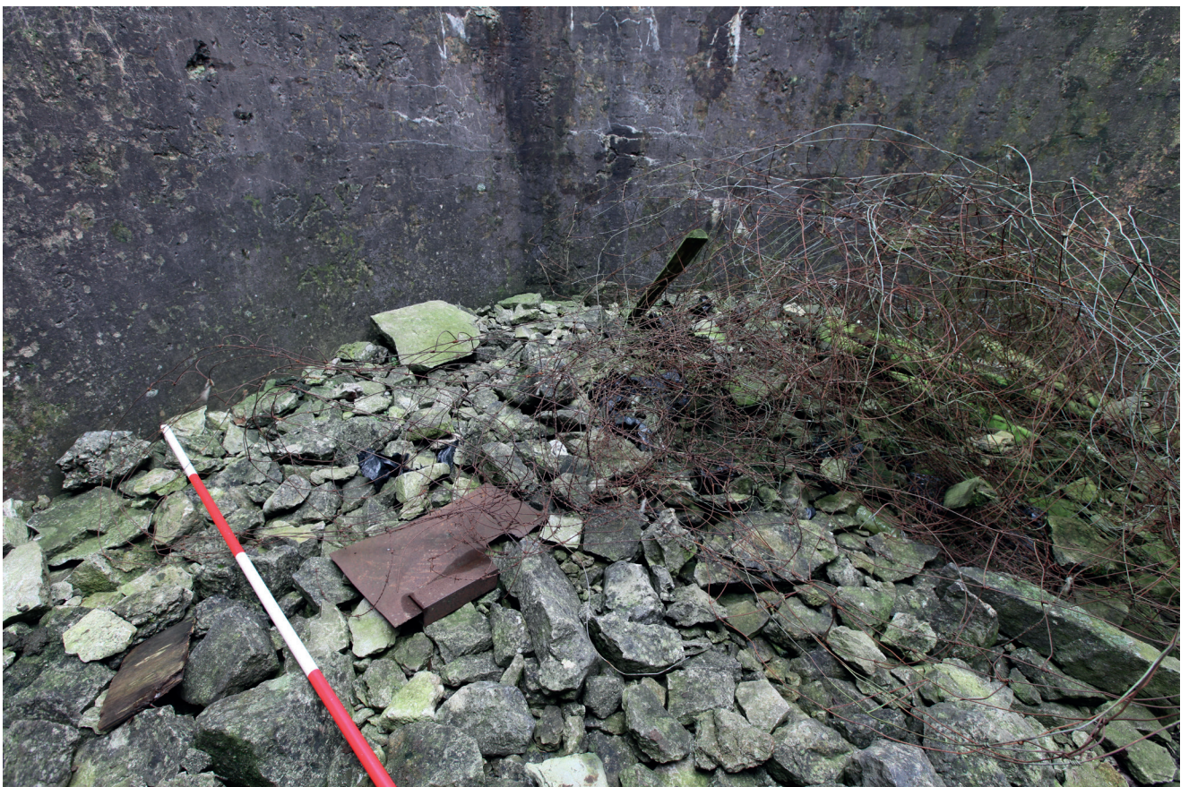
Plate 26 (ref.int07_02_01_22) - rubble stone floor
