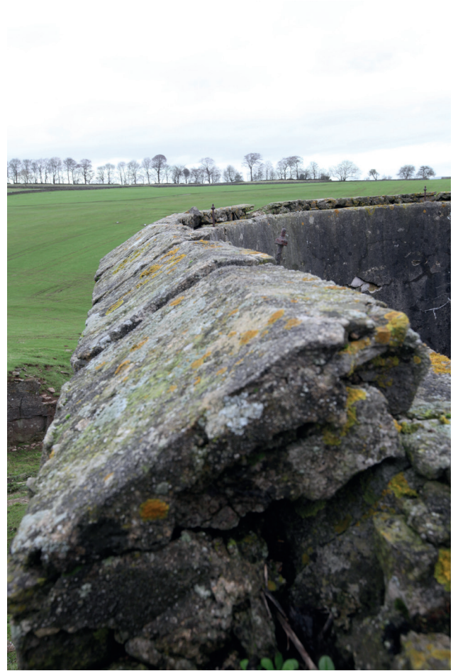
Plate 25 (ref.int12_02_01_22) Location of internal wall-plate and threaded bolts
