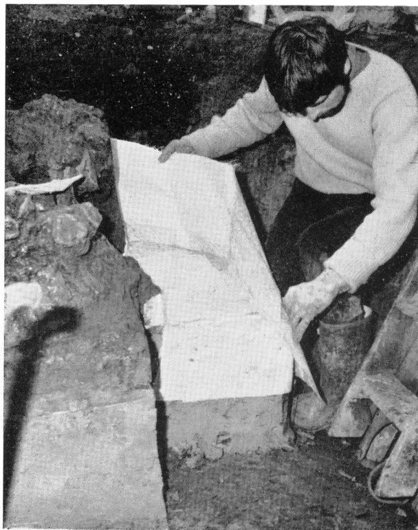
Stage 5—Making a glass-fibre cast of the foundation.
