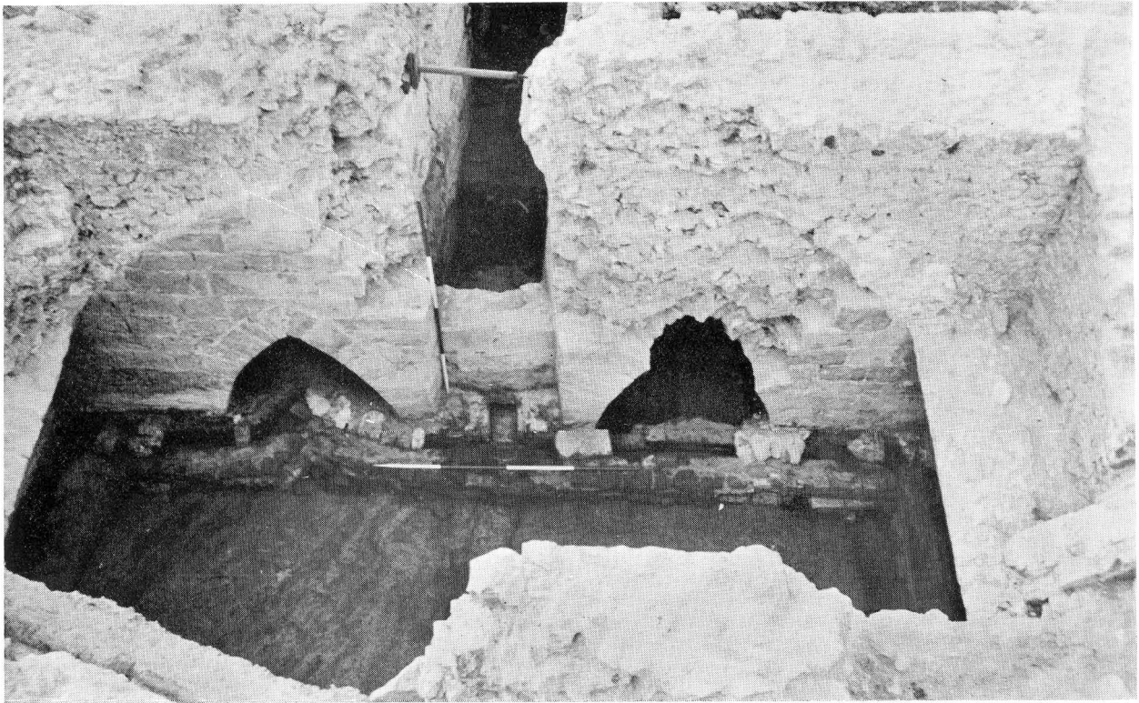
Fig. 3: The western end of the undercroft, showing the relieving arches, the springers of the vault and the ghost of the vault itself, the doorway and drains.
