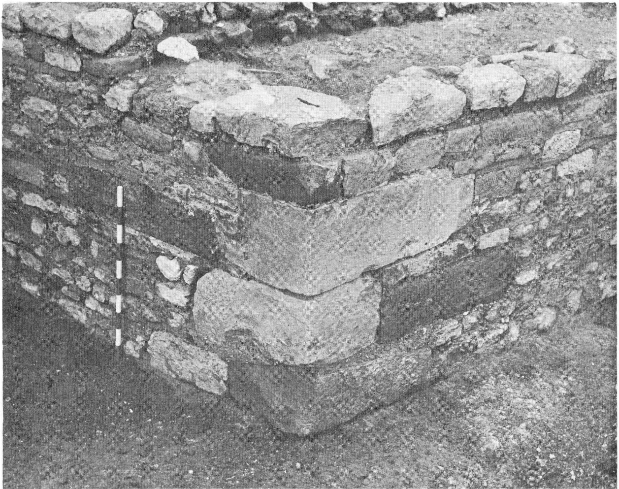
Fig. 2: corner showing re-used architectural stone.
