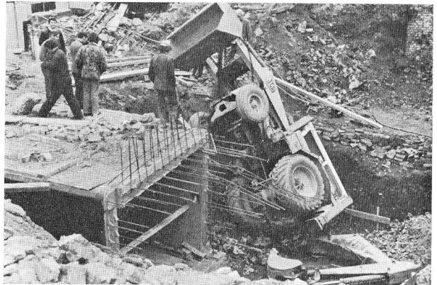
Fig 2: Collapsed J.C.B. in Area 2.
