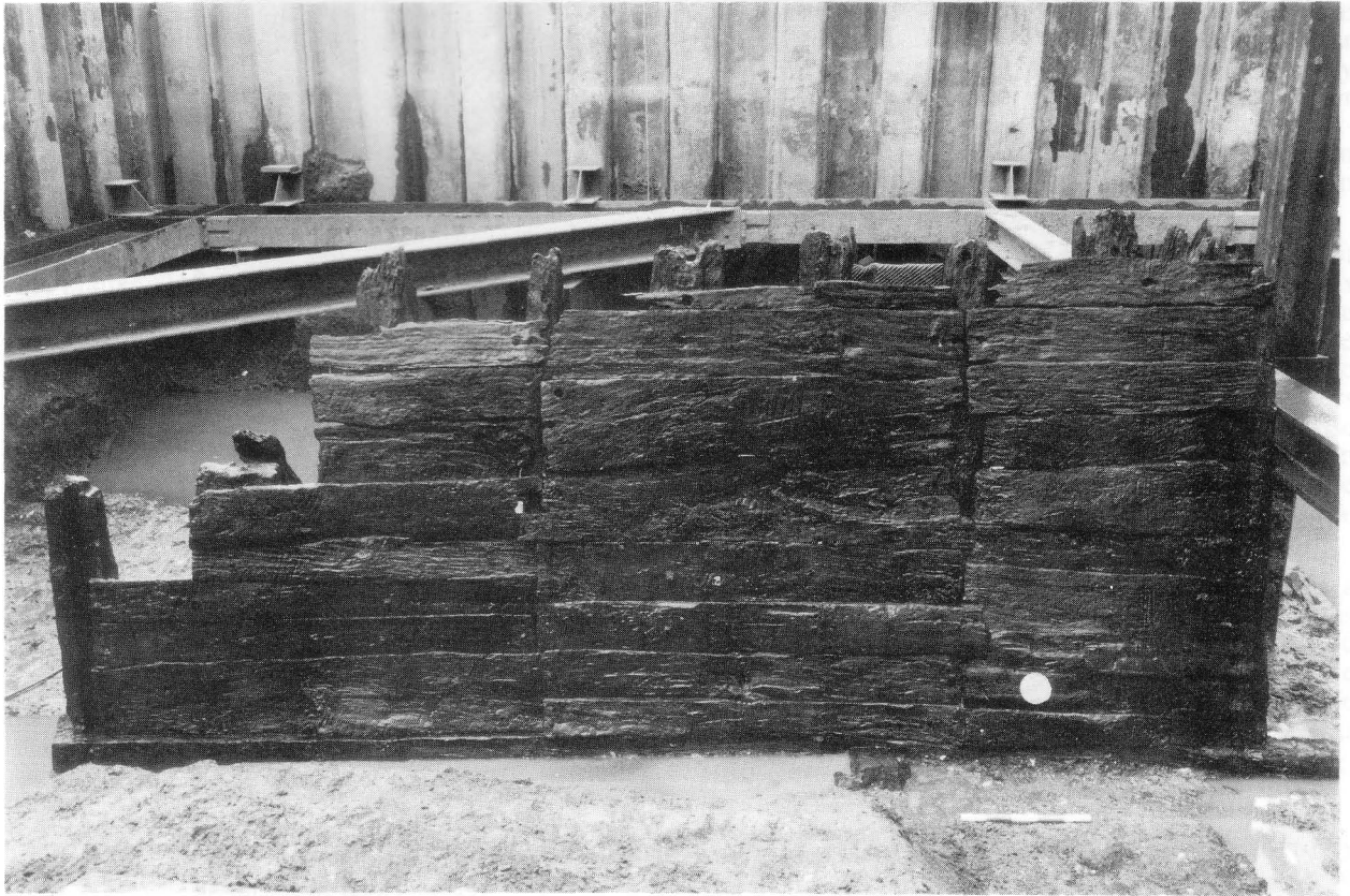
Fig. 1: View of the Billingsgate waterfront in situ . Note the carpenter's mark on the planking. The timber in Fig. 2 is marked on the bottom right-hand side.
