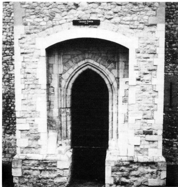
Fig. 6: view of the outside (south side) of the Cradle Tower.
