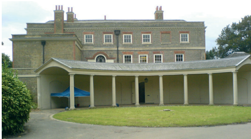
Fig. 2: photo of Valentines Mansion (south facing, showing porte-cochère)
