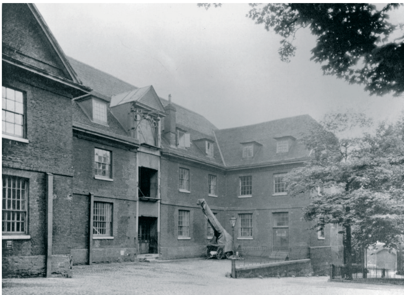
Fig. 2: the New Armouries viewed from the north-west in the 1920s. The original casement windows were replaced with sash opening during the 19th century and the high security brick wall that once screened the entrance and formed a courtyard in front of the building has all but disappeared (© Royal Armouries)
