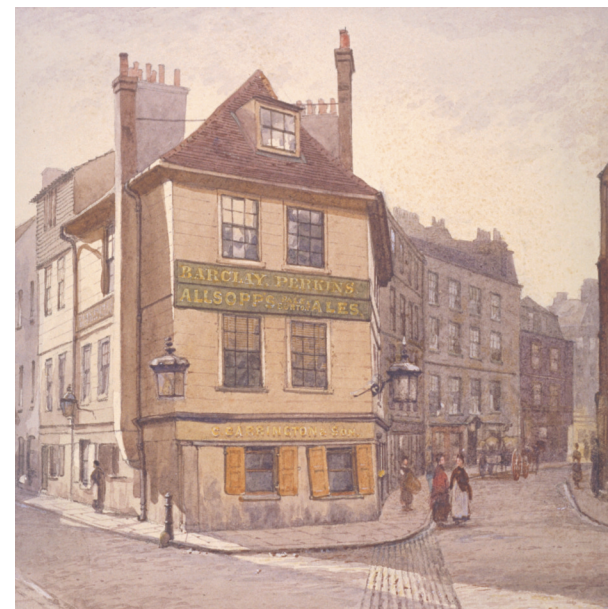
ABOVE Glass from 1820s cesspit clearance group ©MOLA RIGHT Corner of Fort Street and Gun Street in 1884 (London Metropolitan Archives, City of London, q803178x)
