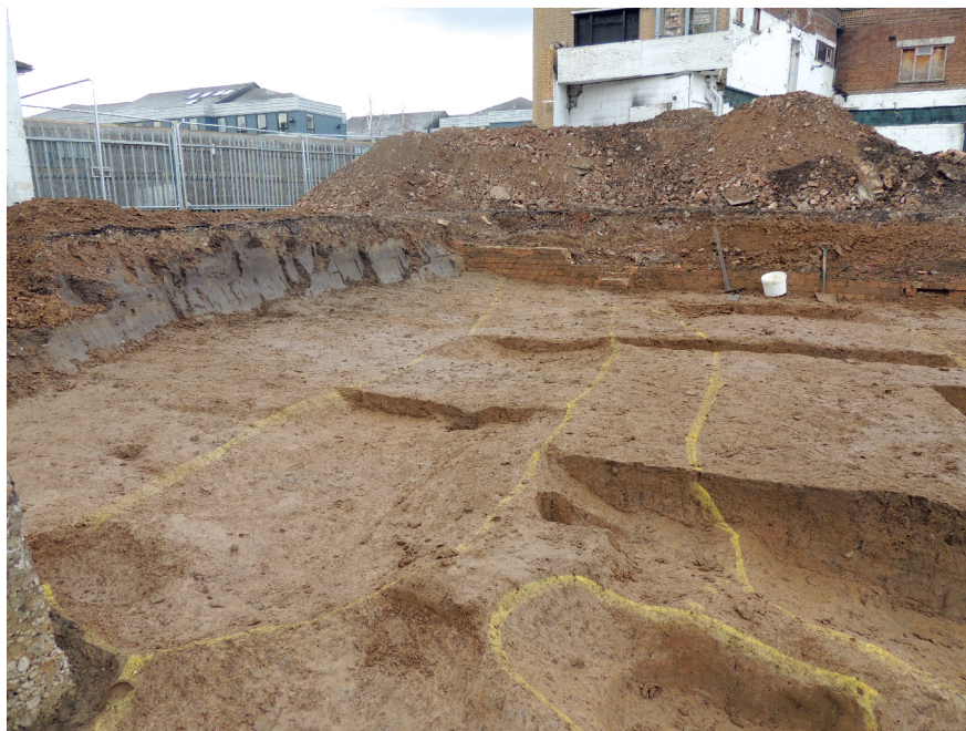
Fig. 3: photo of ditch termini, with posthole in the foreground. The edges of the features have been outlined with yellow spray marking
