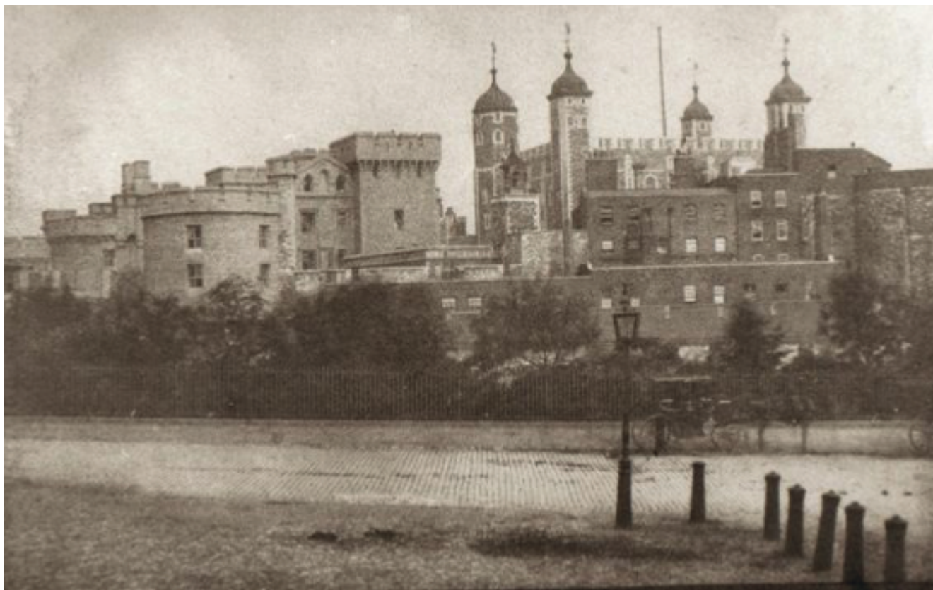
Fig. 1: the earliest known view of the Tower, taken by George Hilditch and displayed at the Society of Arts London Exhibition in 1852. Note the condition of the upper part of Flamstead's Tower on the north-east corner of the White Tower (left) before the introduction of the great clock the following year. The iron railings and the embryonic garden were laid out in 1828 under the instructions of the Duke of Wellington, and together with the medieval road in the foreground beyond were sadly swept away in 2005.
