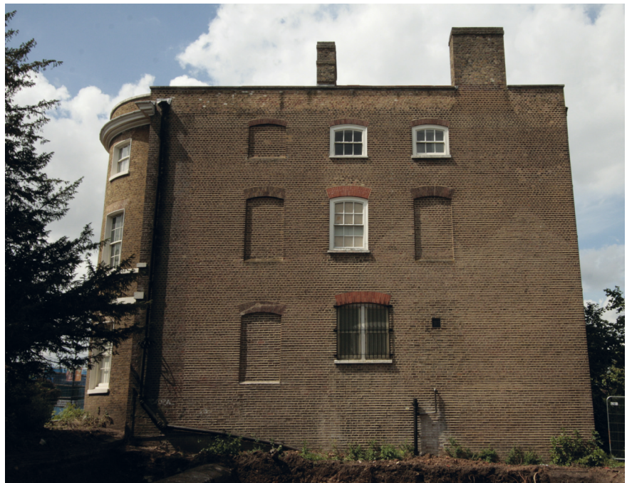
Fig. 9: East elevation of Water House and wall scars
