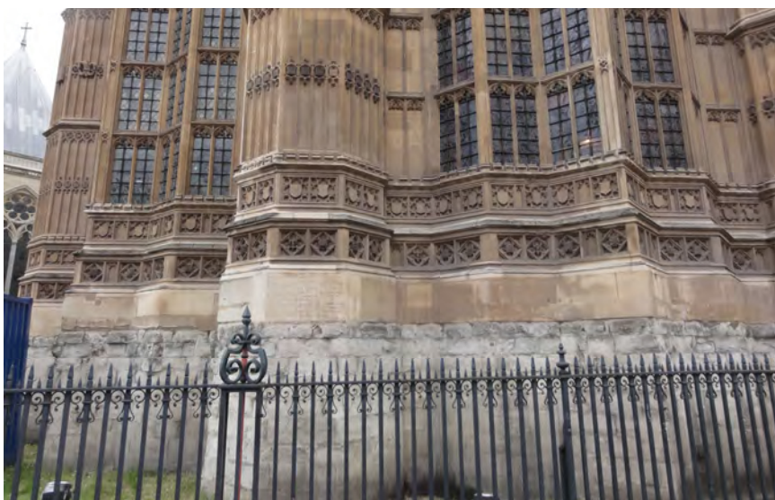
Fig. 7: plinth of the Henry VII Chapel, Westminster Abbey (left) with the detail of the ragstone masonry (right)
