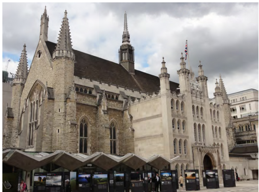
Fig. 5: the London Guildhall with Kentish ragstone to the left of the 18th-century porch
