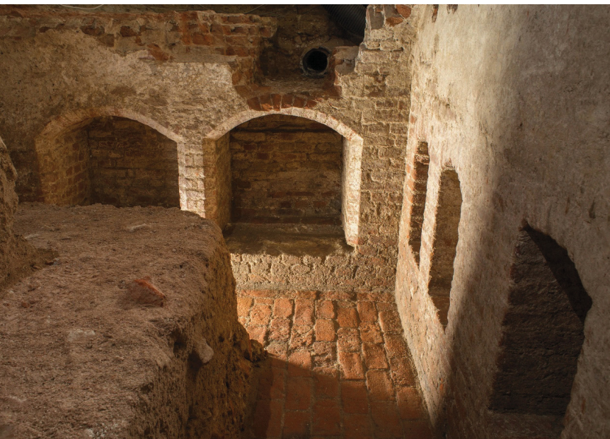
ABOVE view looking south with one of the Tudor cellars with larger bee boles to the south and smaller ones to the west Both photos © Pre-Construct Archaeology Limited
