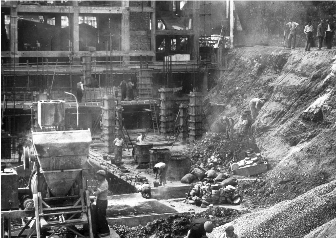
Fig 3: St Swithin's House, site photograph showing the building methods of 1949
