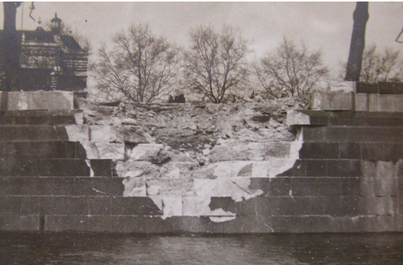
ABOVE: Serious damage to the Embankment in April 1941, next to the Victoria Tower, photographed by LCC's Thames Flood Prevention team (Peter Kennedy/LMA)
