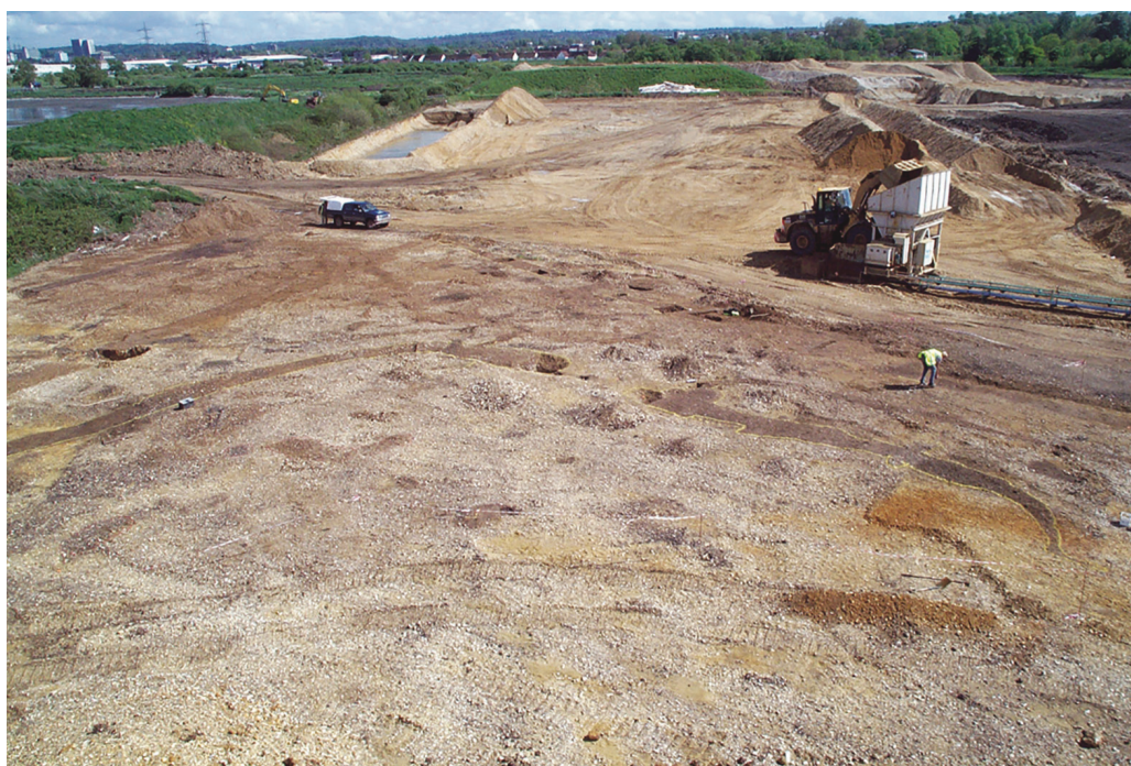
Fig 1: excavations in progress; south-east facing view across corner of a later Bronze Age enclosure (6101)
