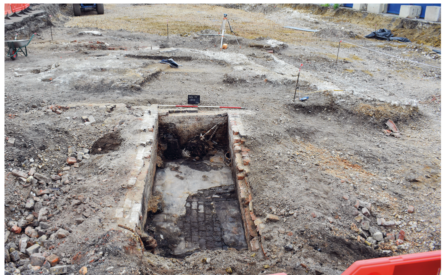
Fig 13: overview of the excavation showing the chalk yard surface in the background and Building D in the foreground
