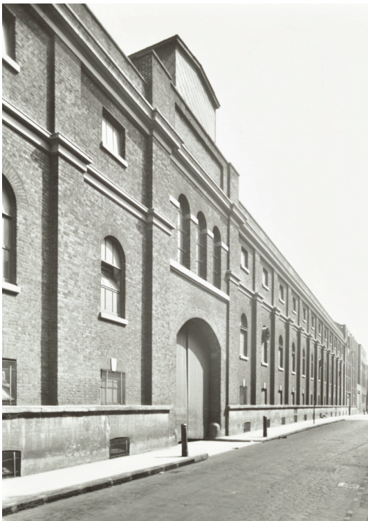
Fig 6: the mid-19th century Wilkes Street frontage of Truman Brewery's, view looking south; photo taken in 1955 (© London Metropolitan Archives, City of London)
