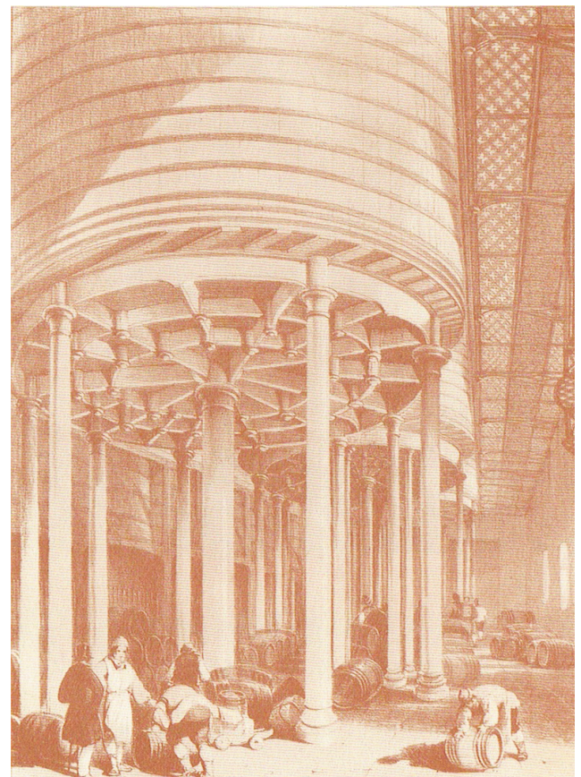
Fig 5: 1830s lithograph of large fermenting vats on the site of the Brick Lane brewery (© British Library Board: Document Supply Wq1/5735)
