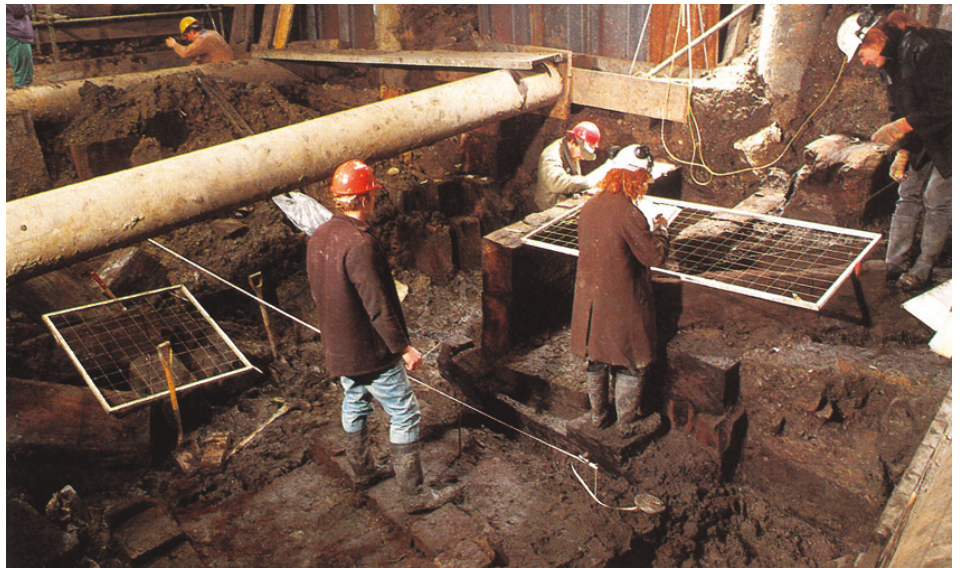
Fig 2: recording and dismantling the Roman waterfront timbers under Cannon Street viaduct (LYD88). The difficulties of excavating under the vaults were compounded due to problems with shoring, lighting and fumes (MOLA).
