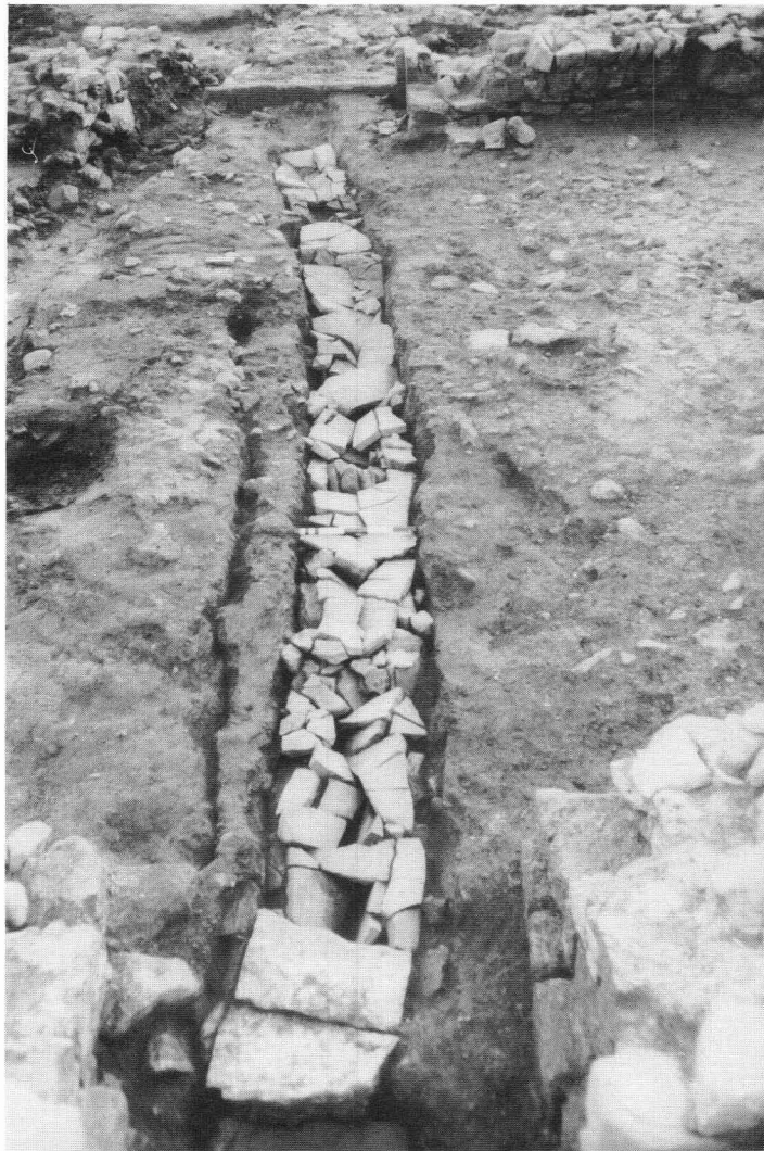
Plate 9 Site 11: the Period 3b drain, F52, from the north.
