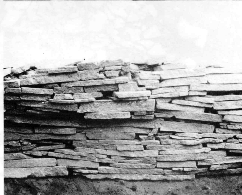
c. Outer revetment wall to the E of Chamber 3, looking S (p. 60). Height of wall \approx 0.6 m.
