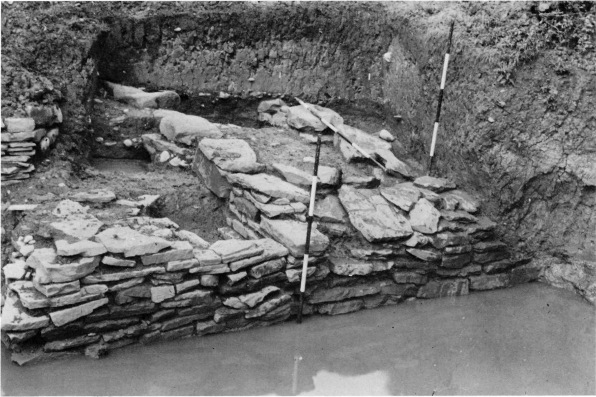
Plate IIIA. Junction of the primary and secondary quay-walls and the return of the primary quay.
