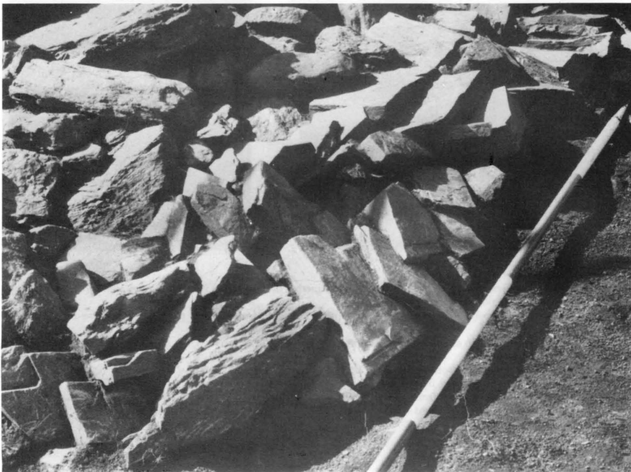
Detail of extra-revetment immediately in front of the retaining wall on the south side of the eastern forecourt.
