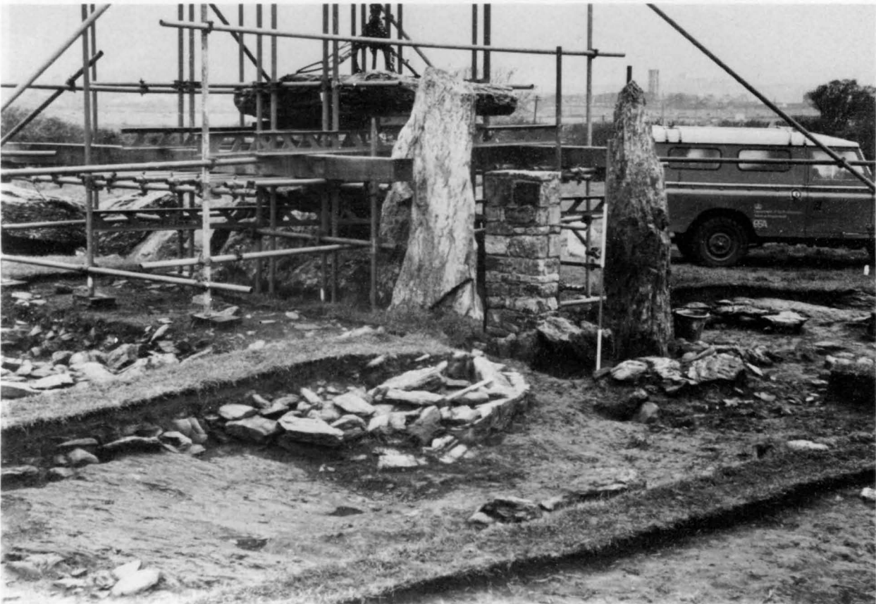
The eastern chamber in 1977, during excavation, looking north west.
