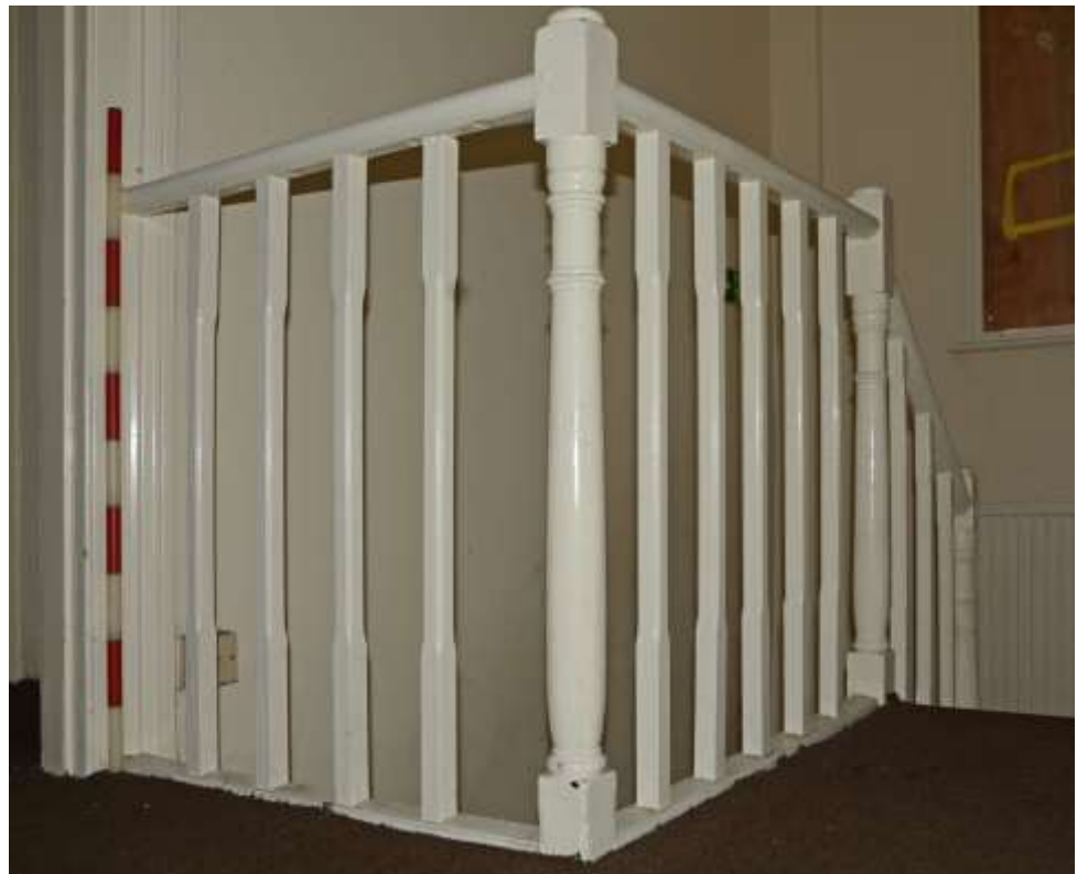
Fig.94: Detail of the balustrade and newel post
