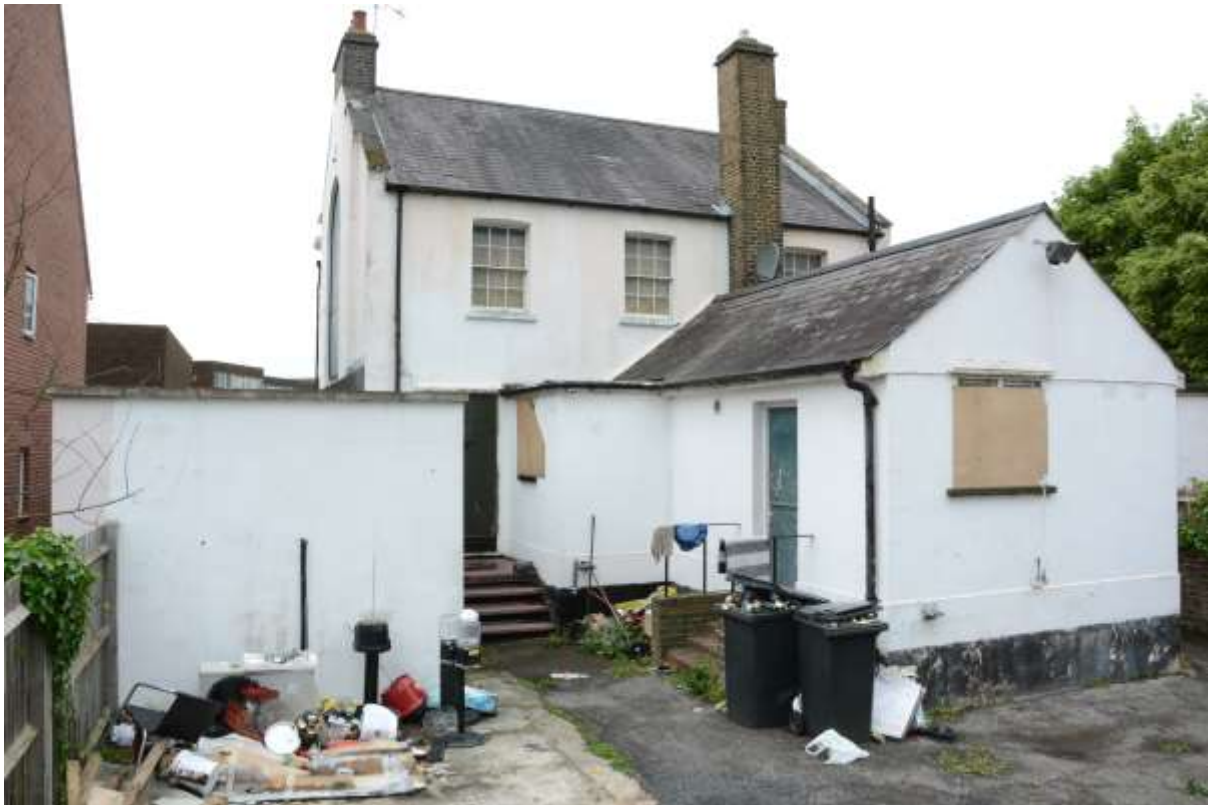
Fig.19: General rear view looking WSW. The two flat-roofed structures are clearly additions – that to the left modern and the smaller in the centre c 1920s. However, the main gable-roofed kitchen block may also have been rebuilt as the original outline is much shorter. It may also be significant that one end of the stone sill below the central first-floor window has been cut at 45° to accommodate the roof slope
