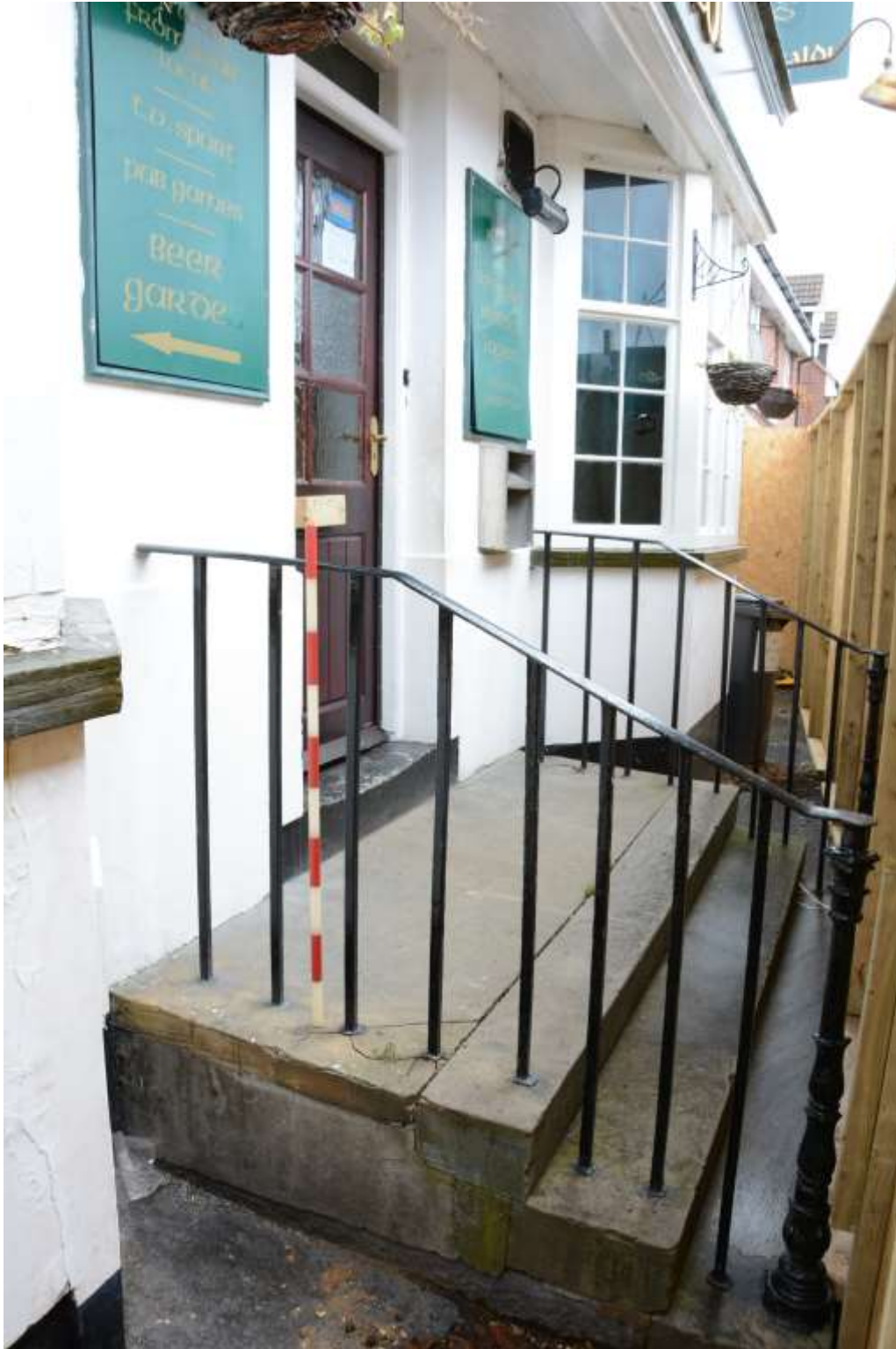
Fig.21: Front entrance steps and railings (1m scale)
