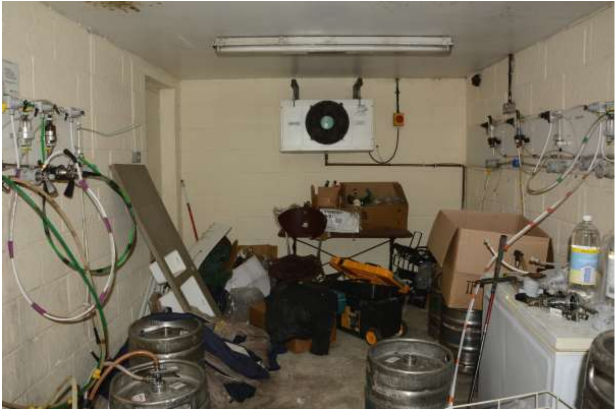
Fig.80: The modern single-storey storeroom at the southeast corner of the property, external door to the left (see Fig.36 for the outside view)
