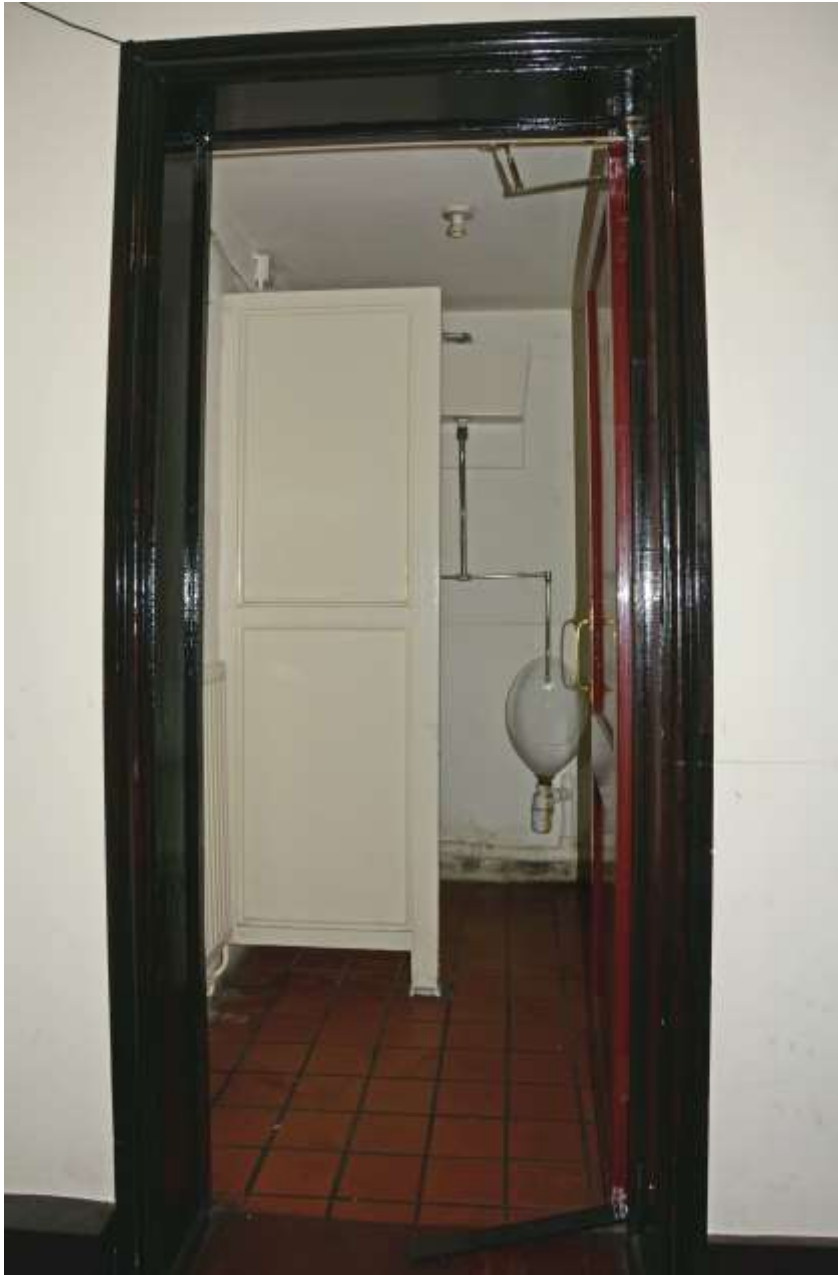
Fig.62: Toilet within the small single storey extension to the rear of the eastern room
