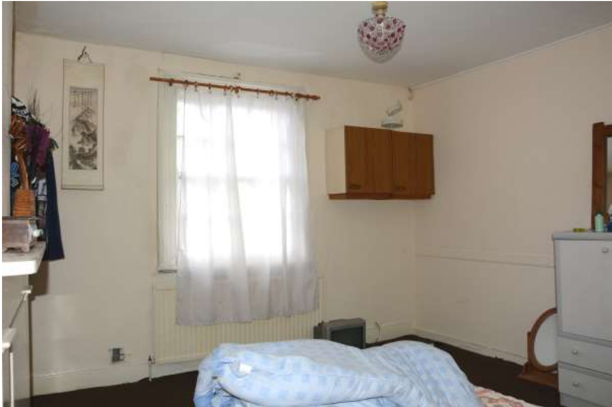
Fig.101: The sash window in the principal front bedroom (see Fig.39 for exterior)
