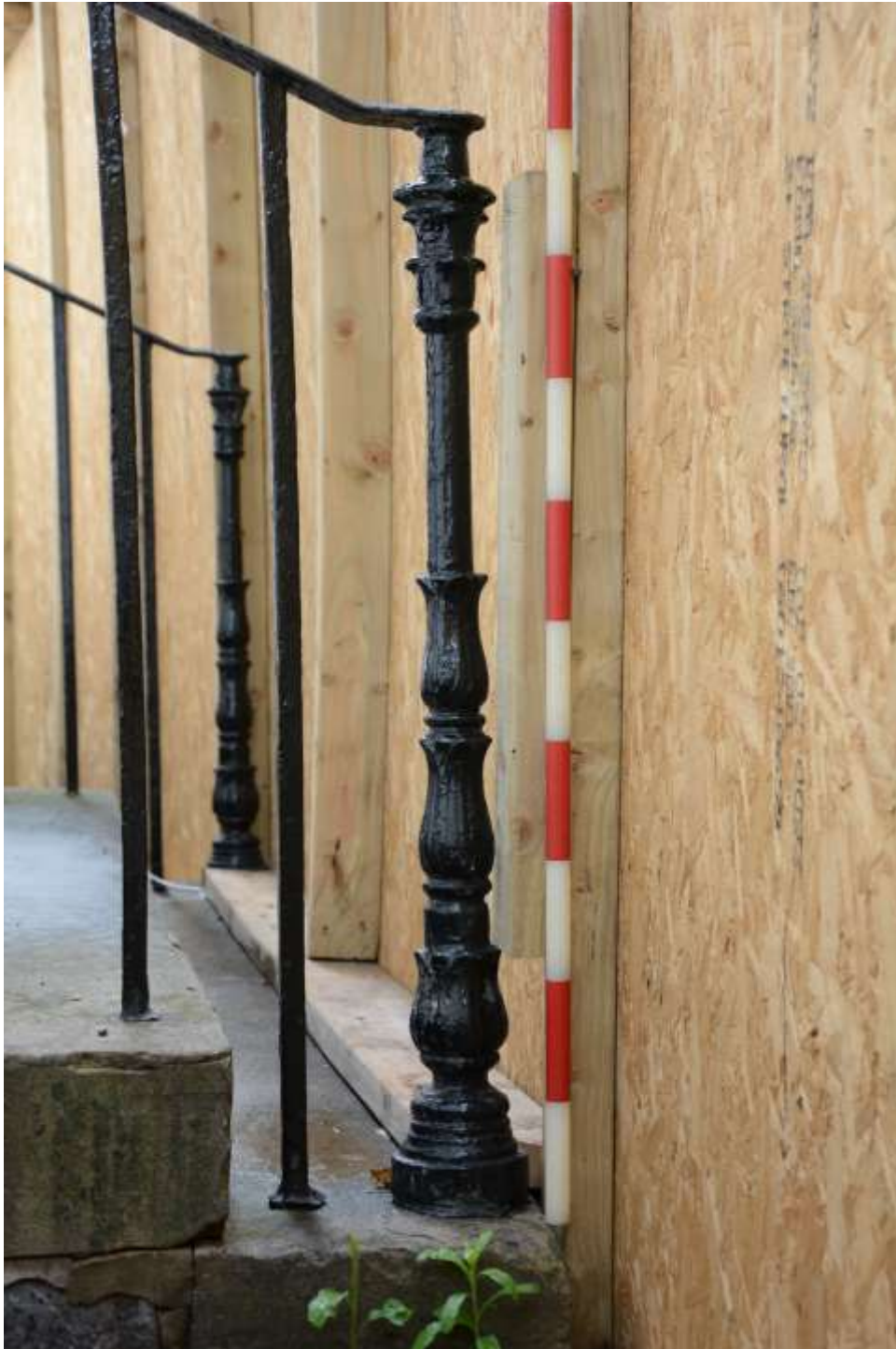
Fig.22: Close-up view of decorated cast iron post at the foot of the entrance steps (1m scale)
