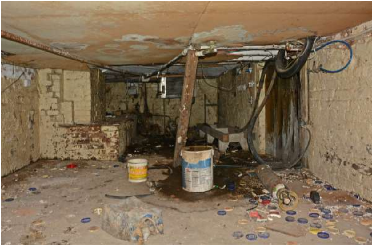
Fig.48: The main cellar, looking towards the rear of the building
