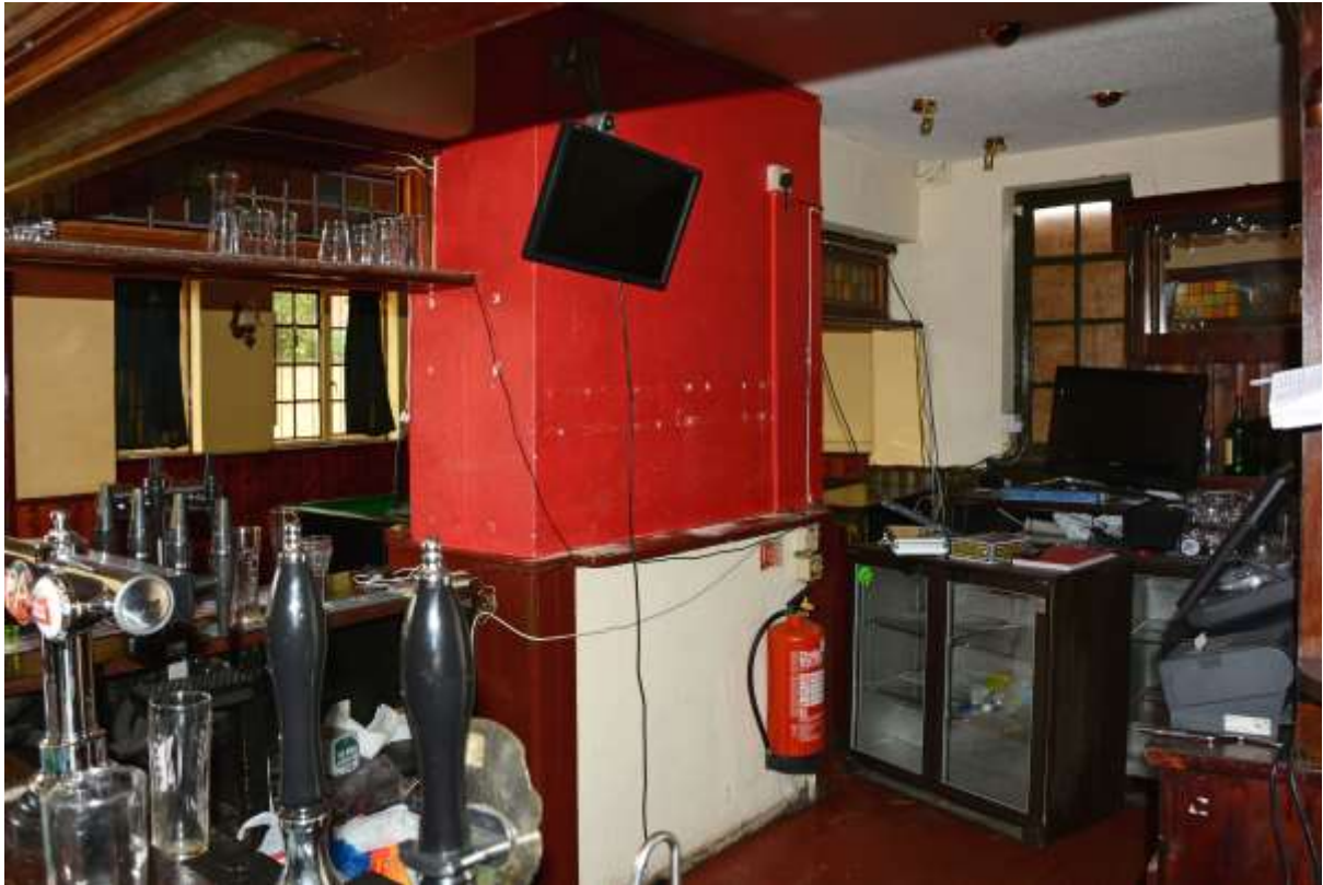
Fig.69: View from behind the bar, including (at centre) the original chimney breast and blocked fireplace opening
