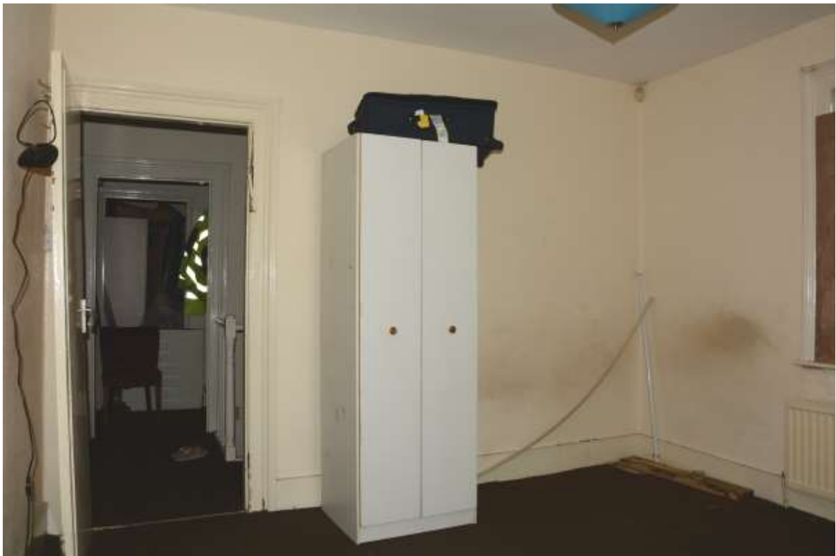
Fig.98: A further view of the bedroom, looking back onto the landing
