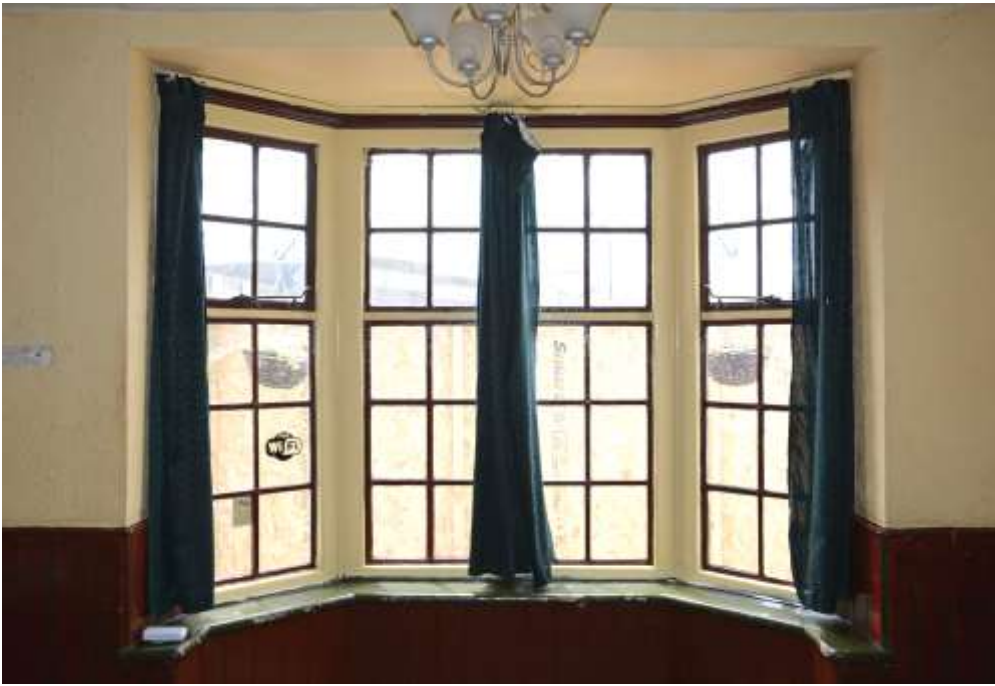
Fig.54: The interior of the northwestern bay window
