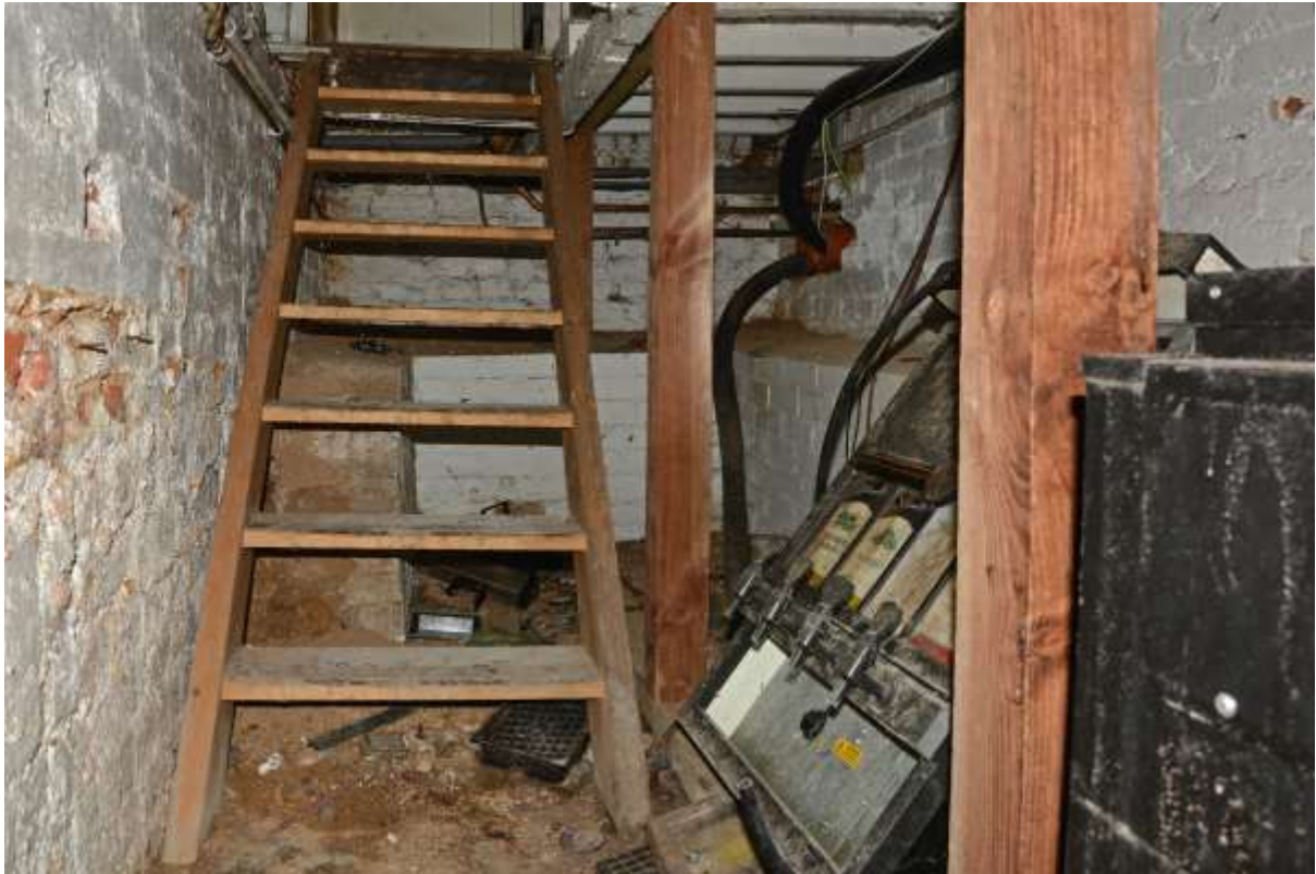
Fig.46: View of the cellar steps from below
