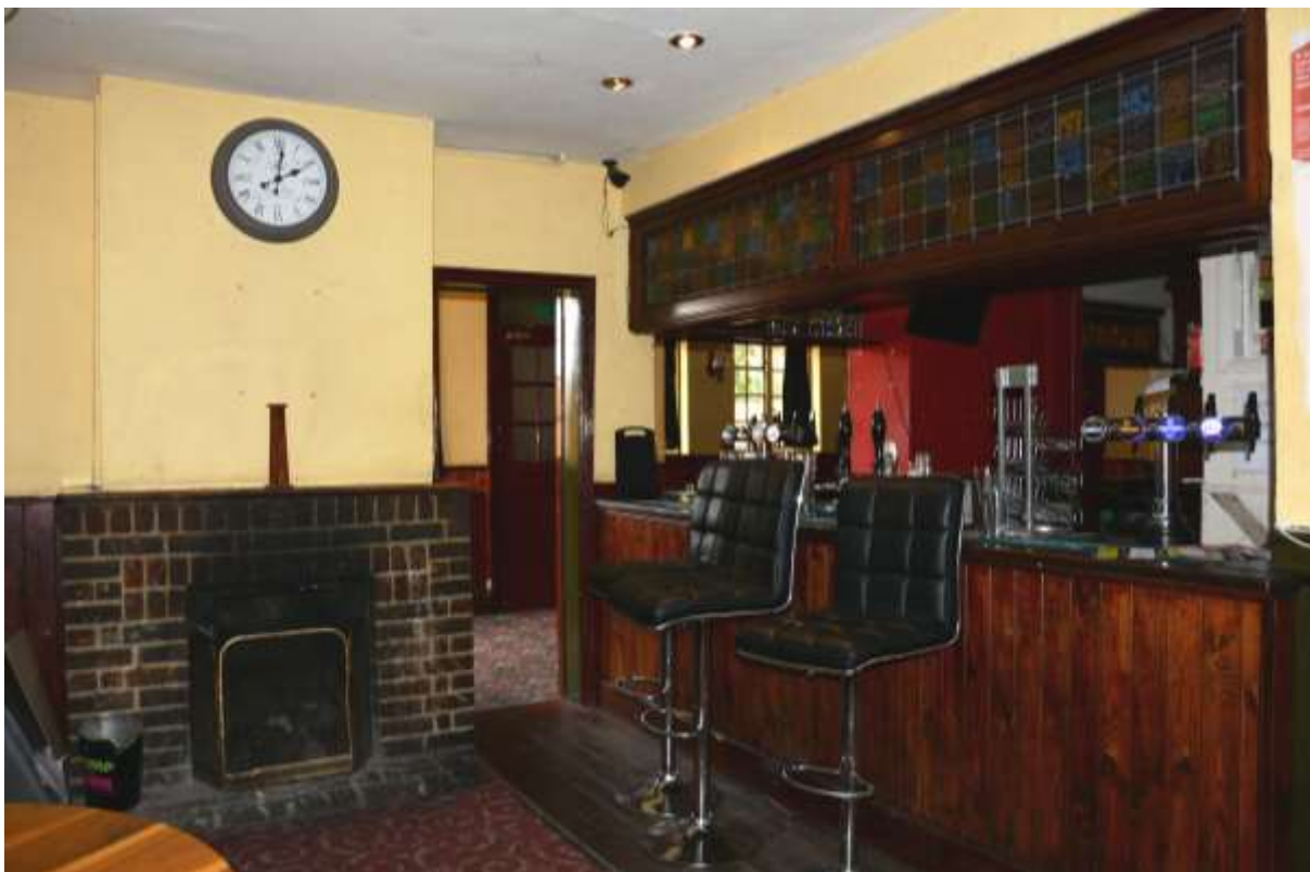
Fig.53: Closer view of the bar and adjacent 20 th century fireplace. Similarly to the previous picture, the plastered beam or girder above the bar is assumed to mark the original division of this area into two separate rooms
