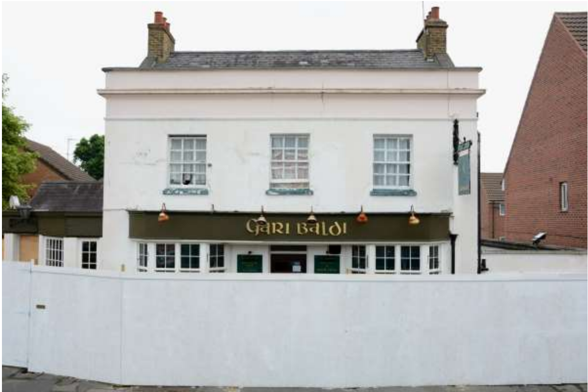
Fig.12: The building frontage, looking northeast
