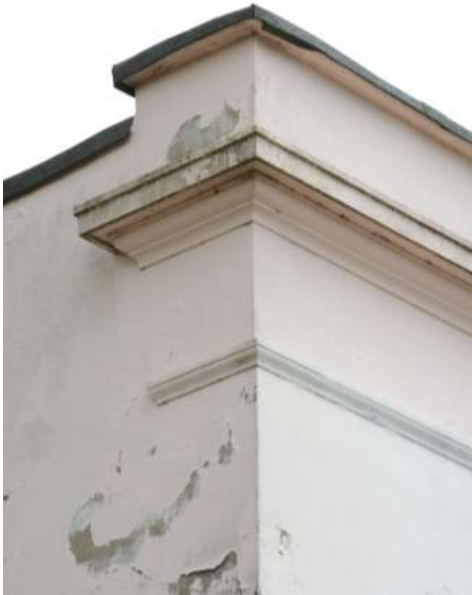
Fig.41: Detail of the northwestern end of the front parapet
