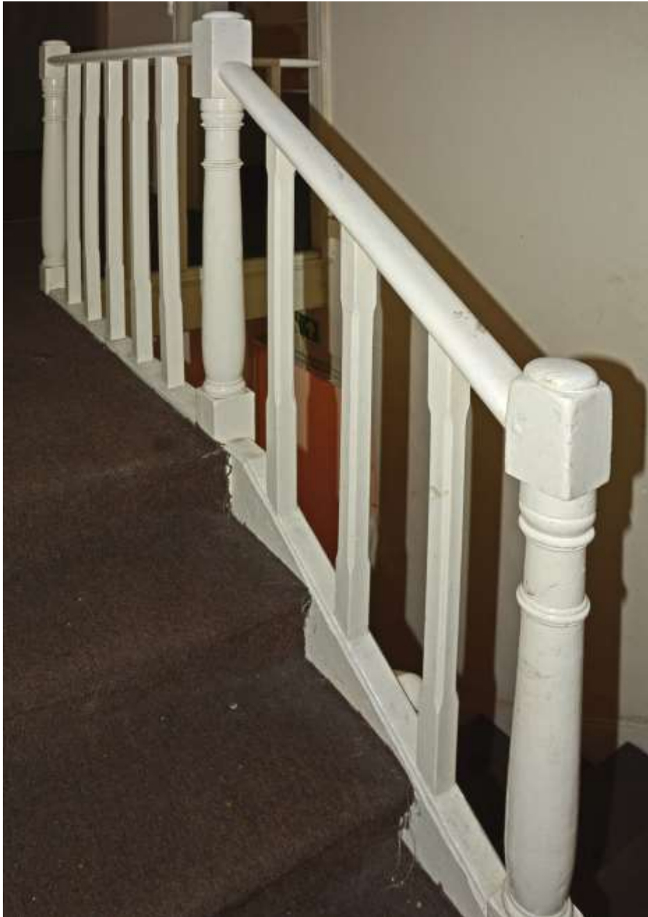
Fig.92: Detail of the upper staircase and balustrade
