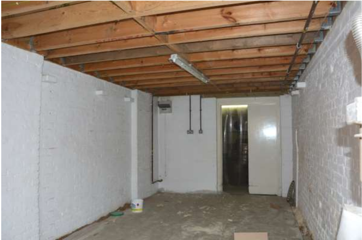
Fig.73: The single-storey garage to the southeast, with the main building (& projecting chimney breasts) to the left. The roof and end wall /doorway are modern but the outer wall (on right) is probably 19 th century, and both side walls retain stone corbels for an earlier roof
