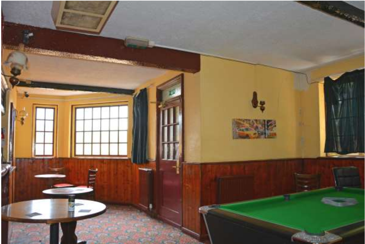
Fig.65: The northwestern area, view towards the door to the entrance lobby. The large beam at top left may represent the division between two phases of earlier 20 th century extension
