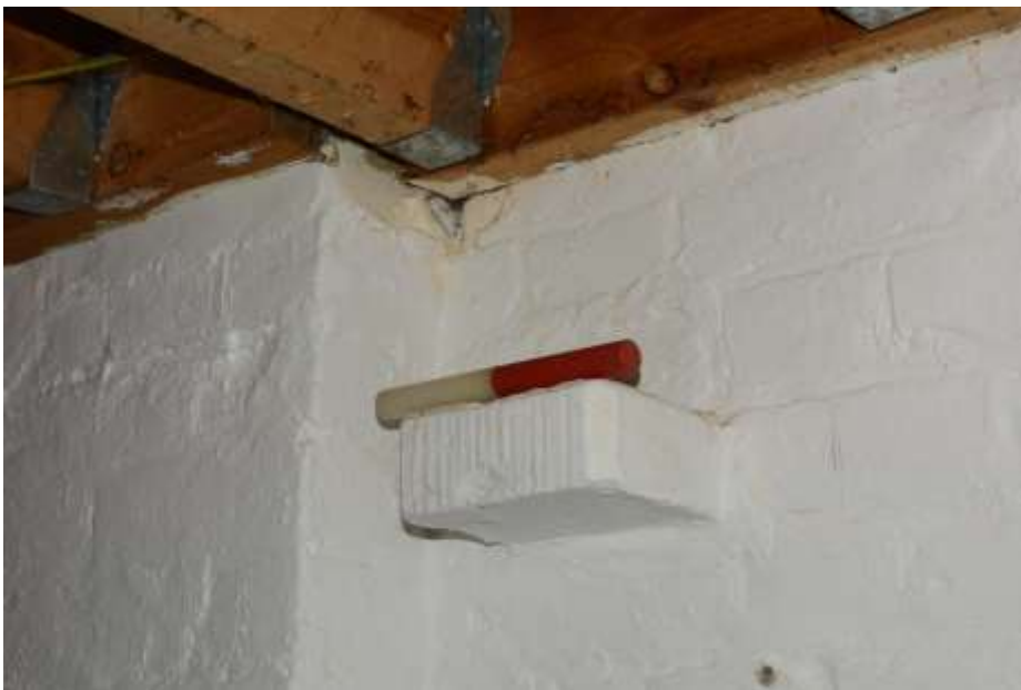
Fig.77: Close-up view of stone corbel on the main wall, adjacent to the SW chimney stack (0.2 m scale)
