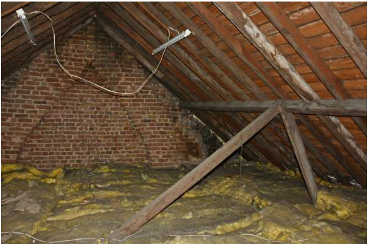
Fig.112: A similar view to the above, orientated SSE
