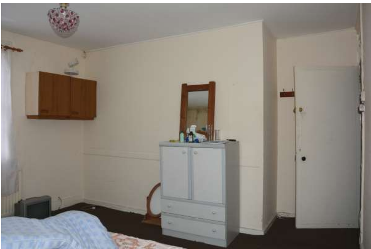
Fig.102: The later NE wall of the principal front bedroom: note the apparently quite modern skirting – plain & much smaller – and also the beading at the top of the wall
