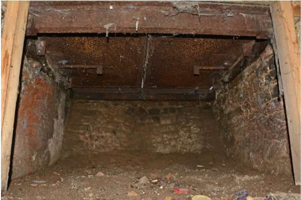
Fig.50: Detail of the external access hatch at the front of the building. The two metal doors with retaining latches can be seen, joining in the centre of the picture
