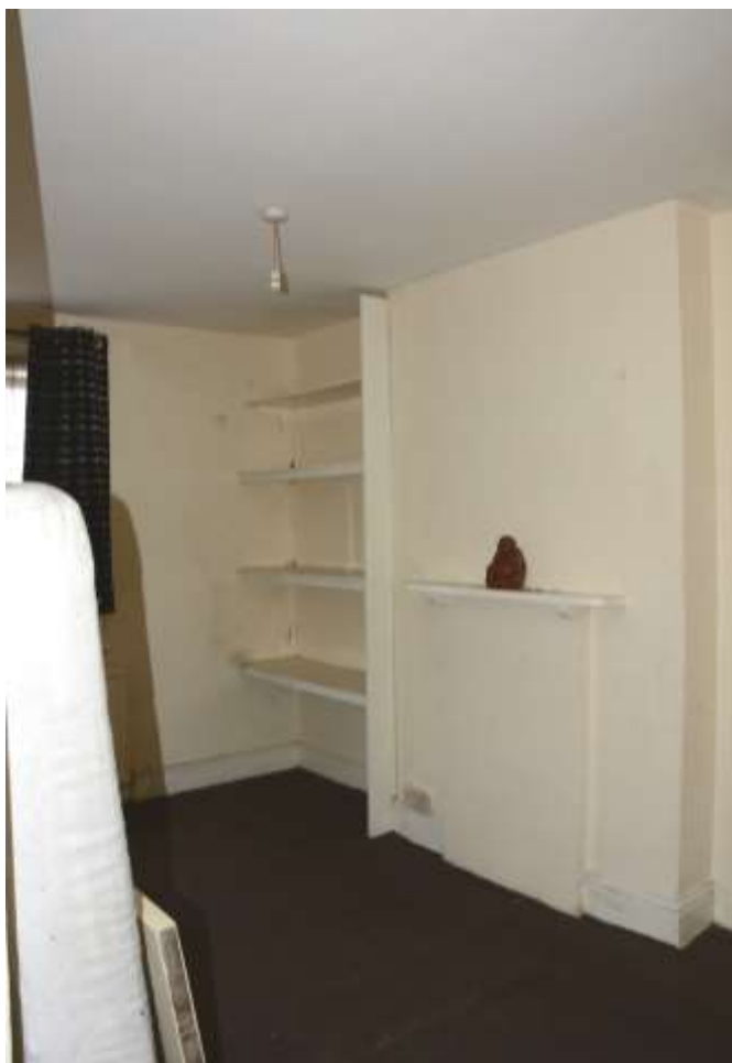
Fig.105: The northwestern bedroom. The moulded skirting on three walls matches that in the other main room, but the fire surround is much closer to that in the rear bedroom and embellished only by simple brackets supporting the shelf
