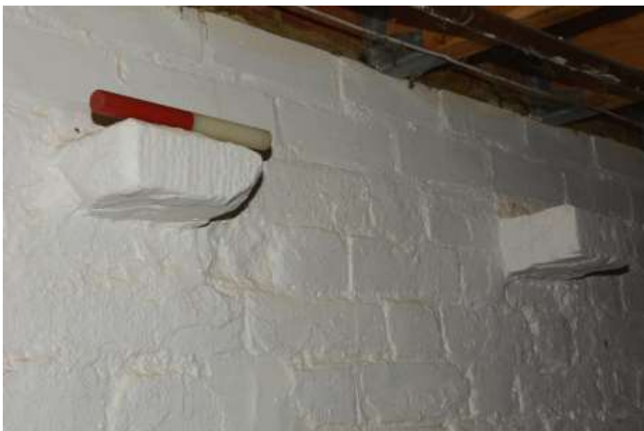
Fig.79: Two of the corbels on the outer wall (a third being located at the SW end). The upper two brick courses are modern
