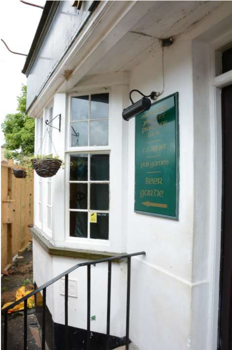
Fig.23: The northwestern bay window and overlying canopy. Although within the original building it is possible that both these features were added in the earlier 20 th century (cf. Fig.32, etc.)
