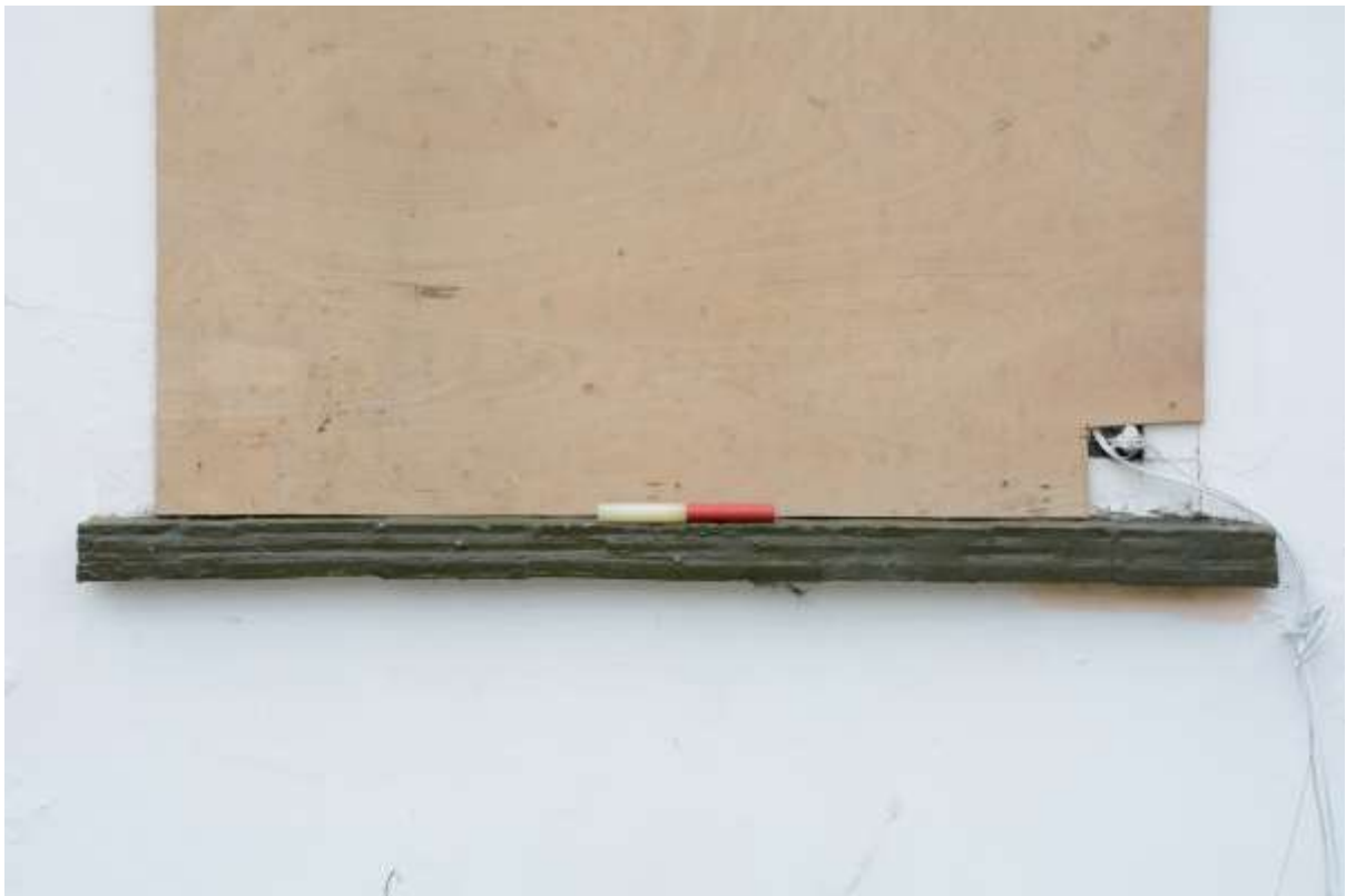
Fig.35: The same sill construction at the projecting centre/rear of the building
