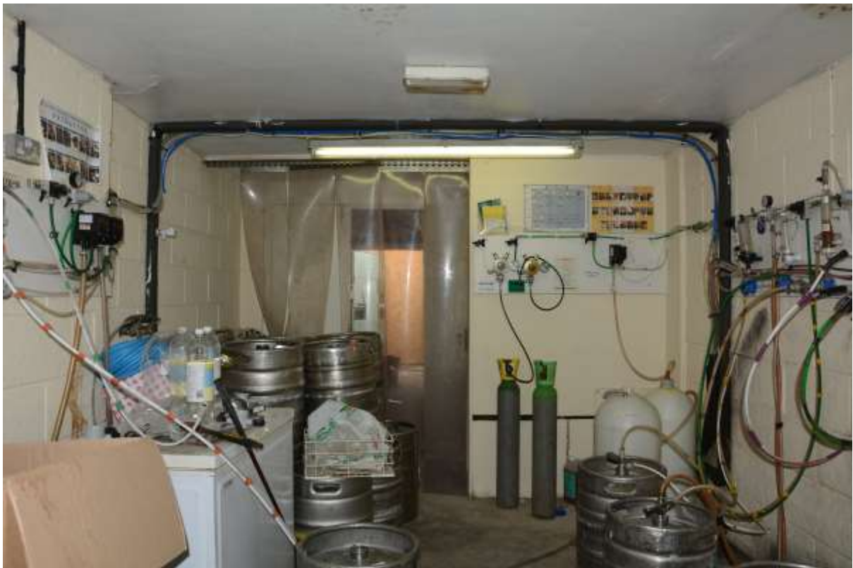
Fig.81: The single-storey storeroom, looking back to the SW towards the garage
