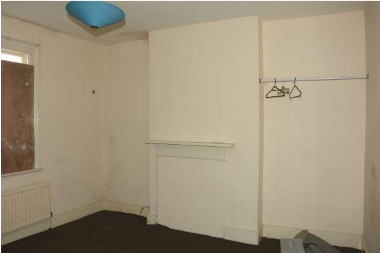
Fig.97: The rear (SE) bedroom, showing the chimney breast, the blocked and very basic fire surround, and adjacent plain skirting board
