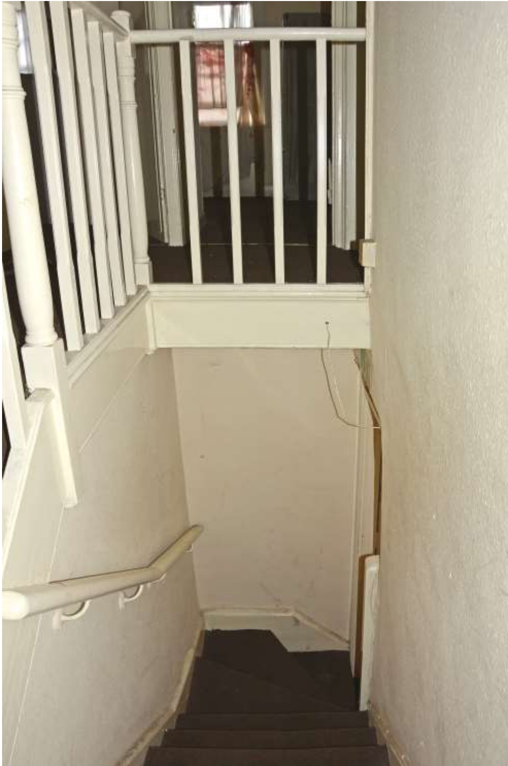
Fig.91: View looking down the lower flight of stairs (compare with Fig.89). There is nothing to suggest that the staircase and balustrade are not original features of the building, although it may be that they were originally approached more directly than the passageway (Fig.88) that now exists
