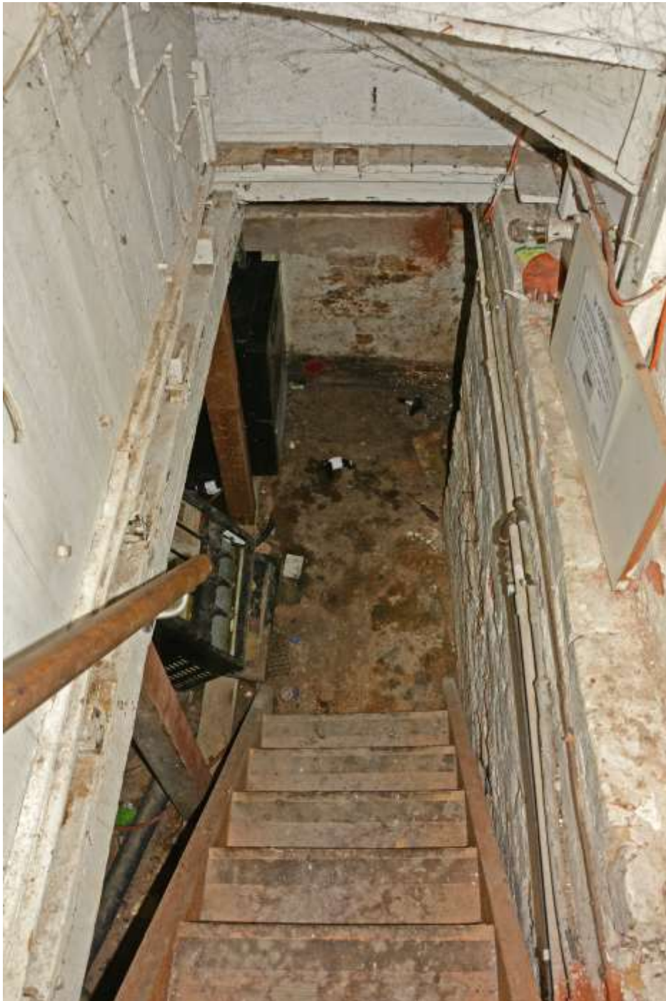
Fig.45: Wooden steps giving access to the cellar
