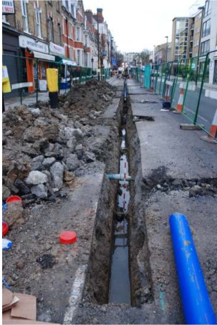
Figure 26 Monitored open-cut trench on Blackstock Road (Trench 1 – 13/01/11) looking south (1m scale).
