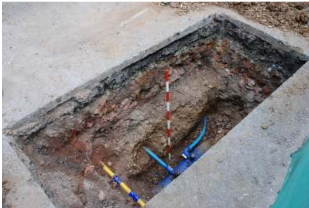
Figure 42: Pit at the south end of Wyatt Road showing clean gravel towards the base of excavations.
