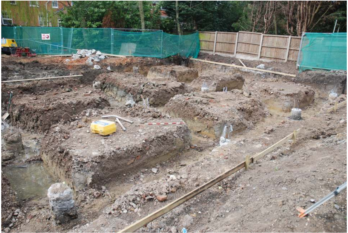
Fig 8 Oblique view of the excavations looking approximately west.
