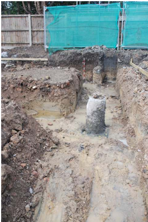
Figure 9 General view of the northernmost strip of the footprint looking NW and showing the scale standing against the higher surviving section (Fig 10-11).
