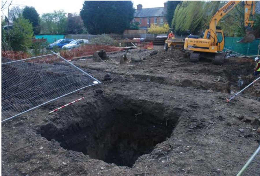
Figure 12: General view of the test pit looking approx. south (1m scale)
