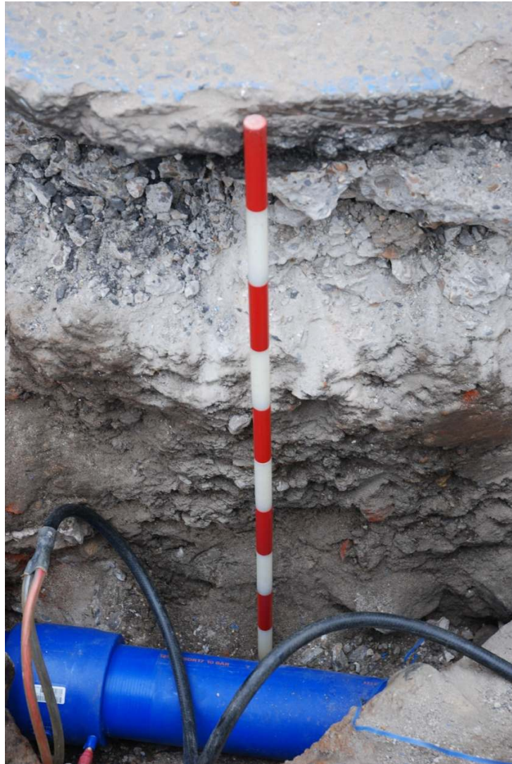
Figure 23: North facing section of trenching on President Street (1m scale).
