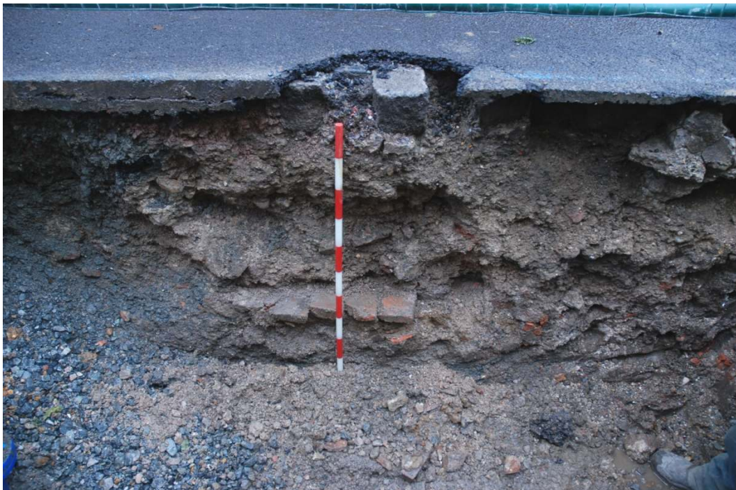
Figure 8: Single course of 19 th century brick-work exposed in trenching immediately north of Coombs Street (1m scale).
