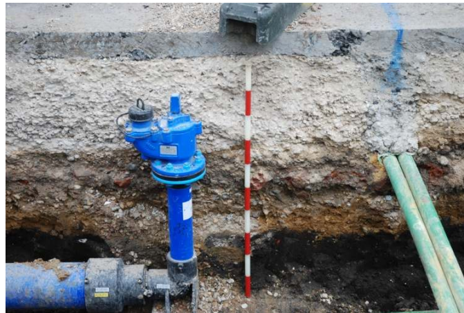
Figure 14: West facing section of trenching on Macclesfield Road showing modern road layers overlying 19 th century buried soil.
