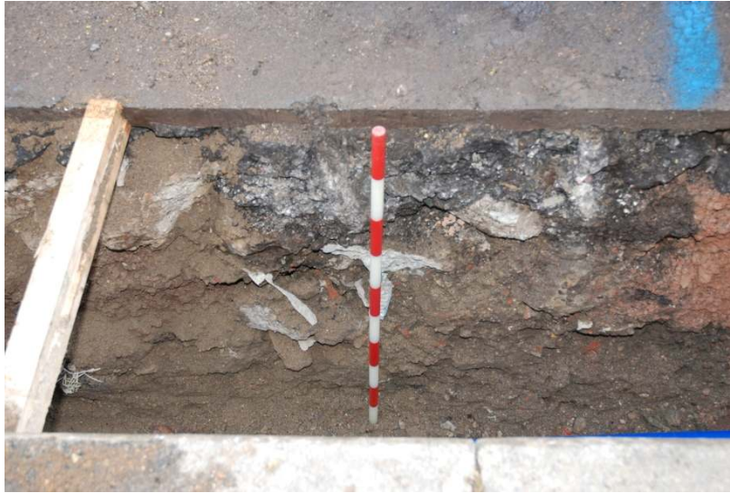
Figure 16: South facing section of trenching on Moreland Street showing modern road layers over made-ground (1m scale).
