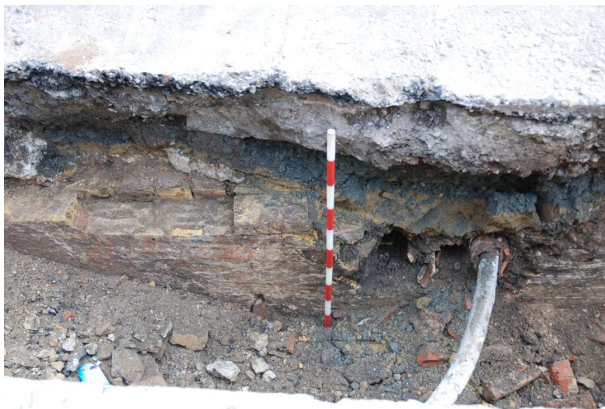
Figure 5: Cellar wall in the west facing section of trenching on Central Street , cut by a modern service and backfill (1m scale).
