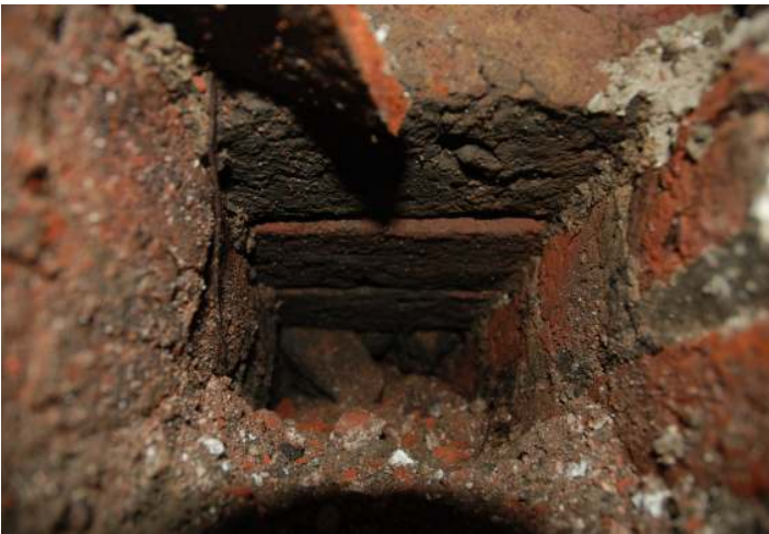
Fig. 36: Photo of interior of drain in trial pit 10B.
