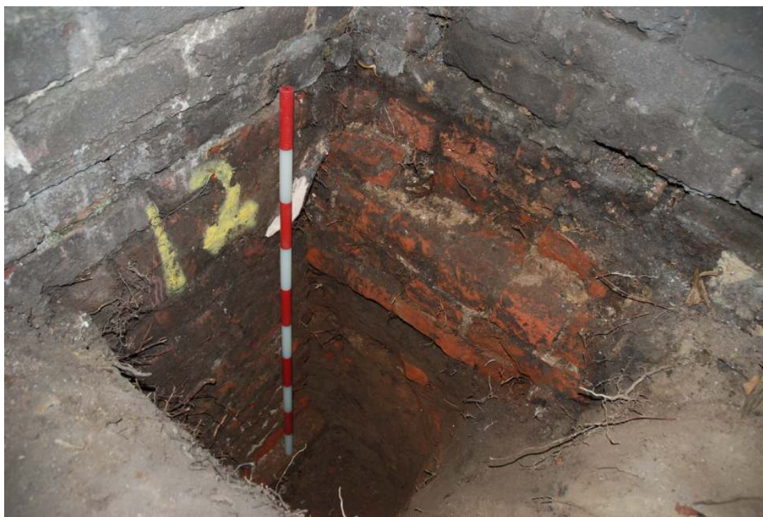
Fig. 42: Photo of trial pit 12, clearly showing the foundations of both the garden wall (left of the scale) and boundary wall (right of the scale)
