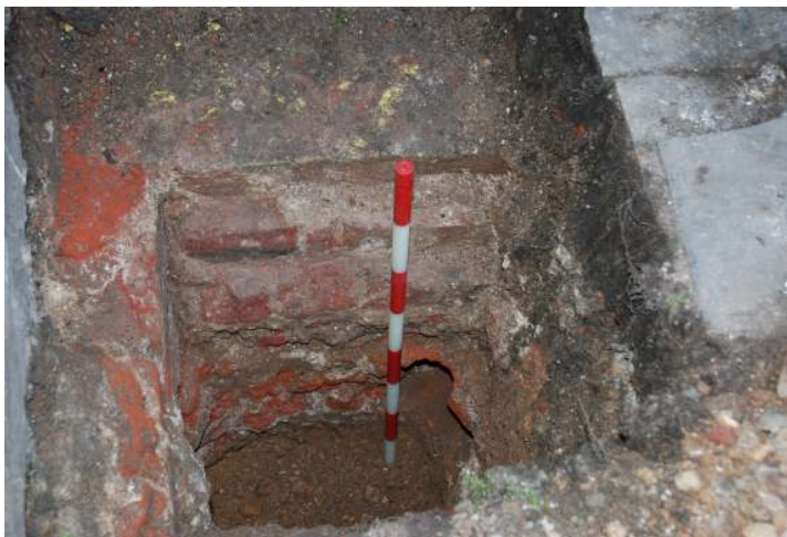
Fig. 37: Photo of trial pit 10B, from the south-east, clearly showing the drain gully in the north-west corner of the pit, and the brick wall in the western section.
