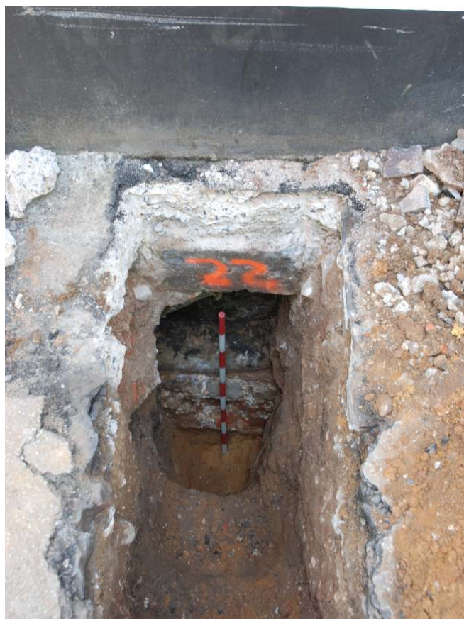
Fig. 63: Photo of western section in trial pit 22.
