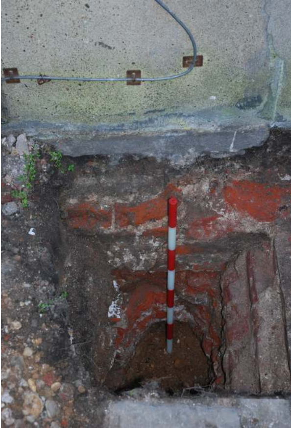
Fig. 34: Photo of brick walls in the southern and western sections of trial pit 10B.
