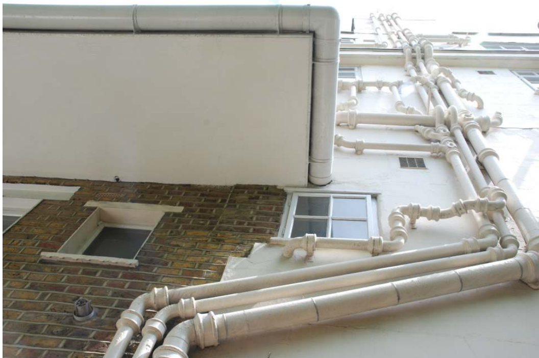
Fig. 4: Photo of the side of No.95 Cheyne Walk, directly above trial pit 1. In the centre of the photo, directly to the left of the window in the white part of the building, is a line in the brickwork which may represent the original back end of No.95 Cheyne Walk, discussed in relation to the wall base in trial pit 1.
