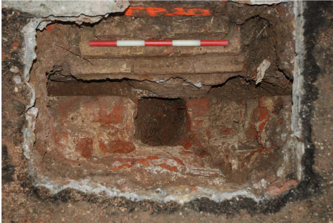
Fig. 61: Photo of trial pit 20, clearly showing the east-west running wall.
