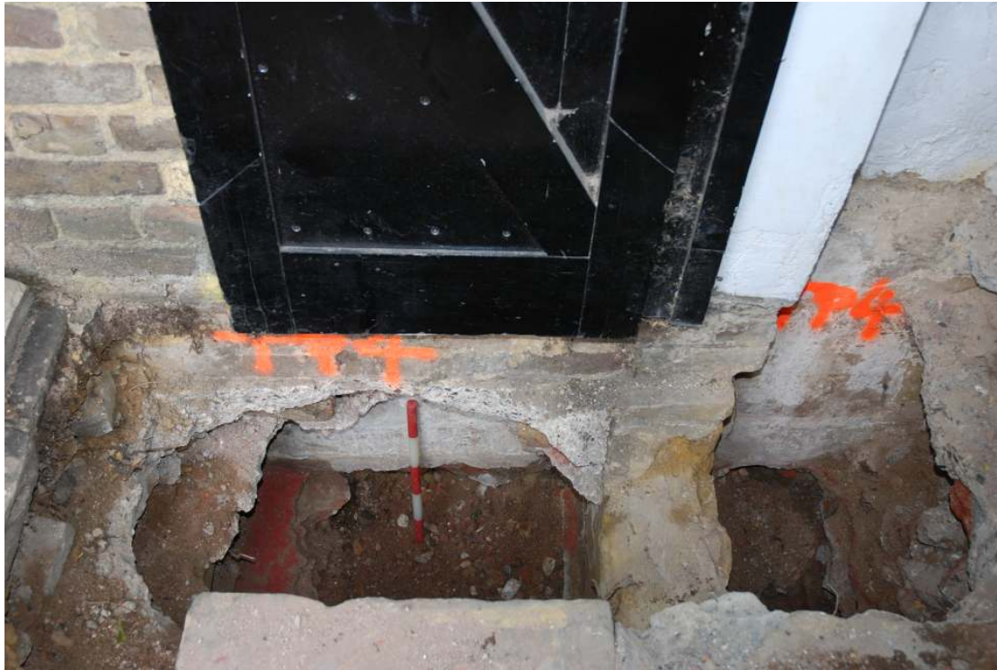
Fig. 14: Photo of trial pit 4, from above.
