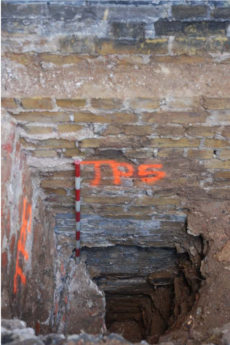
Fig. 17: Photo of trial pit 5, clearly showing the yellow stock brick wall foundations in the northern section.
