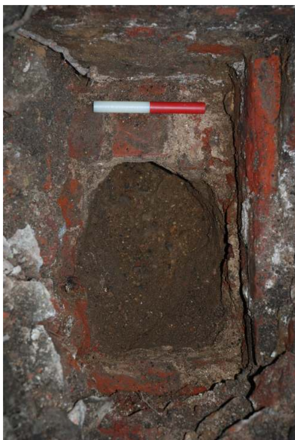
Fig. 28: Photo of brick plinth / floor in trial pit 10A, a deeper hole cut through the centre to expose the underlying natural deposit.
