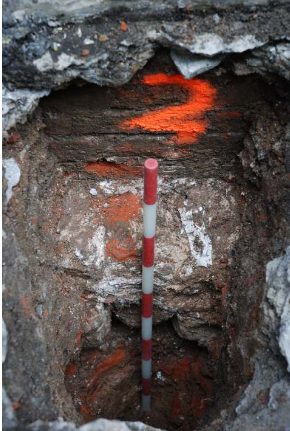
Fig. 8: Photo of the eastern section of trial pit 2, clearly showing the mid 19 th century wall foundations of No.95 Cheyne Walk
