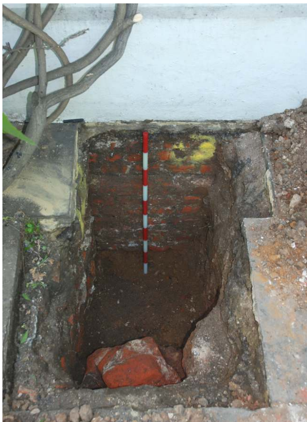
Fig. 44: Photo of brick foundations in trial pit 13 (taken from the south), with the earlier section of brickwork also visible in the foreground.
