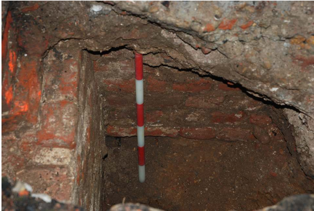
Fig. 24: Photo of brick wall in the southern section of trial pit 8.
