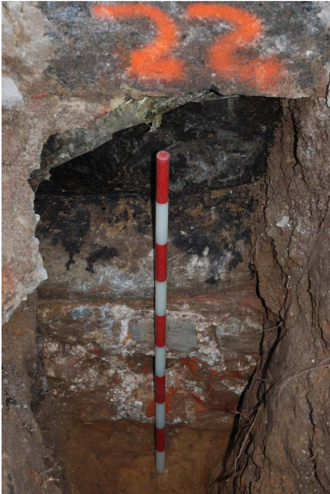
Fig. 64: Photo of the earlier wall base (behind the lower 0.6m of the scale) in the western section in trial pit 22.
