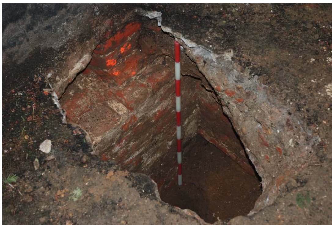
Fig. 21: Photo of wall in eastern section of trial pit 8.
