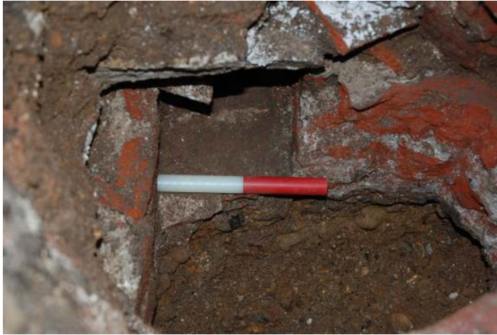
Fig. 35: Photo of drain gully in trial pit 10B.
