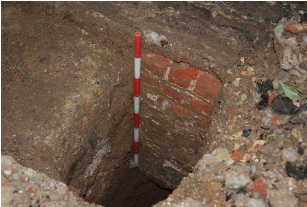
Fig. 9: Photo of wall foundations in the eastern section of trial pit 3.
