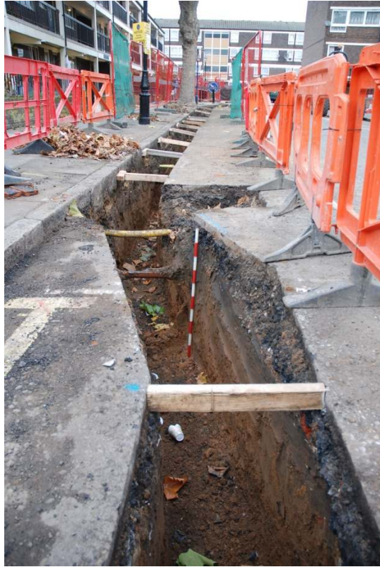
Figure 22: Trenching on Stafford Road looking towards the junction with Shetland Road.
