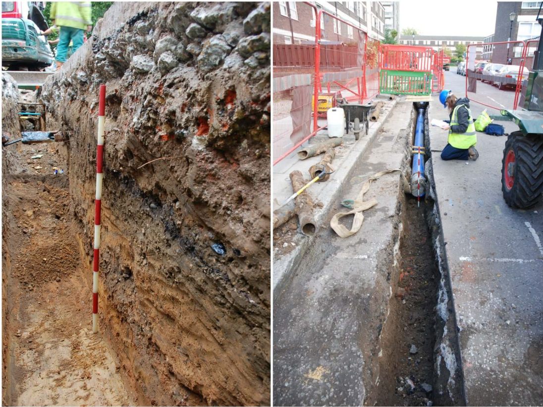
Figure 23: Section and general view of trenching on Saxon Road.
