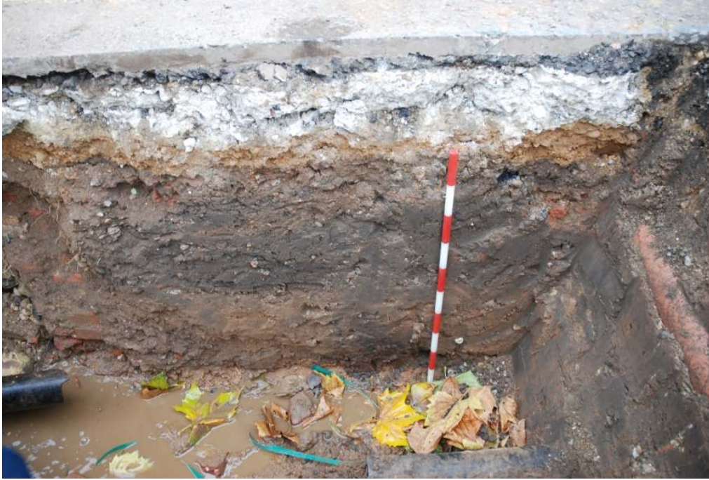
Figure 20: Trenching on Shetland Road.
