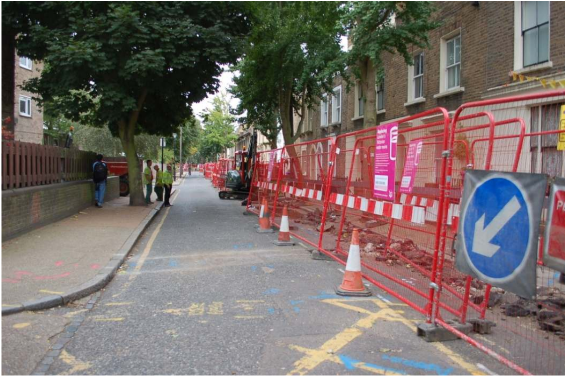
Figure 24: General view of trenching on Norman Grove, looking south.
