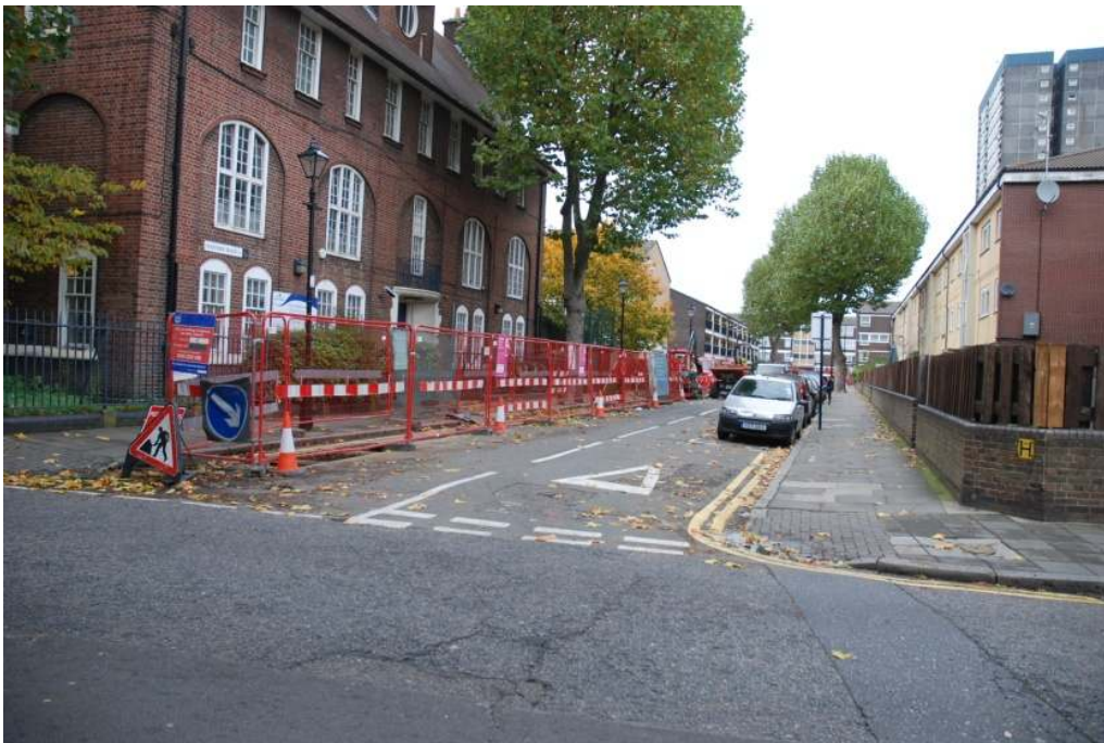
Figure 21: Groundworks on Stafford Road from the junction with Tredegar Road.
