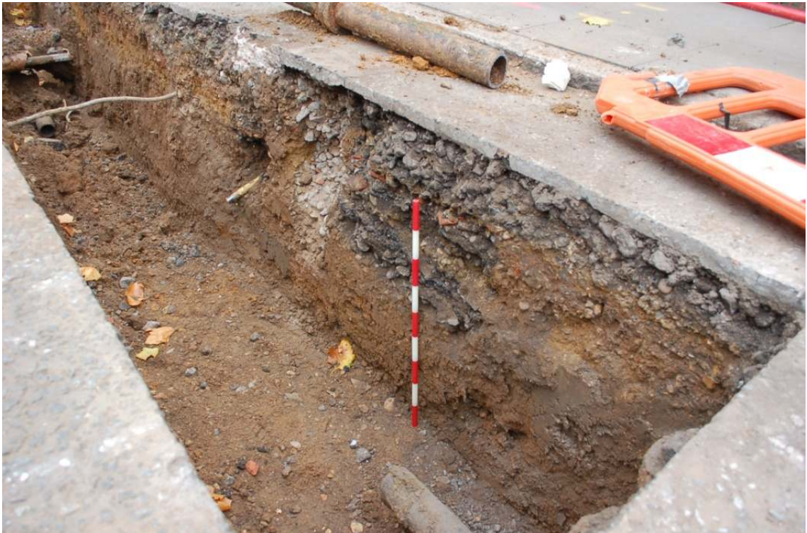
Figure 25: Section of trenching on Norman Grove.
