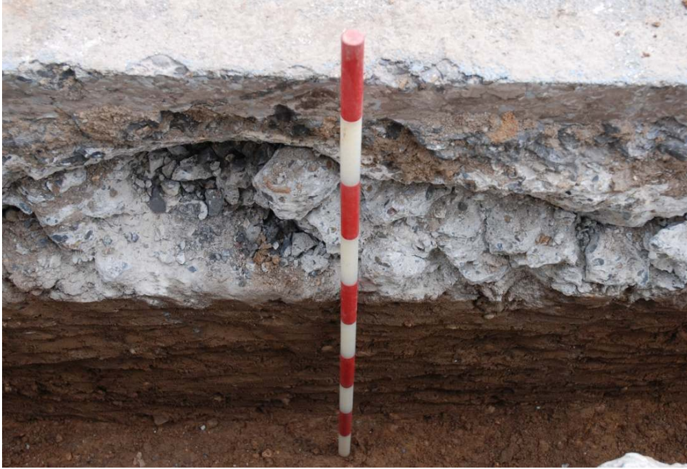
Figure 10: Section of trenching on Roman Road showing subsoil deposit [8] (see Figures 9 and 11 for general views).
