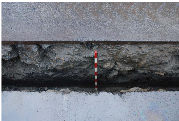
Figure 19: Section of trenching on Limehouse Causeway.
