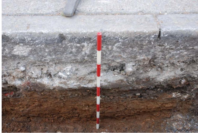
Figure 15: Section of trenching on Rich Street.
