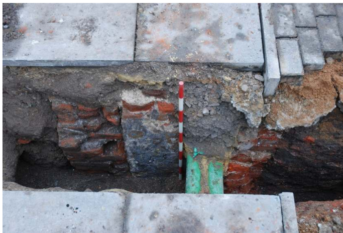
Figure 10: Truncated 19 th century cellar wall in trenching on Gill Street.
