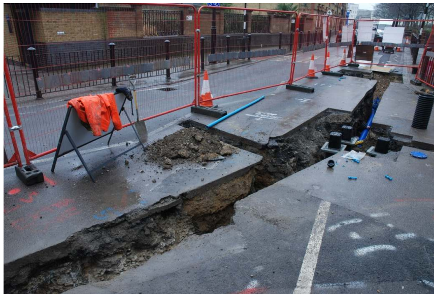
Figure 16: Trenching on Limehouse Causeway at the junction with Gill Street.
