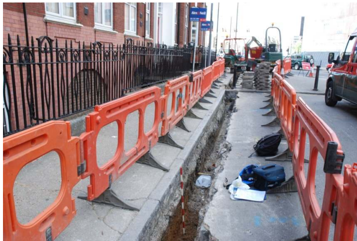
Figure 14: General view of trenching on Rich Street.
