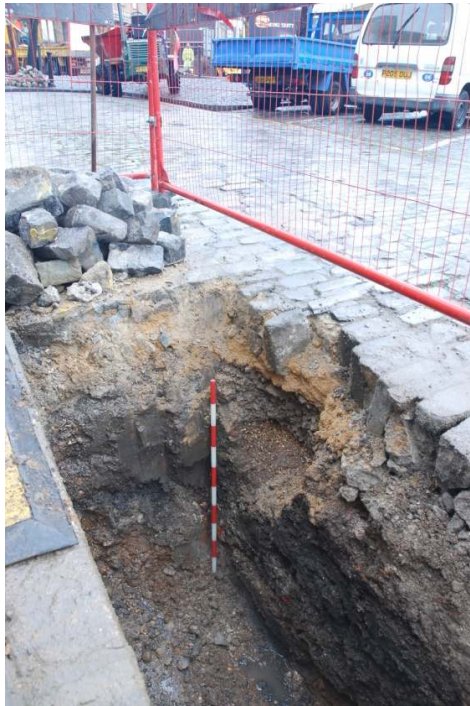
Figure 13: Launch pit on Salter Street.
