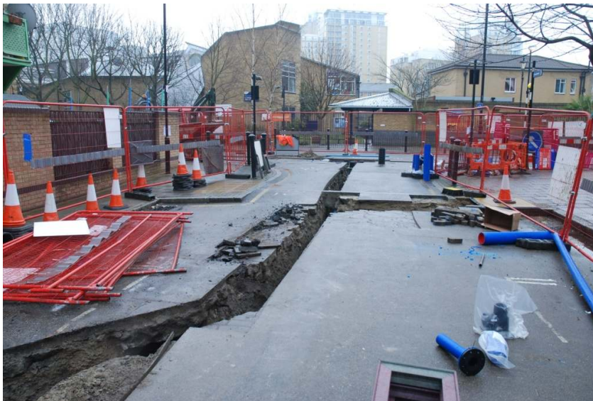
Figure 12: Trenching at the south end of Gill Street.
