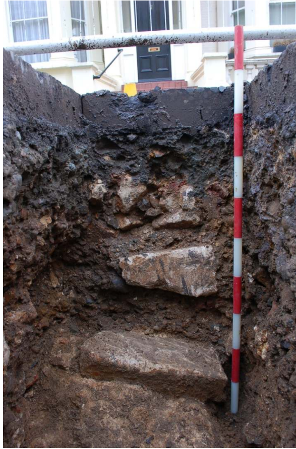
Figure 11 In-situ worked stones in 19 th century made-ground in Section 2, trenching on Penywern Road.
