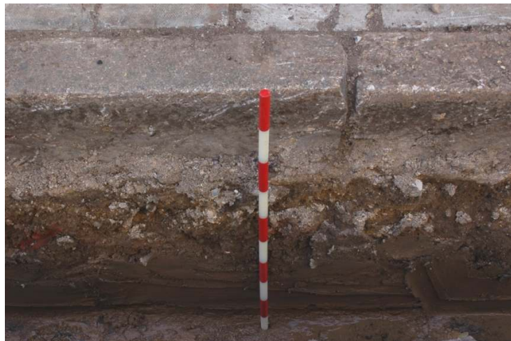
Figure 7: Section of trenching on Hillsleigh Road (1m scale).
