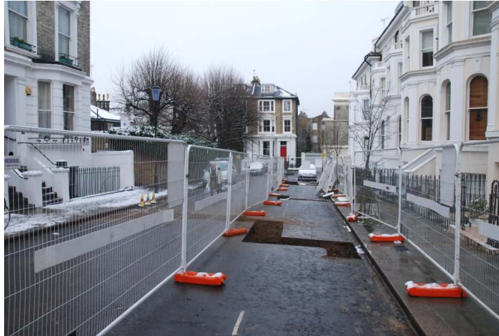
Figure 10: General view of trenching on Campden Hill Gardens, looking north.
