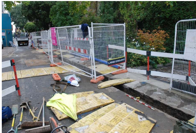
Figure 24: General view of trenching on Aubrey Walk looking east (1m scale).
