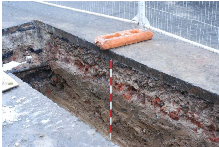
Figure 11: Section of trenching at the south end of Campden Hill Gardens (1m scale).
