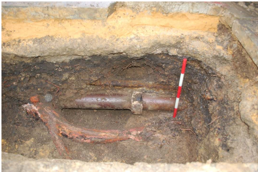
Figure 17: Section of trenching at the east end of Duchess of Bedford's Walk (0.5m scale).
