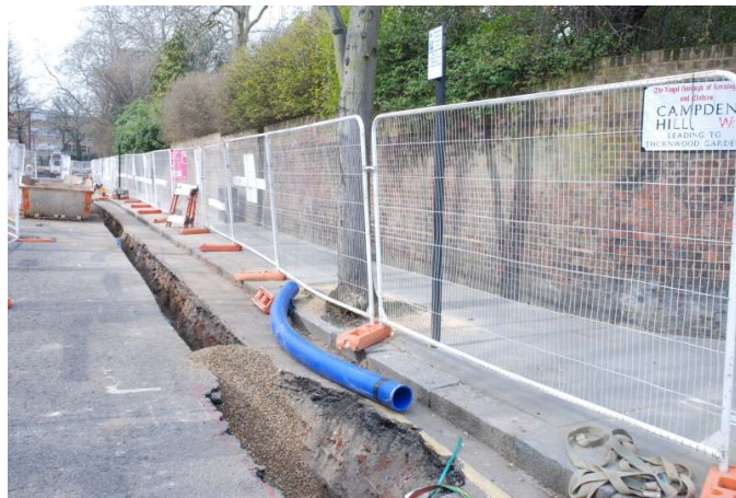
Figure 22: General view of trenching at east end of Campden Hill.
