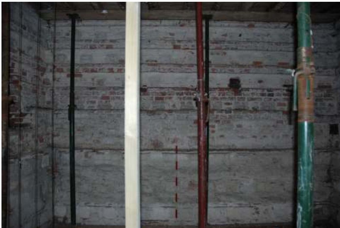
Fig. 27: Photograph of the interior eastern wall – first floor. Original build up to c.50mm above the top of the scale, after which the blocked nesting holes are distinctly different.
