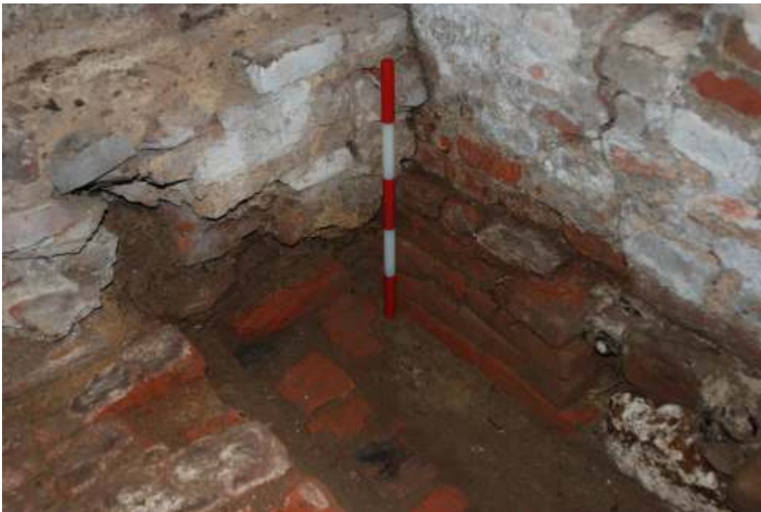
Fig. 40: Photograph of the small area of brick foundations observed in the western wall, looking south-west. This is possibly evidence for an earlier door in this wall.
