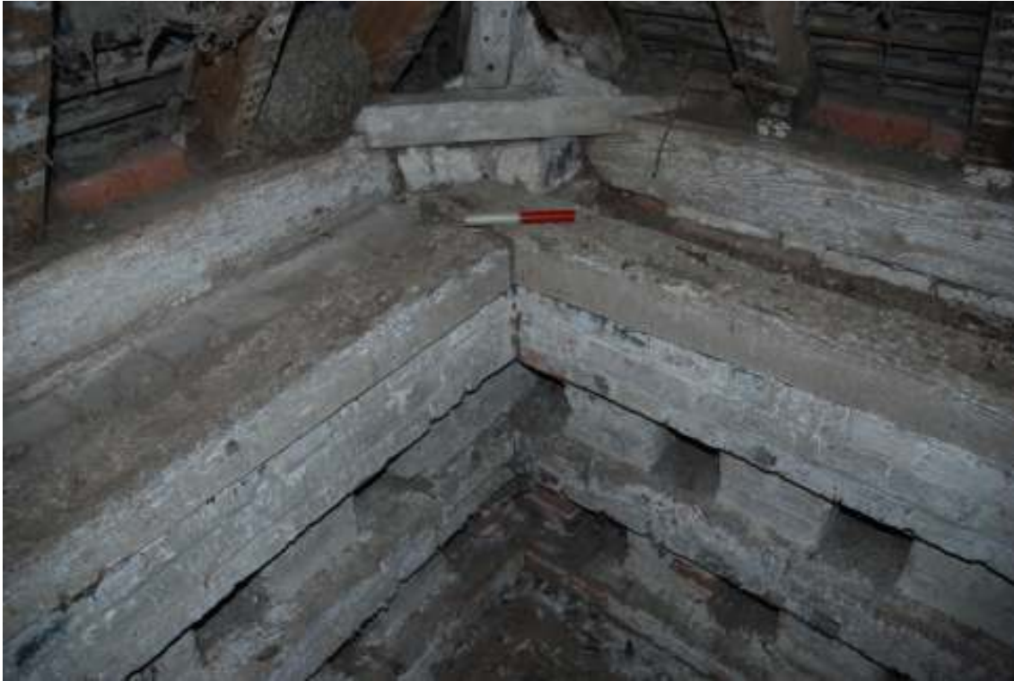
Fig. 79: Photograph of the earlier timber in the foreground along the top of the dovecote wall (south-east corner).
