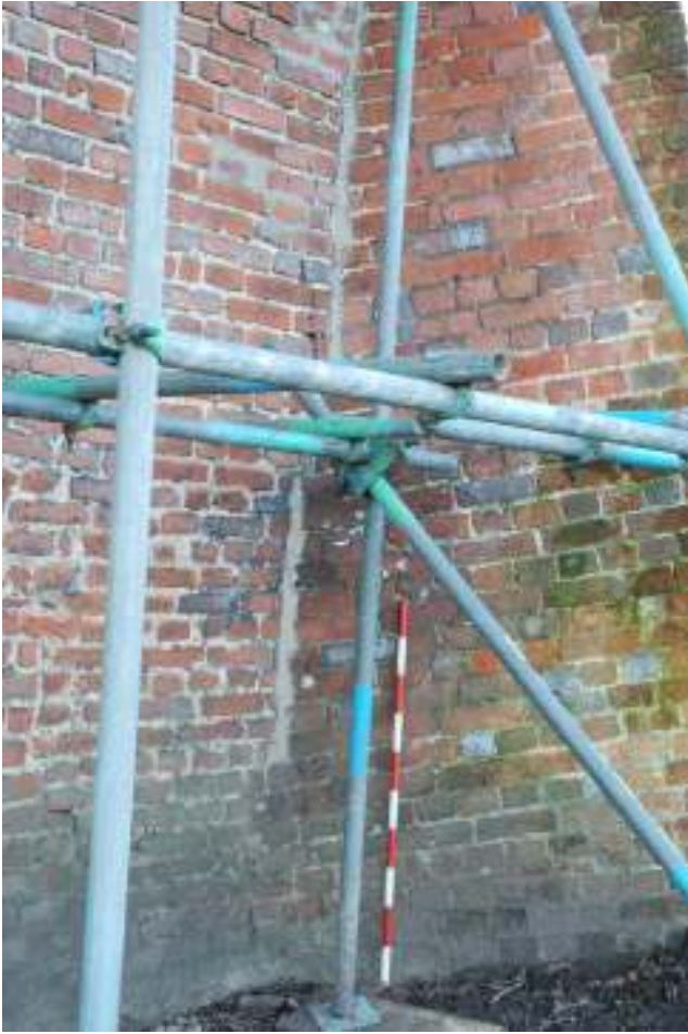
Fig. 93: Photograph of part of the southern side of the north-eastern buttress. This clearly shows the buttress abutting the main dovecote wall, and the grey mortar attaching this.
