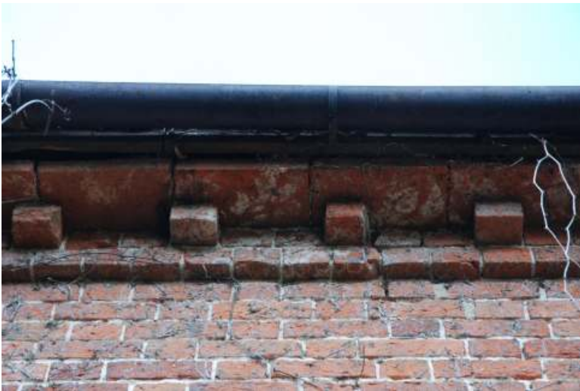
Fig. 82: Photograph of the exterior top of the dovecote at Eastcote. This shows the outwards-projecting bricks and flat tiles, and no way for doves to enter under the eaves.
