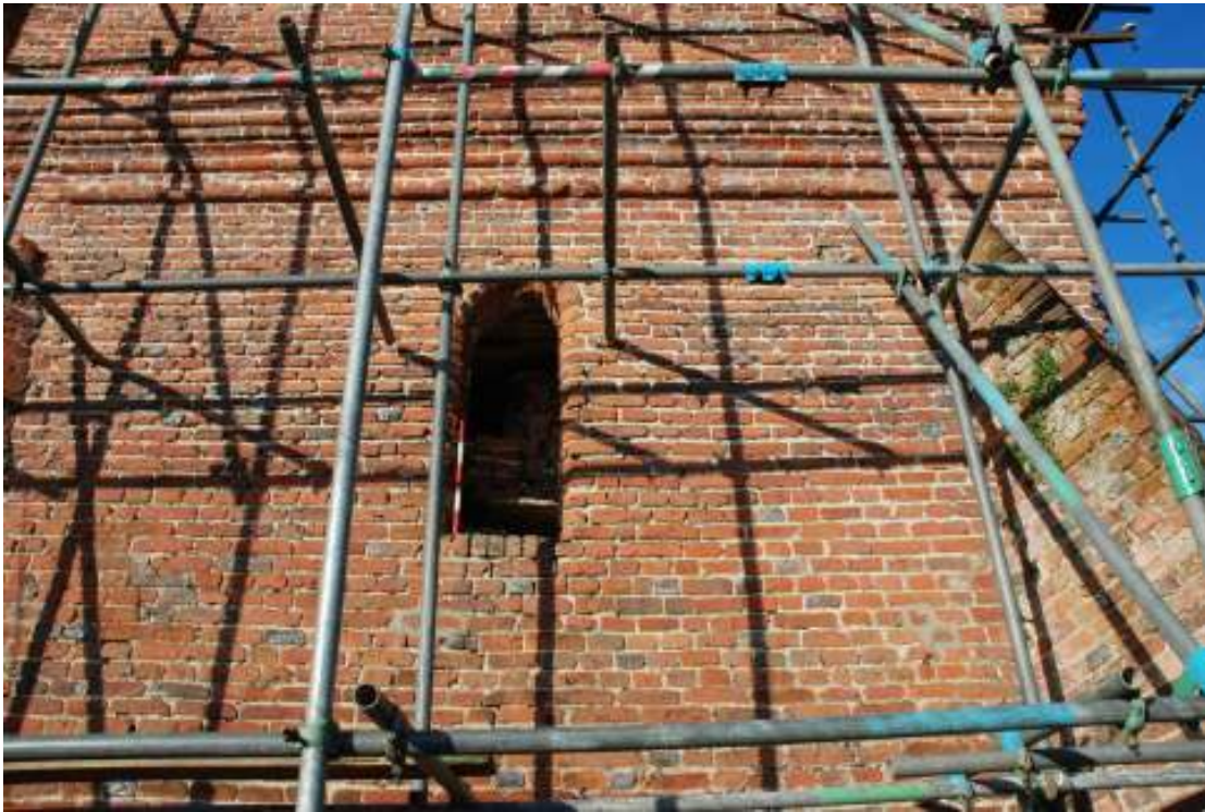
Fig. 31: Photograph of the window in the southern wall of the dovecote (from the outside). This clearly lies within the area of the original build (i.e. beneath the moulded courses of brickwork), and there is no indication that it was inserted at a later date.
