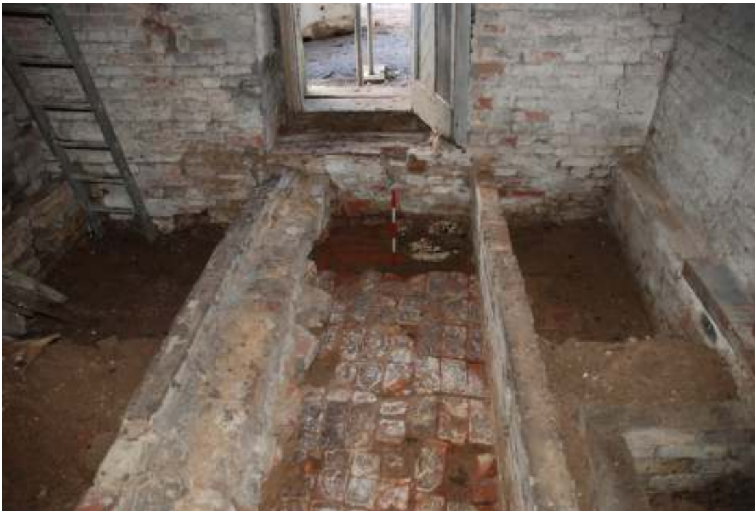
Fig. 84: Photograph of the brick floor, looking towards the western door.
