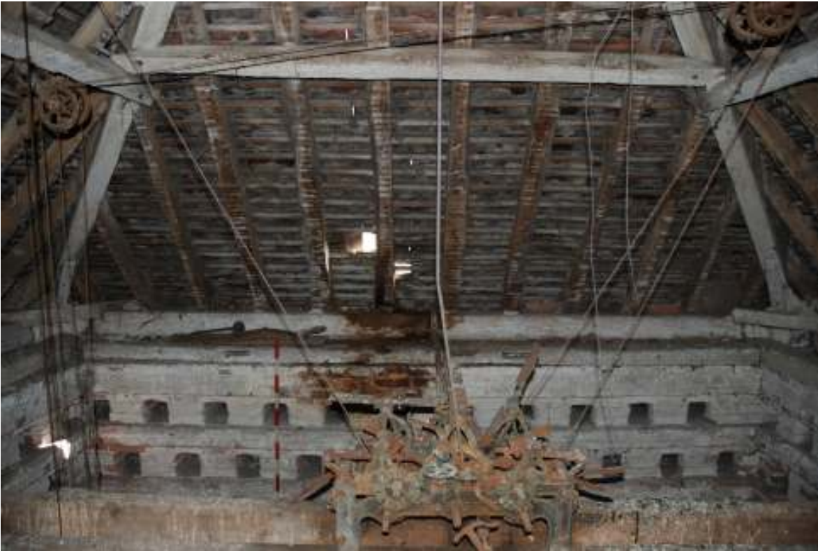
Fig. 117: Photograph of the interior roof of the dovecote. This clearly shows the wall-plates; hip-rafters; purlins; and rafters.
