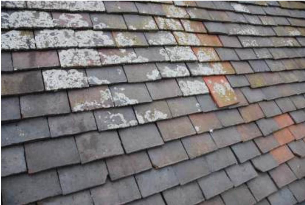
Fig. 115: Photograph of the overlapping tiles on the exterior of the roof.
