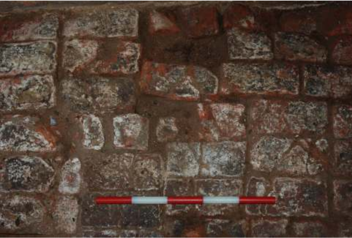
Fig. 85: Close-up photograph of the brick floor.
