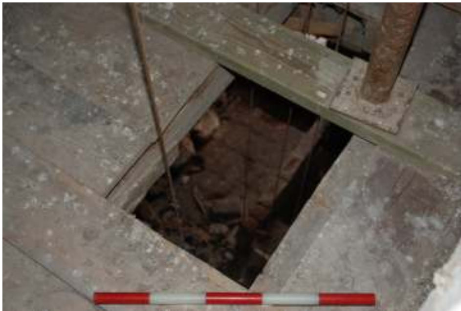
Fig. 159: Photograph of the modern floorboards on the first floor, overlying the earlier floorboards.
