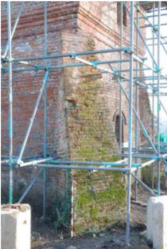
Fig. 101: Photograph of the north-western buttress.
