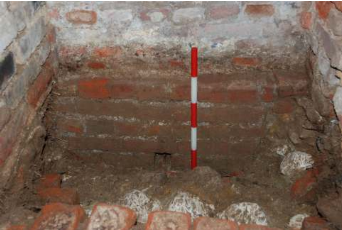
Fig. 89: Photograph of the interior of the eastern doorway. This shows the blocking-up of the lower part of the doorway, and the drain hole at the base of this.
