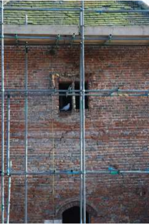
Fig. 75: Photograph of the window in the western wall (from the outside).
