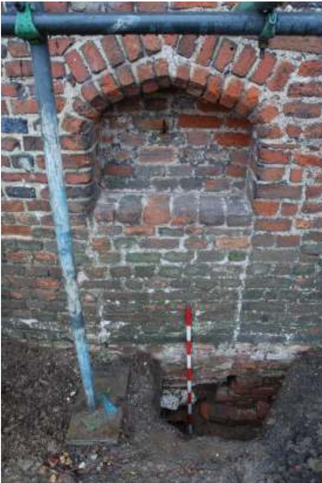
Fig. 120: Photograph of the exterior of the blocked-up eastern doorway. This clearly shows how it has been infilled.
