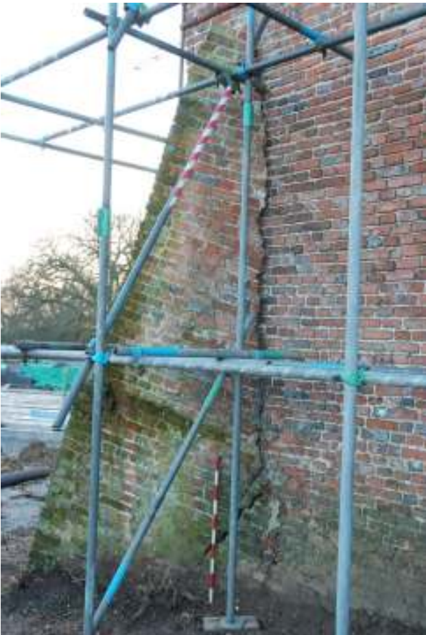
Fig. 96: Photograph of the eastern side of the south-eastern buttress. This clearly shows the rough abutting of the buttress to the main dovecote wall.
