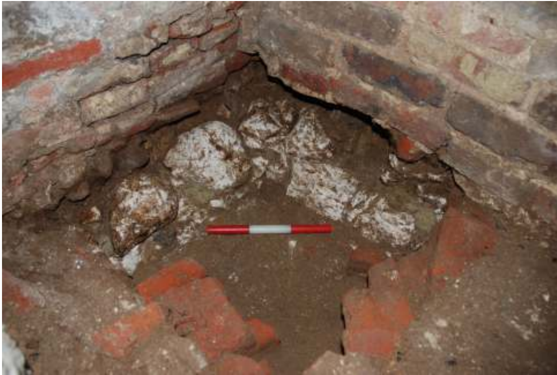
Fig. 42: Photograph of the chalk foundations observed in the north-west corner of the dovecote.
