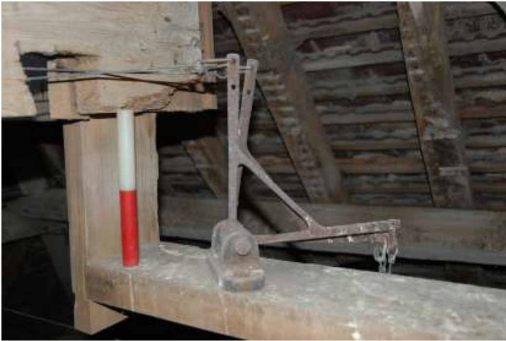
Fig. 140: Photograph of a pair of the bell-cranks.
