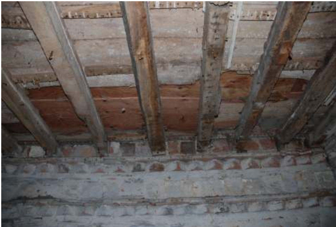
Fig. 104: Photograph of the underside of the first floor taken from the ground floor. This clearly shows how the joists are stuck into the nesting-holes.
