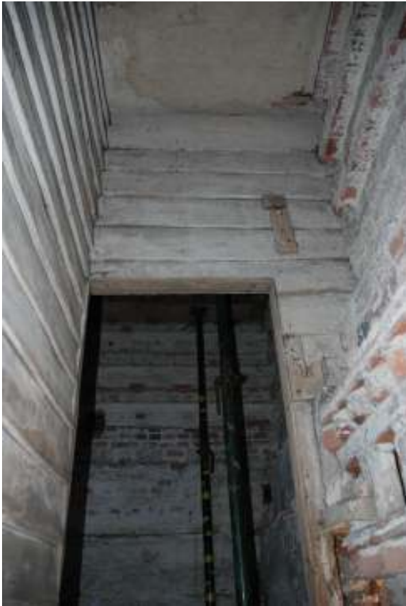
Fig. 106: Photograph showing the inside of the wooden 'chamber' surrounding the ladders on the first floor, with the lathe and plaster ceiling clearly visible.
