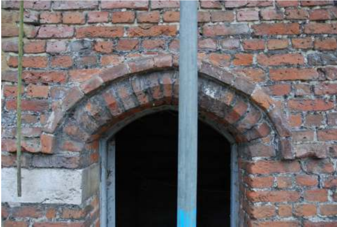
Fig. 123: Photograph of the exterior door-hood of the western doorway.
