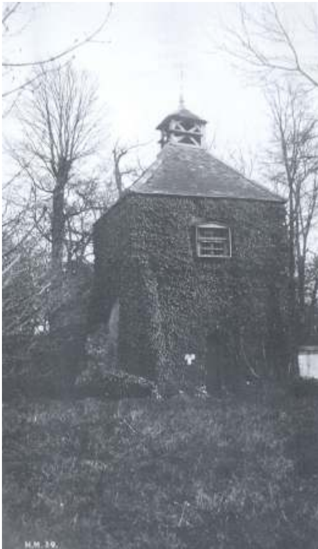
Fig. 7: 1923 photograph of the western side of the dovecote, clearly showing the existing western door and window; timber roof; cupola; and buttresses.
