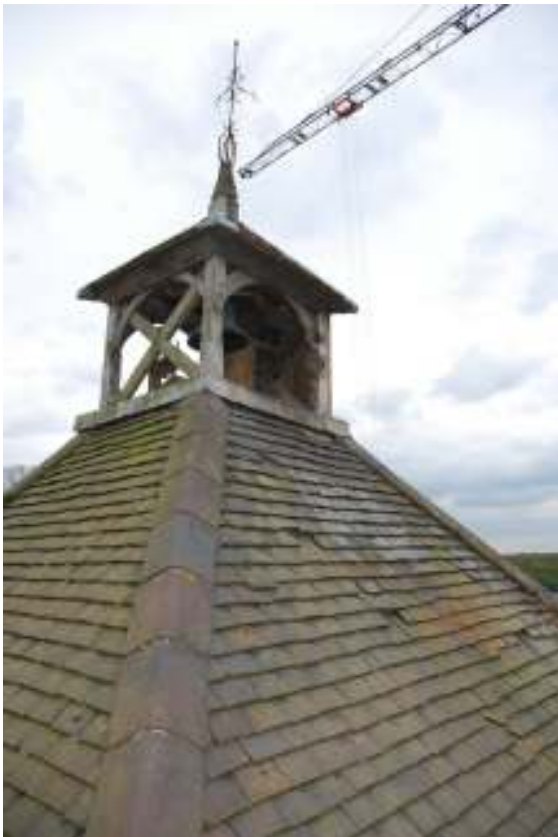
Fig. 114: Photograph of the roof and cupola, from the outside.
