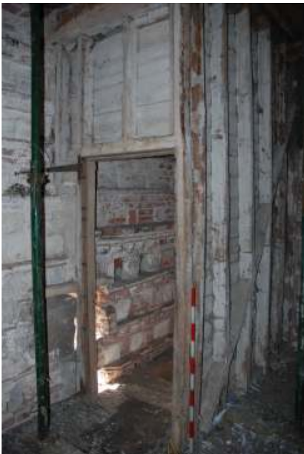
Fig. 107: Photograph showing the outside of the wooden 'chamber' surrounding the ladders on the first floor and the doorway into the first floor, clearly showing the hinges.
