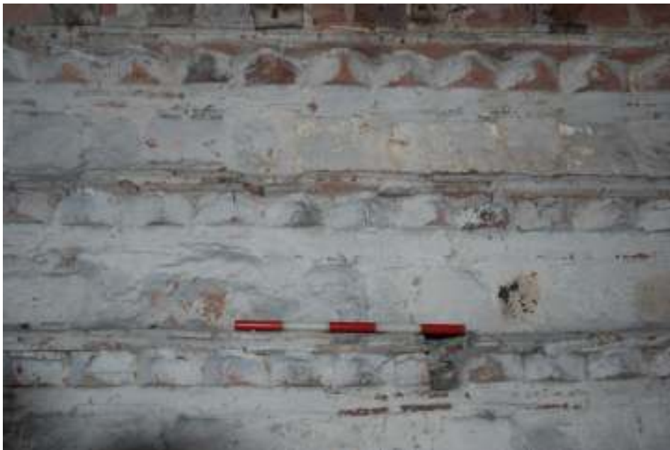
Fig. 103: Photograph showing a series of blocked-up nesting-holes on the ground floor. The nesting-holes have been blocked over by bricks or tiles placed horizontally.
