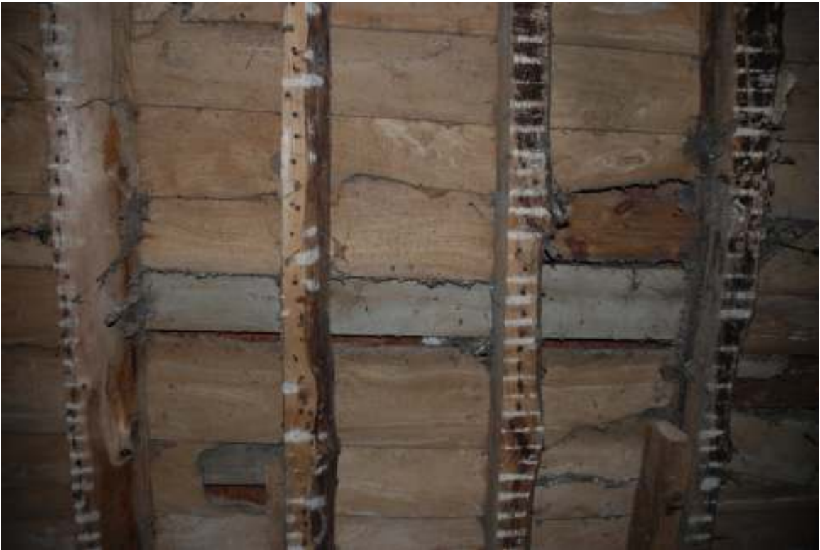
Fig. 111: Photograph showing beams with nails sticking out of them on the first floor (for the lath-and-plastering of the ceiling). The white lines visible horizontally across the beams are further evidence for the act of lath-and-plastering.
