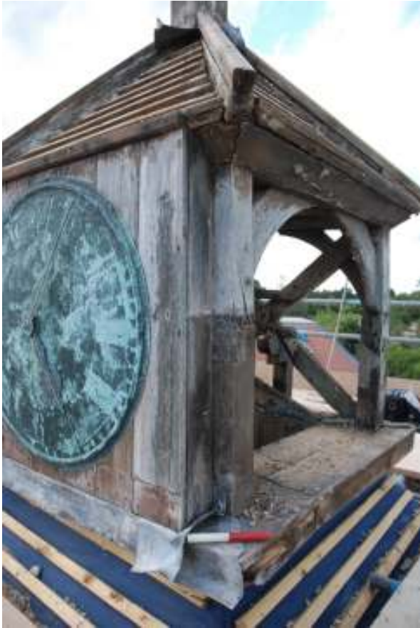
Fig. 116: Photograph of the wooden cupola at the top of the roof.
