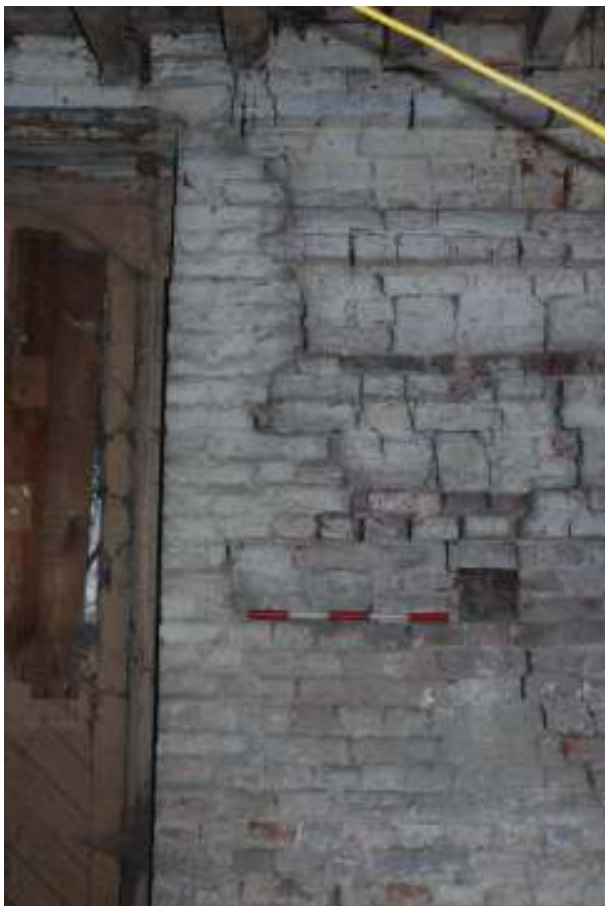
Fig. 126: Photograph of the northern side of the interior of the western doorway. This clearly shows how it was inserted at a later date.
