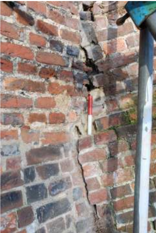
Fig. 100: Photograph of the western side of the south-western buttress. This clearly shows how the buttress roughly abuts the main dovecote wall.
