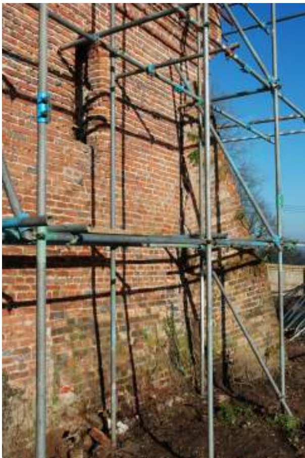
Fig. 130: Photograph of the patching on the southern wall of the dovecote.
