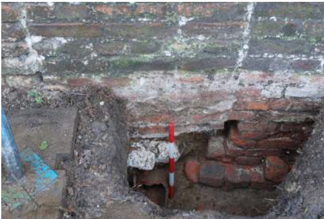
Fig. 36: Photograph of the small-scale excavation around the exterior of the eastern doorway. This shows the brick foundations and the two bricks with finished edges that may have formed the edge of some form of threshold into the dovecote.
