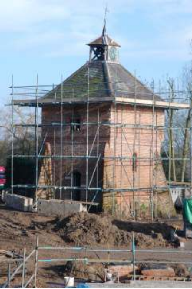
Fig. 113: Photograph showing the square roof and cupola, from the south-west.
