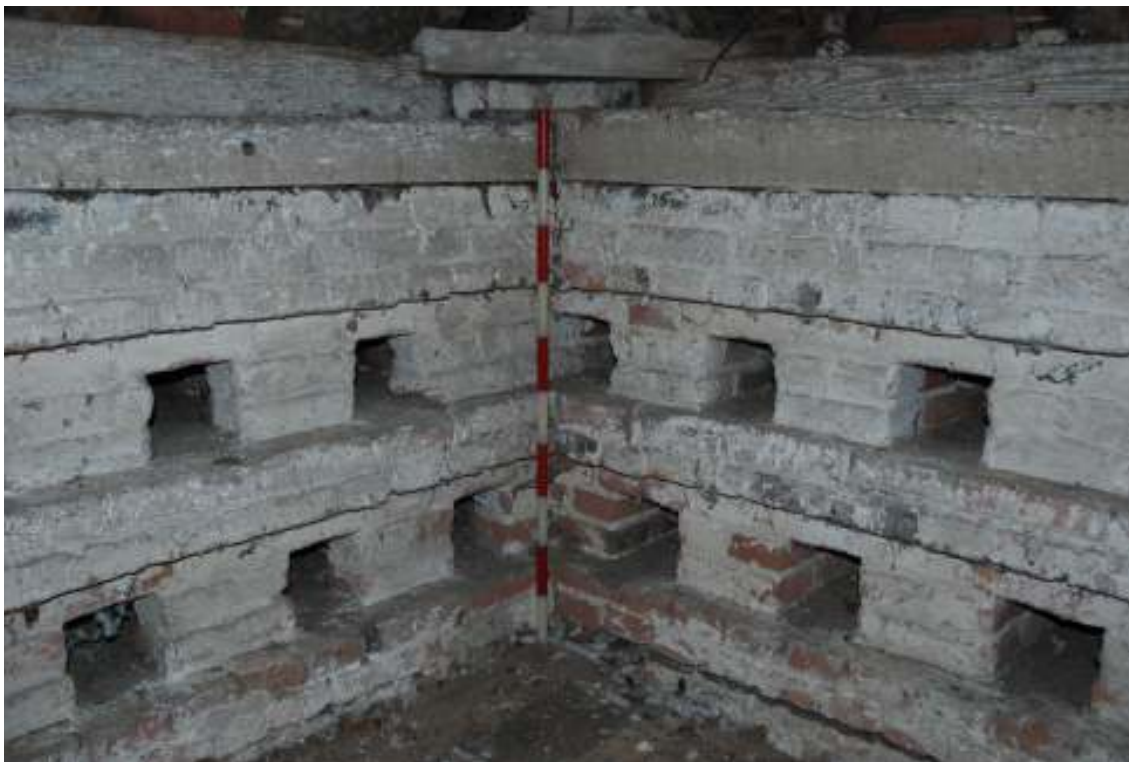
Fig. 63: Photograph of the nesting-holes in the south-eastern corner of the second floor. These are clearly the second type of nesting-holes (part of the rebuild) – with brick ledges.
