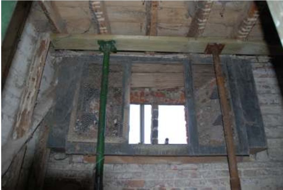
Fig. 157: Photograph of the western window, clearly showing the iron mesh between the nesting-holes and room.
