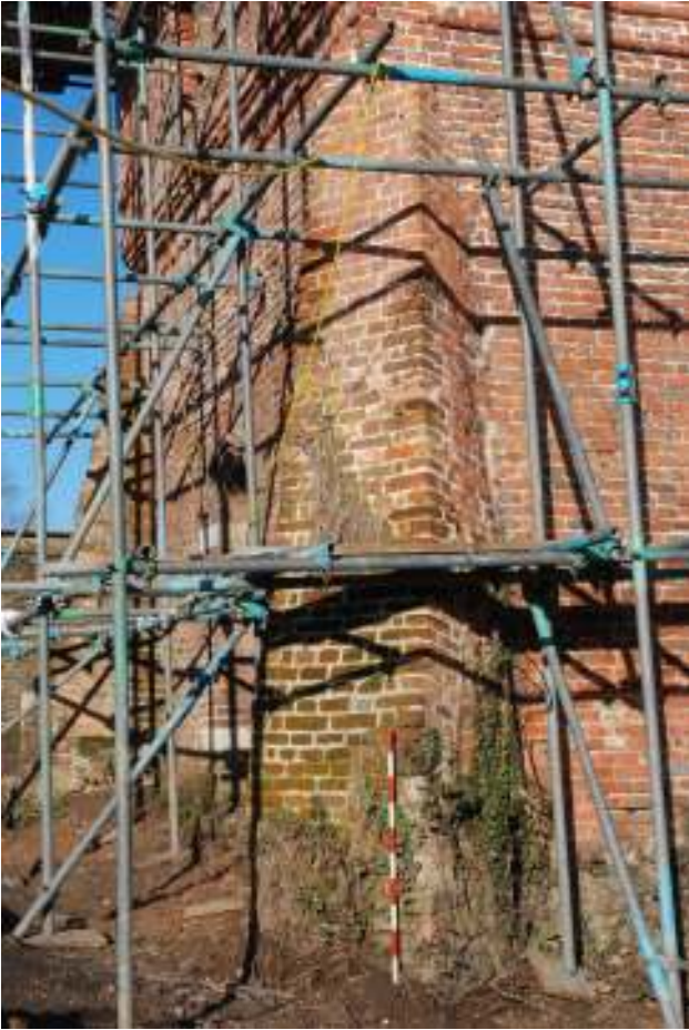
Fig. 99: Photograph of the front of the south-western buttress.
