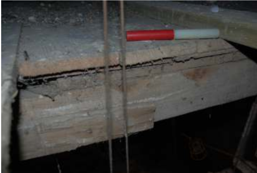
Fig. 145: Photograph showing the cutting-through of the original first- floor floorboards to make way for the clock weights. Saw cuts can be seen not only across the boards, but also on the side of the underlying joist.
