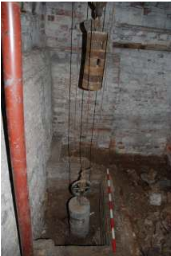
Fig. 147: Photograph of the going and striking train weights (going train weight above striking train weight).
