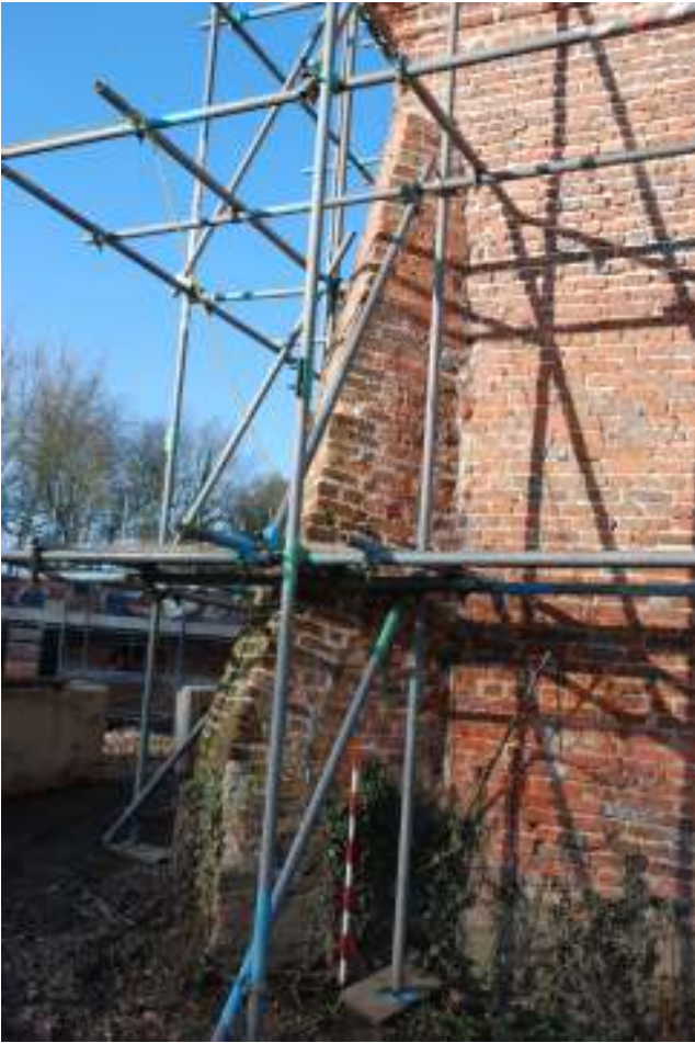
Fig. 97: Photograph of the eastern side of the south-western buttress. This clearly shows the later patching of the edge of the buttress.
