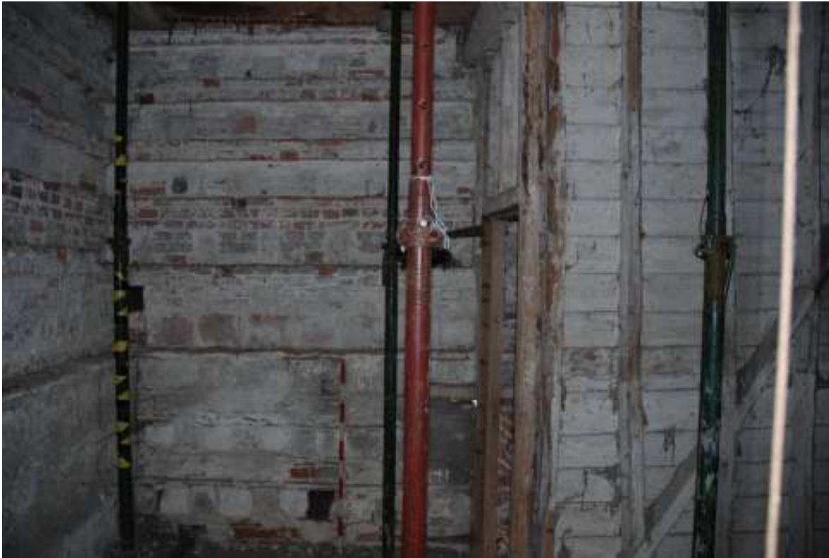
Fig. 53: Photograph of the interior southern wall – first floor.
