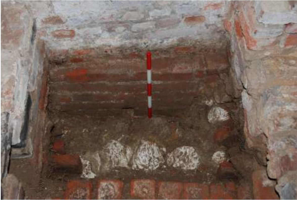
Fig. 43: Photograph of the chalk foundations that appear to head underneath the brick floor, just under the eastern doorway. This may represent the chalk base of an earlier floor.
