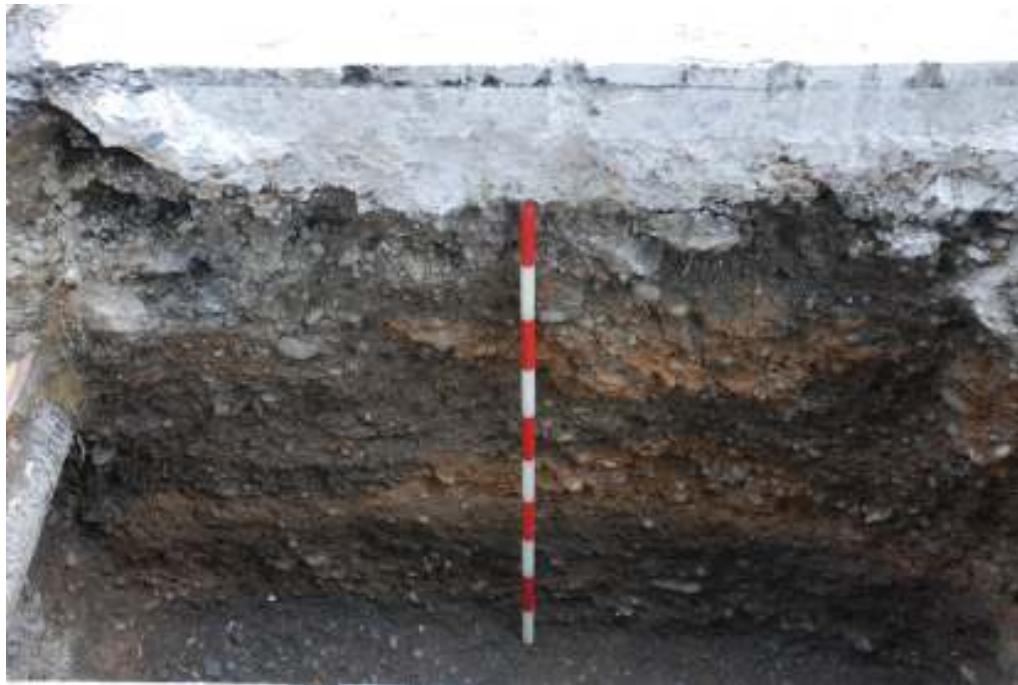
Fig.12: West facing section of pit at southern end of Trench 2 showing previous road make-up levels
