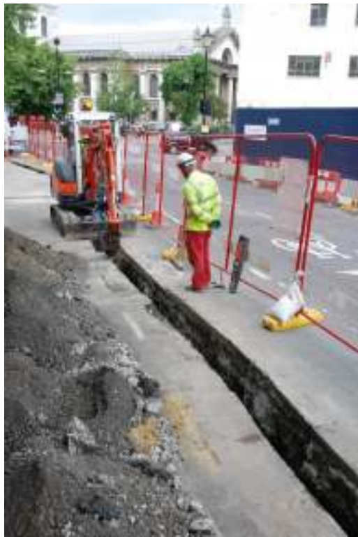
Fig.11: Stockwell Street trenching, looking approximately North
