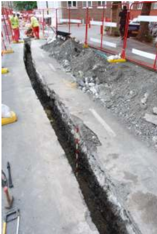
Fig.9: Stockwell Street open cut trench, looking SE
