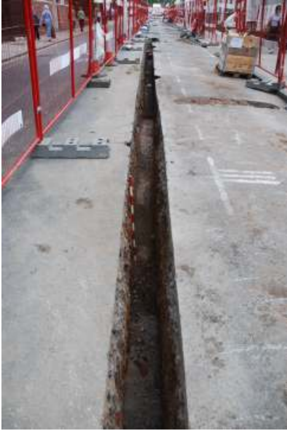
Fig.19: Trench 6 facing south, with underground rail tunnel in foreground
