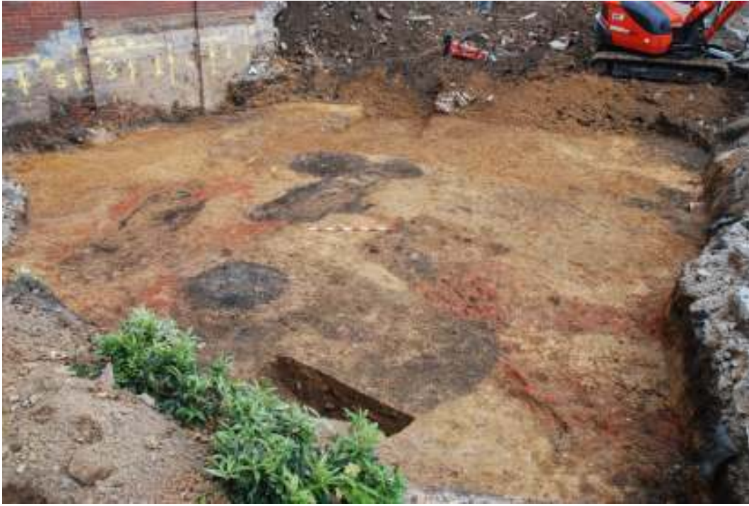
Fig. 58: Photograph of rubbish pit [64], looking north-west – dark brown area in the foreground, with half of it excavated.
