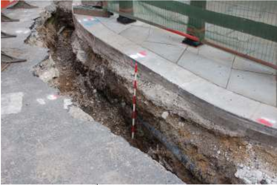
Fig.39: Basinghall Street 7 th June 2011. Section through trench Facing NE
