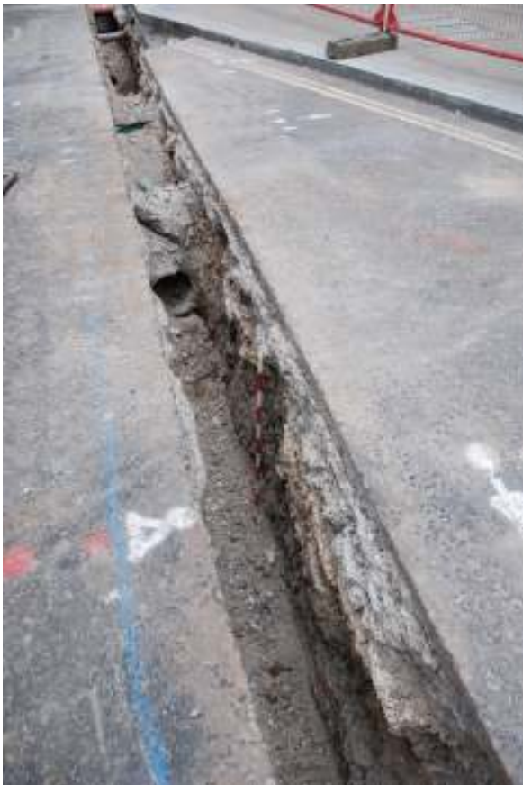
Fig.47: Wood Street 27 th July 2011, Facing S
