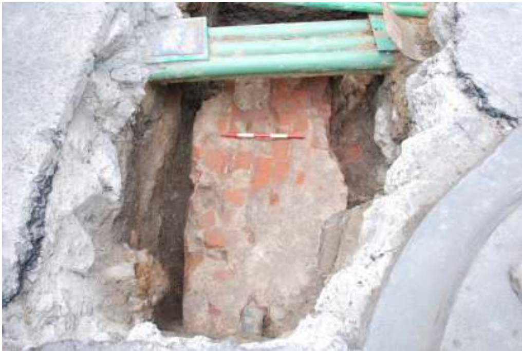
Fig.16: Brickwork of former Moorgate exposed in Trench, facing S, (0.6m scale)
