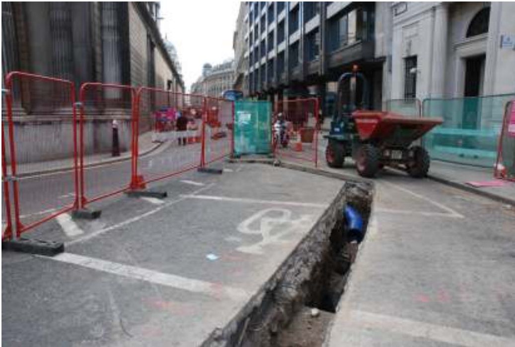
Fig.43: Lothbury 9 th August 2011, facing SE
