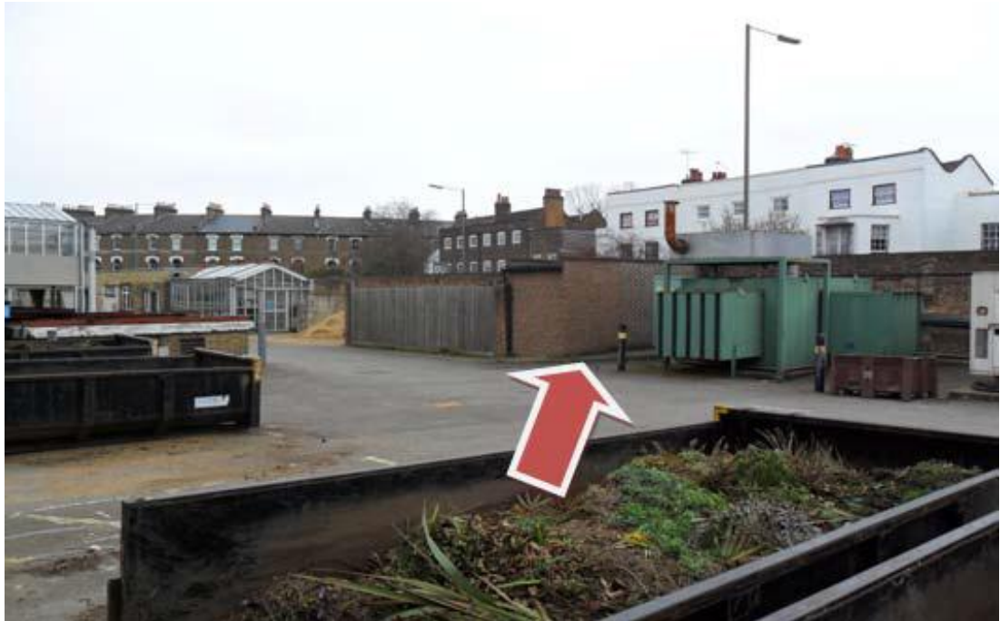
Fig 15 Location of the VO unit at the Jodrell Switch Chamber.
