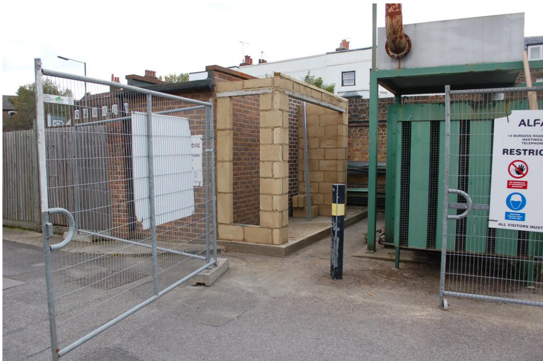
Fig 16 The VO Unit under construction.
