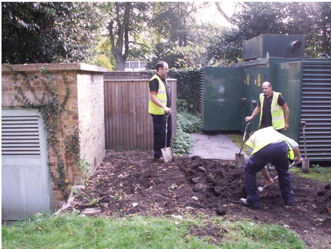
Fig 19 Ground reduction of surface topsoil for construction of the VO Unit.
