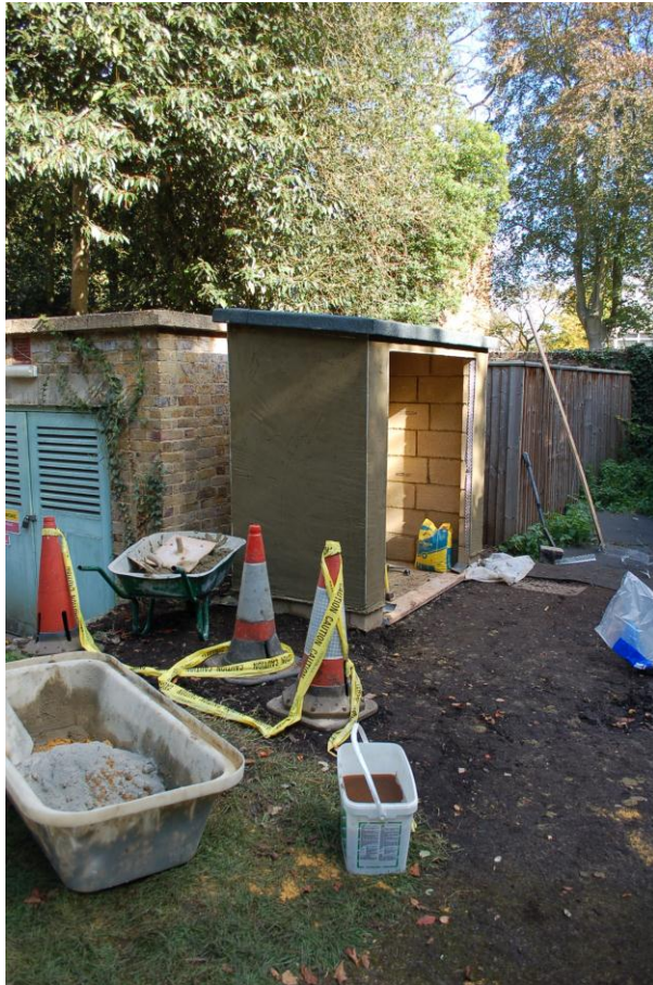
Fig 24 The MNG VO Unit under construction.
