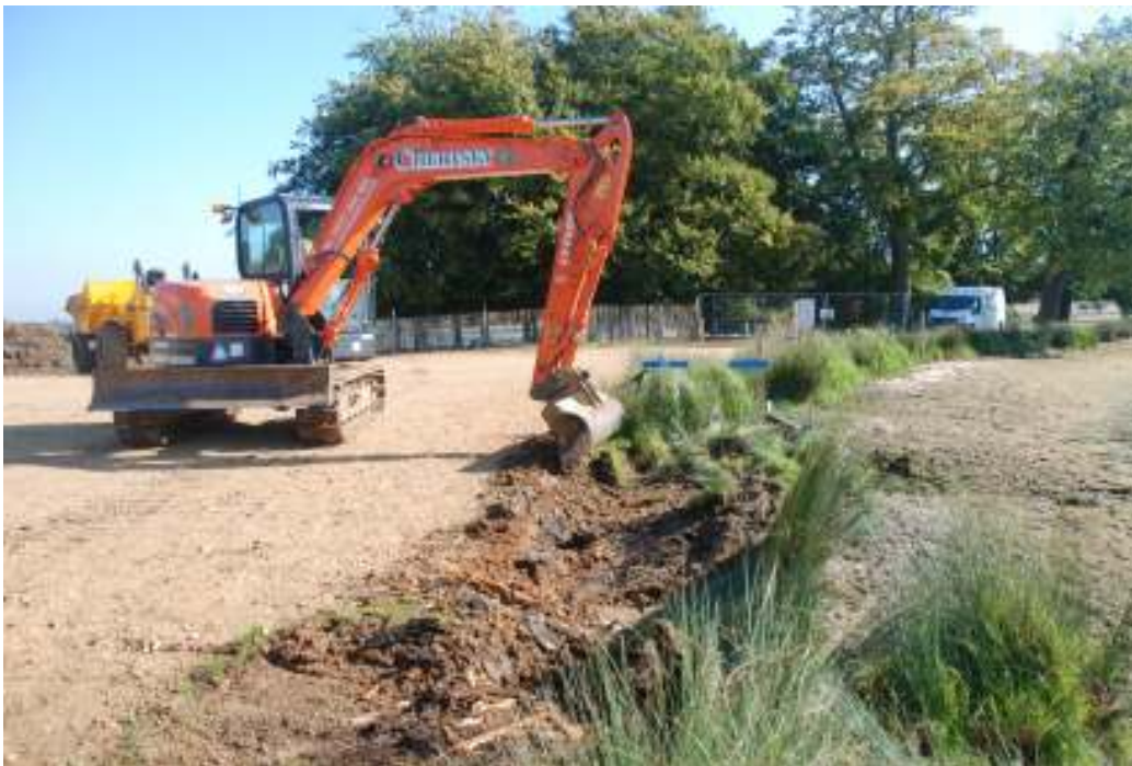
Fig.22: Working shot by Upper Pen pond, facing E along pond edge
